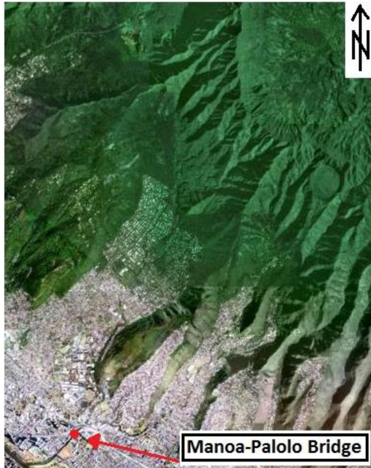
Figure 3-4 The Manoa-Palolo Watershed and surrounding area
