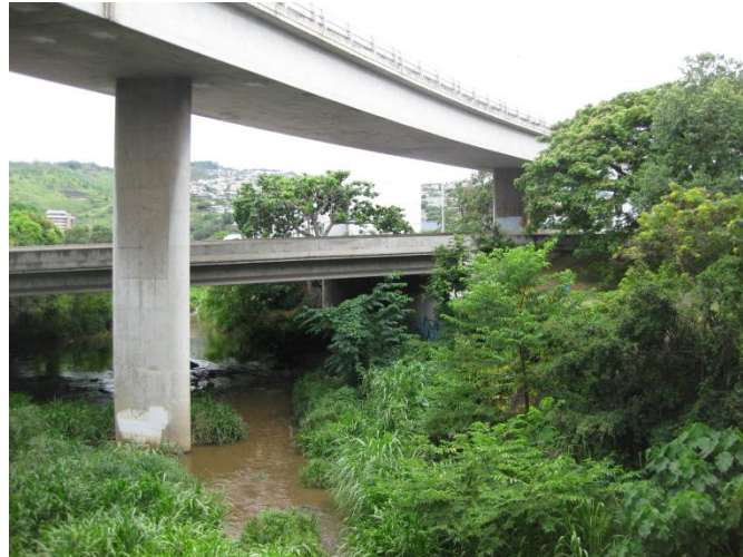
Figure 4-2 Manoa-Palolo Bridge, Honolulu, HI
