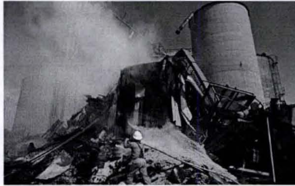
Figure 5.7 Silo explosions are an example of the highly combustible properties exhibited by many dusts.
