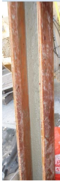
Figure 3-11 Prime the flow trough
