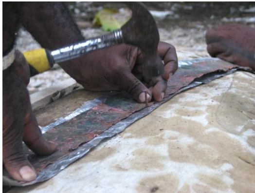
Copper strips seal the gap between the iwa and the yepe waa . Reflective roofing insulate underneath seems to work well in indigenous theory.
