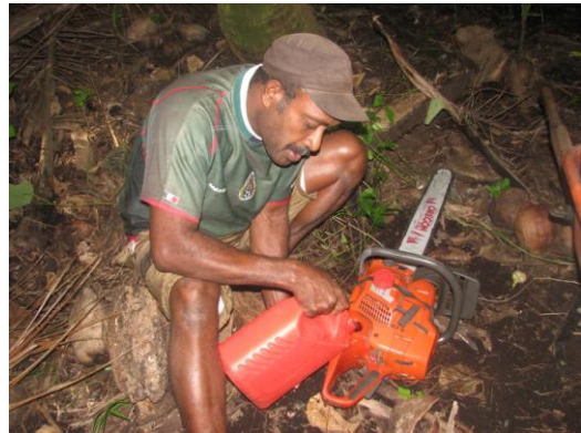
Thirty minutes with Ben Kalo's chainsaw saved the builders three days of work with axes and adzes.
