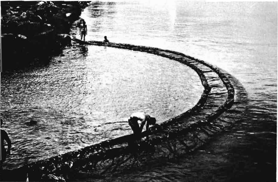
Figure 5. Double membrane curtain in place (stream inflow is from left)
