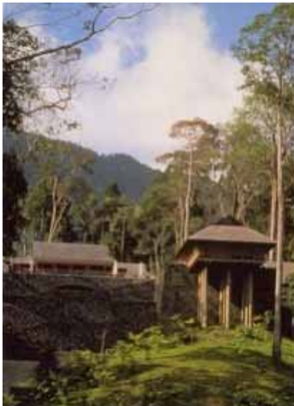
Right: Figure 5. Some of the felled tree trunks were left in their original form giving the impression that the colonnaded area was an extension of the forest (Source: Architect's submission to AKAA)
