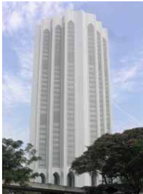
Figure 9. Exterior view of Dayabumi Complex. (Source: Author’s photograph)
