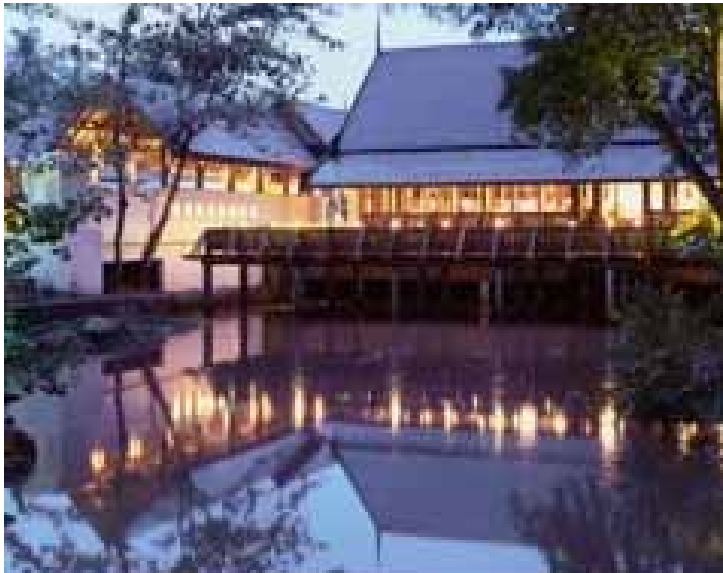
Figure 14. View of the New Tanjong Jara Hotel (Source: Tanjong Jara Hotel official website)
