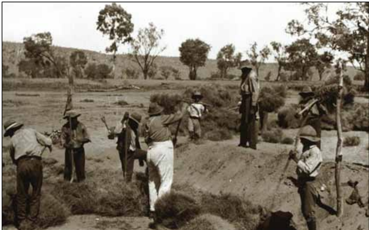
Figure 13. Workers laying spinifex during road construction in Central Australia 1912-1951. Photograph is part of the Australian Inland Mission Collection (nla.pic-an24666817). [Image courtesy of National Library of Australia].
