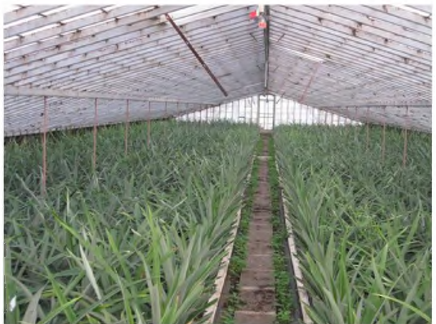
Figure 1. A typical pineapple production house on S. Miguel Island, Azores. The structure is very similar to the original counterparts from the late 19th century.
