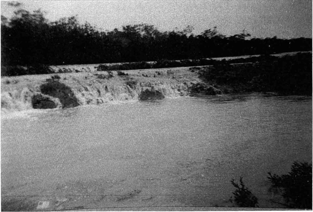
FIGURE 12. High seas caused by storm surge associated with Cyclone Gavin spilling over the sea wall at Tabucola on the northern coast of Vanua Levu near Labasa, 1400 hours on 7 March. Photo courtesy of Drainage and Irrigation, Public Works Department.
