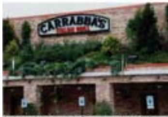
An intensive green roof on a restaurant in Lansing Michigan.
