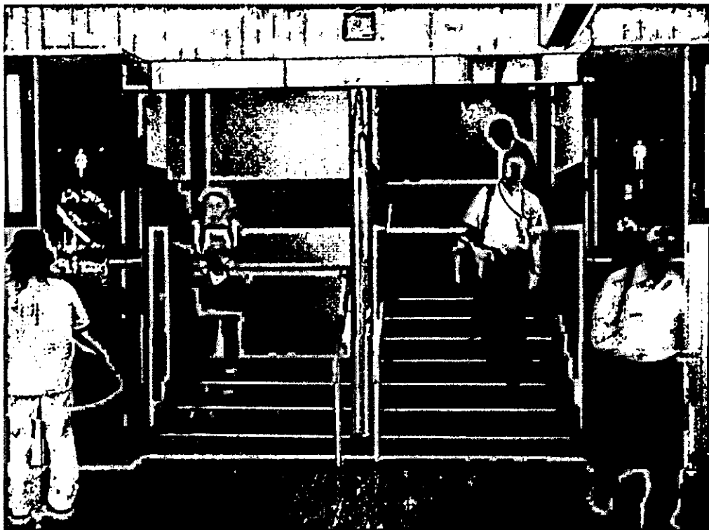
Photo 32 This inaccessible bathroom is at the top of the steps from photo 31.
