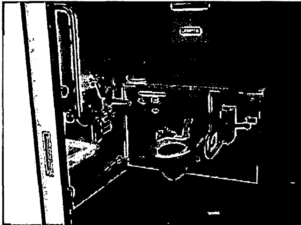
Photo 36 Interior of the accessible bathroom.
