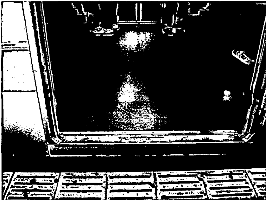
Photo 29 Announcements tell you to be aware of the gap between the train and the platform. But the step up to the train can be just as much of a problem.
