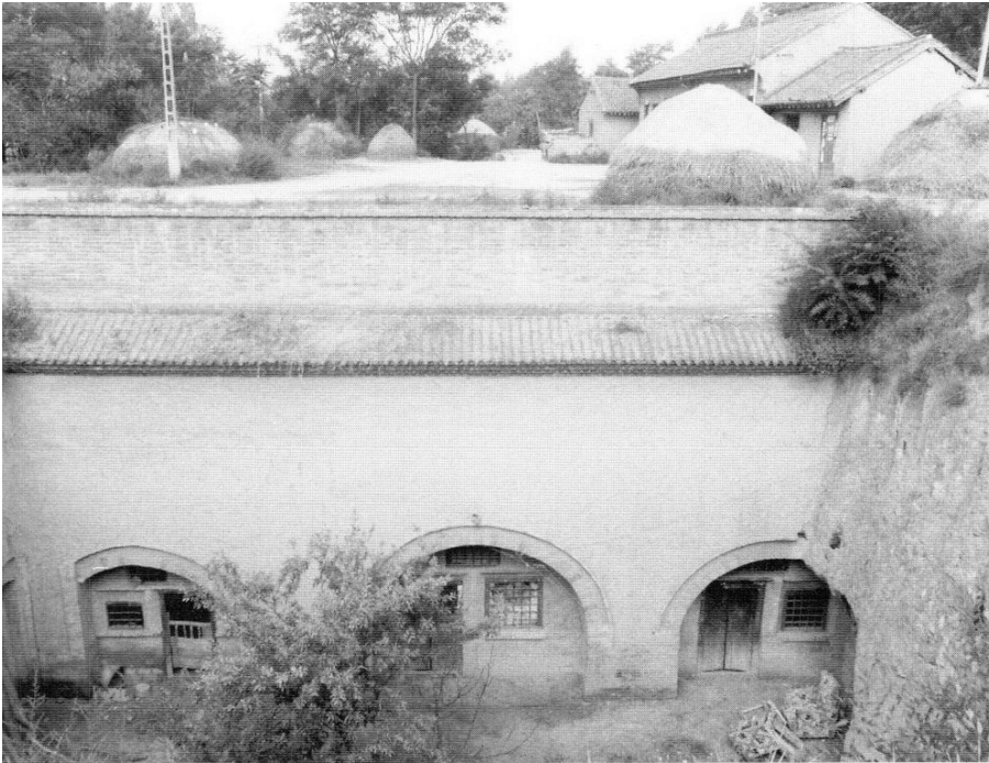
Figure 4.74 (top left). To protect the flat wall surfaces from deteriorating from rain-wash or gravity displacement, they are sometimes capped with brick and tile and finished with a lime plaster. Houwang cun , Pinglu xian , Shanxi. [RGK photograph 1996.]
