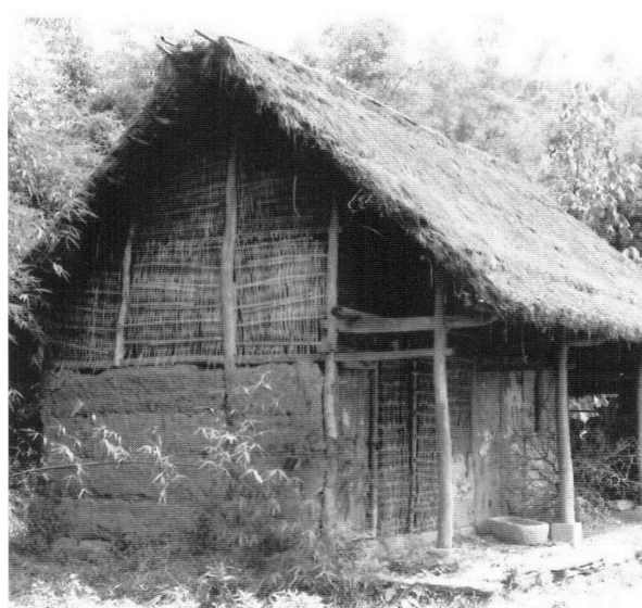
Figure 5.10. Although structurally more complex with its mortise and tenon pillars and beams, this modest three-bay dwelling includes a low wall of tamped earth, above which is woven split bamboo walling. Eaves brackets are extended to the slender peripheral pillars in order to make a portico. The doors are made of woven bamboo. Zhuangyuan cun , near Langzhong, Sichuan. [RGK photograph 1995.]
