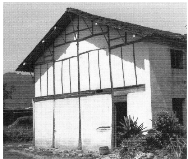
Figure 3.27. It is clear that the five thin pillars rising along the lower wall of this two-story dwelling cannot support the heavy weight above and that the weight is being carried by a load-bearing wall, probably of adobe or fired brick upon which a strong girder has been raised. The upper story is clearly a chuandou framework, with five major pillars and eight minor ones and tie beams in the understory below the eaves. Cangpo cun , Gangtou xiang , Yongjia xian , Zhejiang. [RGK photograph 1990.]
