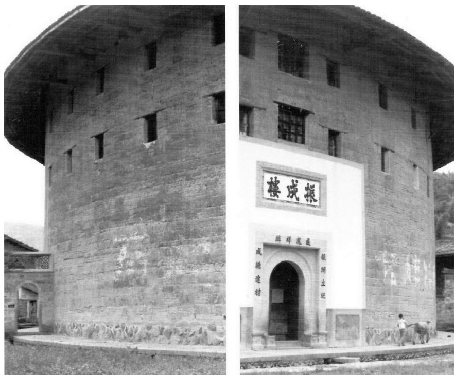
Figure 5.75. Except for a single entry portal that is framed by a white border with the name of the complex inscribed above it, the lower two stories of Zhenchenglou have no fenestration. Openings are only placed along the third and fourth levels. Hongkeng cun , Hukeng xiang , Yongding xian , Fujian. [RGK photographs 1990.]
