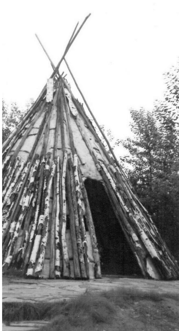
Figure 6.32. Oroqen and Ewenki traditionally built simple conical structures made of larch poles that were covered with birch bark in summer and reindeer hides in winter. As herding and hunting has lessened, more have moved into log dwellings. This is a replica of an Oroqen tepee-like structure in the Chinese Ethnic Culture Park, Beijing. [RGK photograph 1996.]
