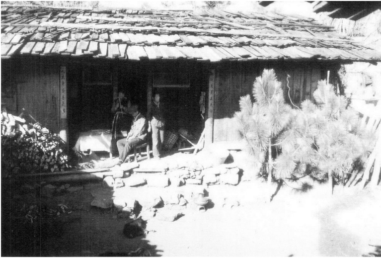
Figure 5.117. In the remote areas of northern Yunnan, Naxi still build single-story house compounds arranged in a village cluster for ten to thirty families. The main structure in each compound includes space for receiving guests, sleeping, cooking, and storage. A raised triangular hearth provides interior space for eating, entertaining, and sleeping. Directly opposite from and parallel to the residential unit is an area that serves as a stable. In this photograph, Han-style red paper couplets have been hung alongside the entry in anticipation of the New Year, while two pine trees are the focus of a Naxi sacrifice to ancestors ritual. Lijiang xian , Mingyin xiang , Yunnan. [Original photograph used with the permission of Charles McKhann.]
