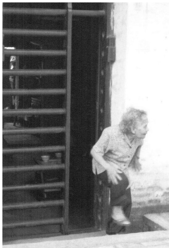
Figure 5.30. In order to enhance ventilation and to provide security in the dwellings of rural Hong Kong and in the towns and villages of nearby coastal Guangdong, ingenious "gates" called tanglong are formed from horizontal wooden bars that slide as a unit into granite sockets hewn into the door frame. Coastal Guangdong. [RGK photograph 1993.]
