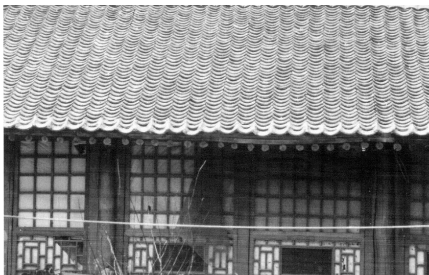
Figure 3.160. Once set in mud and lime on a northern roof, arcuate tiles provide a corrugated surface for water to flow to the eaves. Beijing. [RGK photograph 1987.]
