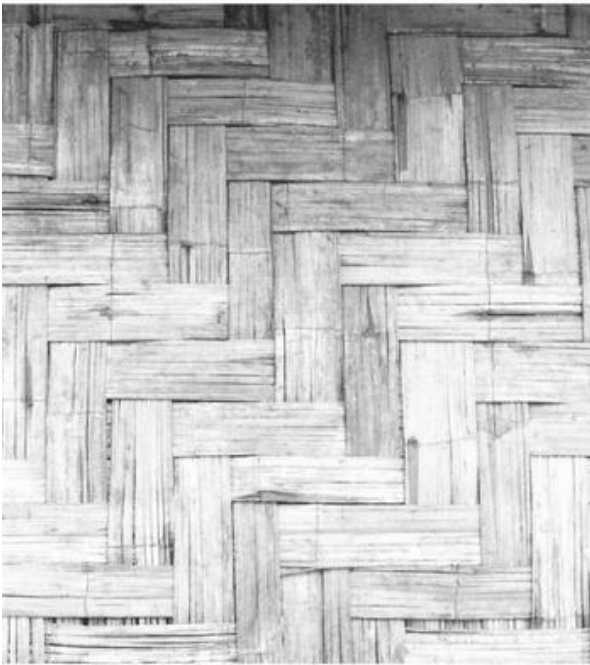
Figure 3.51. Finely split bamboo is woven into broad bands to form artful patterns in this walling of a re-constructed Hani ganlan structure. Chinese Ethnic Culture Park, Beijing. [RGK photograph 1993.]
