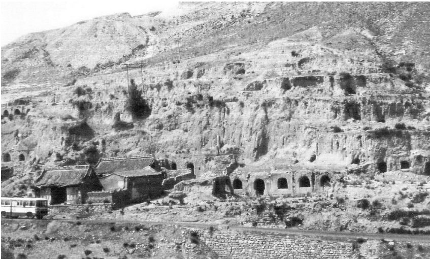
Figure 4.51. Slumping has brought about the collapse of several levels of kaoshan yaodong along this irregular slope. Several unused yaodong are visible as is an abandoned siheyuan complex, perhaps an old temple, that has yaodong associated with it. [Original photograph used with the permission of Kentaro Yamato.]
