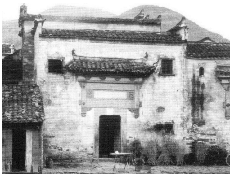
Figure 5.39. Built along the road connecting Tunxi in Anhui and Hangzhou in Zhejiang, this two-story old dwelling is similar in width to the one in Figure 5.38. However, the much more elaborate entryway and the receding rooflines tell us it is a grander dwelling of an earlier period. Ningyuantang, Zhanqi cun , Shexian, Anhui. [RGK photograph 1987.]
