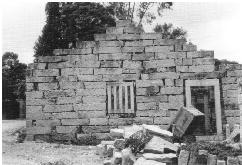
Figure 3.106. Quarried granite slabs for walls as well as window and door frames are stacked loosely, then mortared. Linfang cun , Zhendong xiang , Fujian. [RGK photograph 1990.]
