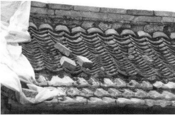
Figure 3.156 (top left). Before tiles are laid on a roof in northern China, a layer of wood, twig, or reed matting is put in place, followed by a bedding layer of mud and a bonding layer of lime. Taiyuan, Shanxi. [Original photograph used with the permission of Arthur J. Van Alstyne.]
