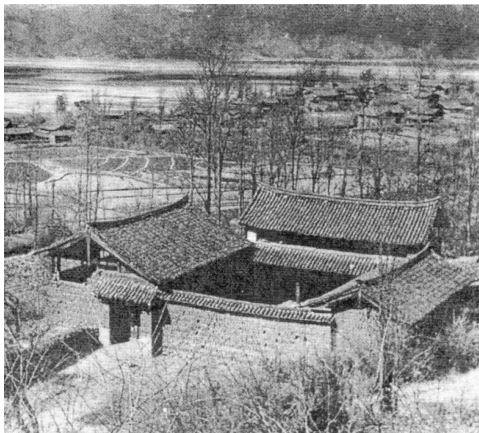
Figure 5.118. Built around a walled courtyard entered through a gate, this Naxi single-story house has walls of tamped earth and a roof of wooden shingles. The overhanging gables allow air to circulate into the complex. Haibei cun , Naxi Lijiang Autonomous xian , Yunnan. [Source: Liu 1990, 275.]
