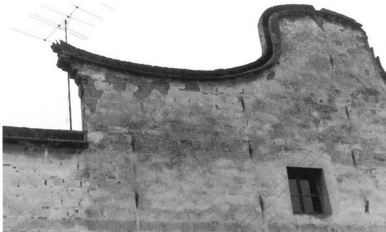
Figure 3.133. Constructed of kongdou brickwork, this elevated wall has a convex middle section and feather-like ends. Zhili zhen, Huzhou shi, Zhejiang. [RGK photograph 1988.]
