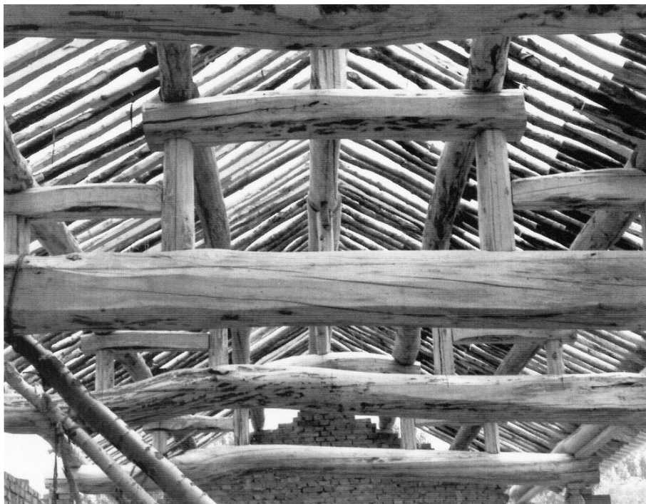
Figure 3.19. Because of the width and depth of this dwelling, several adjustments have been made to the tailiang framework: purlins rest directly on the brick gable walls and short beams have been tenoned into queen posts in order to support an additional set of purlins. Beijing area. [RGK photograph 1987.]
