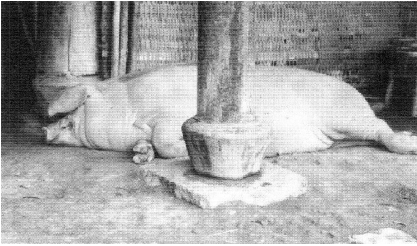
Figure 3.13 (above). Supporting a wooden pillar holding up a roof overhang, this simple stone base rests on a thin piece of square stone set into the earthen floor of this modest dwelling. A matching base along the wall is just beyond the pig's head. Shuitou xiang , Cangnan xian , Zhejiang. [RGK photograph 1988.]
