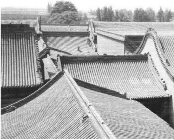
Figure 3.137. Even on roofs of manor complexes, the roofline can be relatively sedate. The single roof ridge running forward is capped by a brick molding to seal the juncture between the two tiled roof slopes. Caojia Manor, Beiguang, Taigu, Shanxi. [RGK photograph 1996.]
