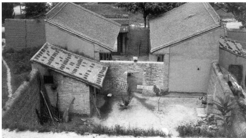
Figure 4.23. This incipient Shaanxi-style dwelling is being built in stages. Viewed from the rear, it is clear that the side xiangfang were constructed first. The walled space remaining in the foreground serves now as a courtyard but will eventually be occupied by a horizontal main zhengfang structure that will link the xiangfang . Each xiangfang has a single-sloped roof draining inward to the narrow courtyard. A simple gate is located along the southeast section of the wall. Central Shaanxi. [RGK photograph 1991.]
