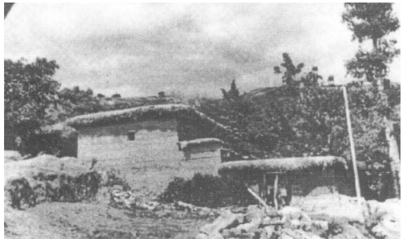
Figure 6.13. Like Tibetans, the Qiang build multistory blockhouses of stone and sometimes adobe on the steep hill slopes of western Sichuan. Dwellings are usually stepped into the hillside, with animals stabled on the ground level and living space above. In some Qiang villages, tall stone towers are used as a refuge during times of strife. Maowen Qiang Autonomous Prefecture, Sichuan. [Source: Cao 1992, 73-74.]
