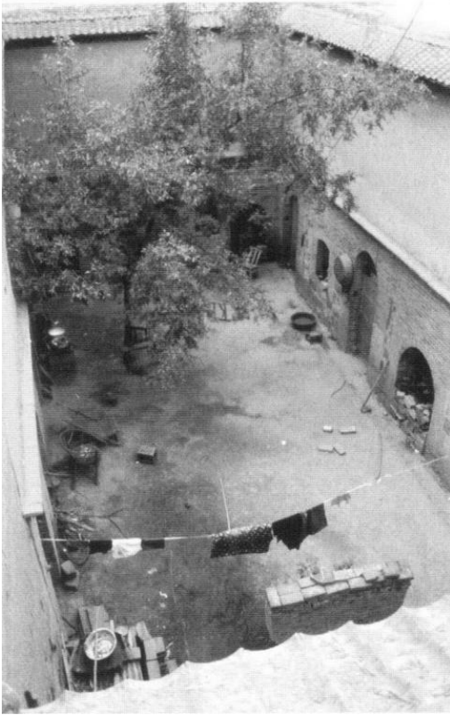
Figure 4.67 (top right). This perspective view shows the recessed courtyard with its four sidewalls into which one, two, or three yaodong are dug. Sloped entries lead to the ground above. While a tree is often planted within a courtyard, vegetation is kept far away from the pit on the surface because of the potential damage from roots. Henan. [Original line drawing used with the permission of the family of the late Paul Sun.]
