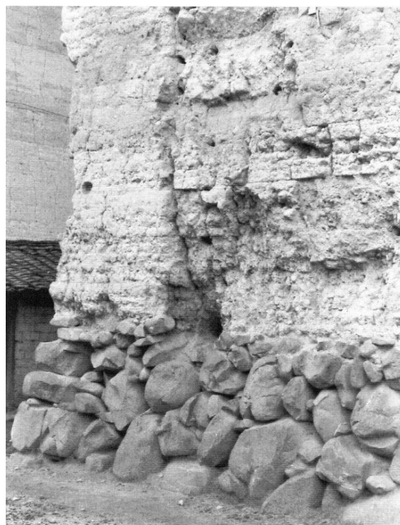
Figure 3.7 (top right). Boulders are carefully placed at the base of this Hakka fortresslike dwelling. Yanglinglou, Nanjing xian , Fujian. [RGK photograph 1990.]
