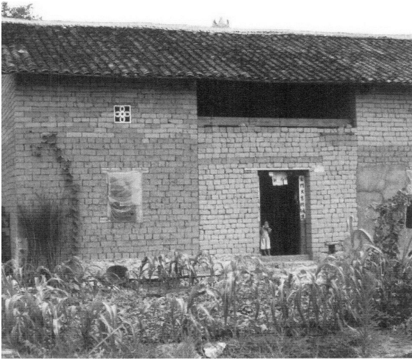
Figure 3.81. Recently constructed of adobe brick with a wooden tailiang frame, this massive two-story dwelling lacks windows on the back and sides. A wall across the middle of the facade stops short of the eaves to let in some light and air and complements the two low windows and upper ventilation ports. Fenghuo xian , Liqun xian , Shaanxi. [RGK photograph 1991.]
