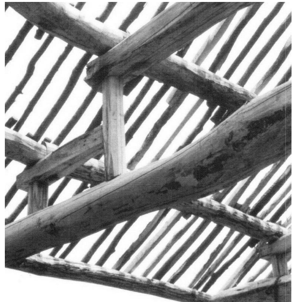
Figure 3.22 (above). Inclined rafters that are slight in diameter are laid across the purlins—from the ridgepole down to the top of the wall—to support the roof covering. Huairou xian , Beijing. [RGK photograph 1987.]
