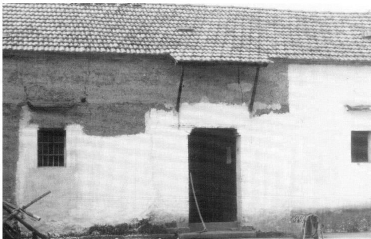
Figure 3.70. Although many tamped earth walls are left a tawny color without any coating, some are spread with a lime or a soil slurry plaster once the wall cures. White walls reflect, rather than absorb solar energy and thus contribute somewhat to limiting a heat buildup. Changle cun , Zhuge xiang , Lanxi shi , Zhejiang. [RGK photograph 1987.]
