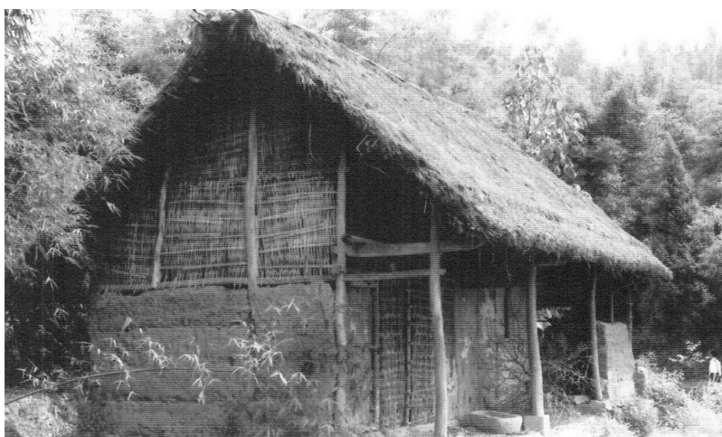
Figure 3.47. The lower walls of this humble thatched dwelling are made of tamped earth, while the upper areas are of plaited bamboo splines. Zhuangyuan area, Langzhong shi , Sichuan. [RGK photograph 1994.]
