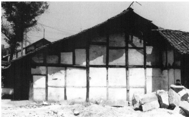
Figure 3.135. "Overhanging gables" [ xuanshanding or tiaoshanding ] are formed when the roof purlins extend beyond the endwalls. The purlins supporting the roof on this dwelling are each held up by wooden pillars in a chuandou frame. The panels between the wooden members are made of woven bamboo covered with a white plaster. The depth of the eaves overhang on the end and at the back is suggested by the extent of shade cast on the structure. Langzhong area, Sichuan. [RGK photograph 1994.]
