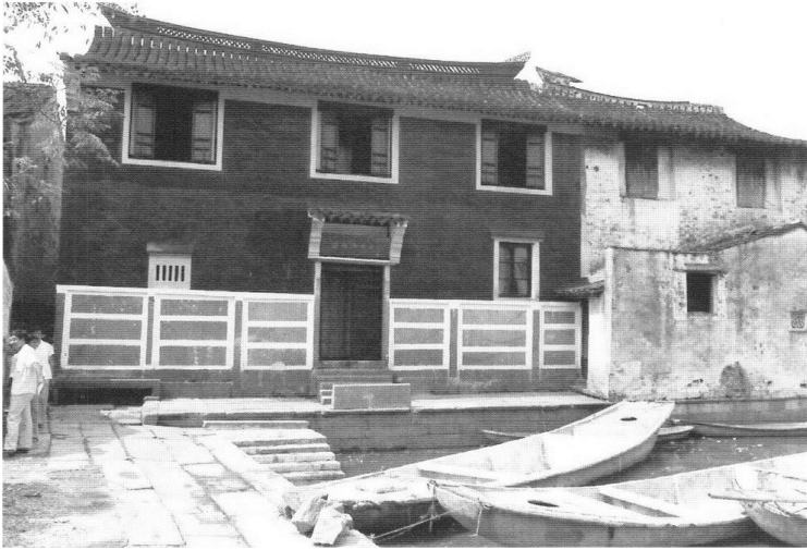
Figure 3.114. This symmetrical canalside townhouse, the home of the early twentieth-century woman revolutionary Xu Xiling, has a unique lower wall made of stone slabs with an upper wall made of kongdou cavity brickwork. Dongpu zhen, Shaoxing shi, Zhejiang. [RGK photograph 1987.]
