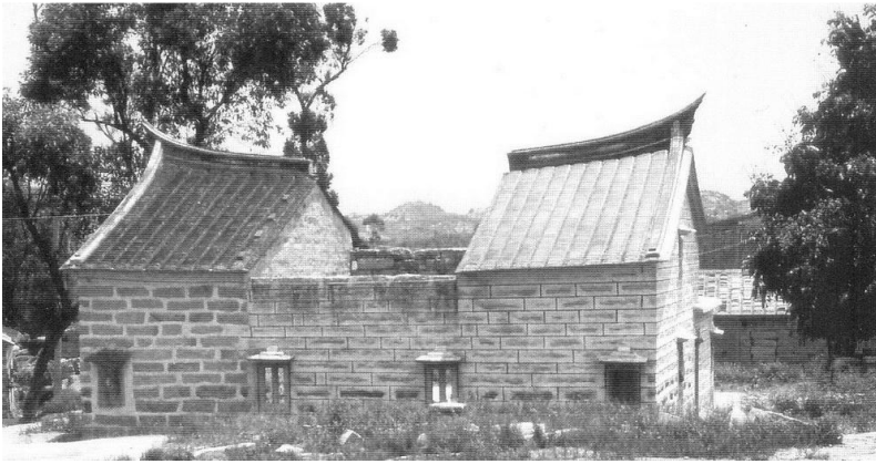
Figure 3.107. Once each of the granite slabs is in place and mortar is applied to seal and finish the joints, dark lines are drawn in order to regularize the pattern. Linfang cun , Zhendong xiang , Fujian. [RGK photograph 1990.]
