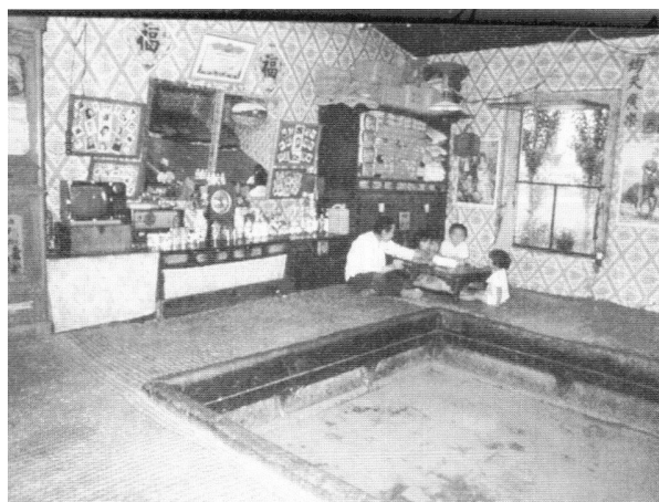
Figure 4.13. U-shaped kang are usually elevated above a floor surface and provide a ring of heat-radiating surfaces for daily life. In this new dwelling, the walls are papered and a large glass window allows winter sun into the dwelling. Northeast China [Source: Lu 1992, 31.]
