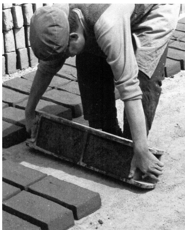
Figure 3.85. Using techniques similar to those shown in Figure 3.84, workers in western Shanxi province place moistened loessial soil into a double nonreleasable mold (top left), smoothening it with the hands before trimming it with a bow-shaped wire cutter (top right). Two uniform bricks are dumped from the frame and left to cure in the April sun (bottom). Lishi xian, Shanxi. [Original photographs used with the permission of Arthur J. Van Alstyne 1982.]
