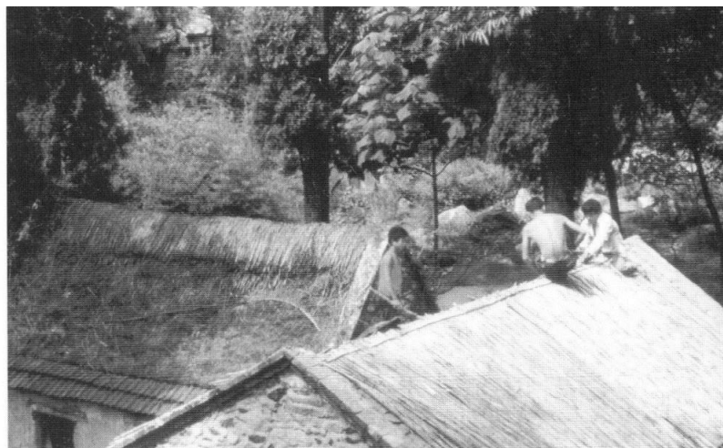
Figure 3.148. In preparation for laying a thatched roof on these stone mountain dwellings, a base of kaoliang stalks is being placed on the roof rafters. Taishan, Shandong. [RGK photograph 1985.]
