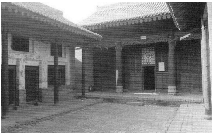
Figure 3.5. Throughout the Ming and Qing dynasty courtyard units in Dingcun, the podium of the main structure is elevated above those of side halls. The drip line for each overhanging roof plane leads rainwater into the sunken courtyard. A stone slab is needed as a step from the courtyard to the podium of the three- jian rear hall. Dingcun, Xiangfen xian, Shanxi. [RGK photograph 1993.]
