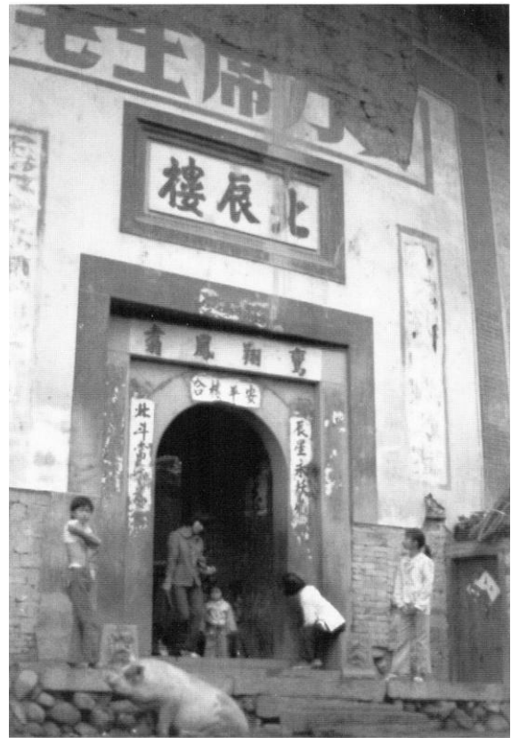
Figure 2.95. The entry to large Hakka yuanlou complexes, discussed in detail in Chapter 5, is normally through a single gateway. At Beichenlou , the gateway is heavily fortified. Framed with granite blocks, the wooden door panels are more than ten centimeters and are encased with an iron skin and reinforced with iron rods. Above the arch-shaped portal, the entry is a focal point for calligraphy. In addition to the bold characters of the name of the complex and couplets added at the New Year, fading characters reveal the ardor of recent revolutionary times. Fujian. [RGK photograph 1990.]
