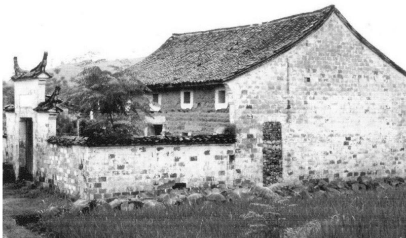
Figure 2.16. The walled courtyard of this rectangular two-story dwelling is entered through an imposing gate. The presence of a bricked-in doorway on the end of the structure suggests the anticipation of an additional bay or perpendicular wing. Nantang xian , Dongyang xian , Zhejiang. [RGK photograph 1987.]
