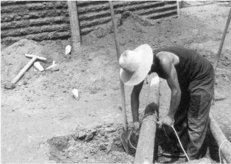
Figure 3.65. With the corrugated wall behind him, this worker is using a rope to scrape accumulated earth from one of the shuttering poles in order to create a tight fit. A stone rammer with its wooden handle rests on the earth. Xi'an area, Shaanxi. [RGK photograph 1984.]
