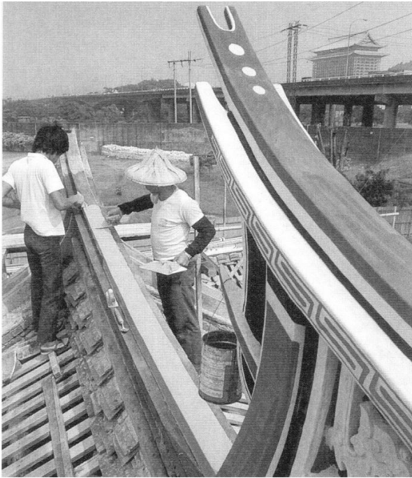
Figure 3.141. The massive size of some “swallowtail” ridgelines can be seen from this illustration of work being done to reconstruct the roof atop the Antai Lin dwelling. Yuanshan, Taipei, Taiwan. [Source: Tseng 1988a, 51.]
