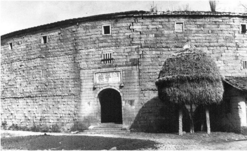
Figure 3.110. Shengpinglou is the only three-story circular fortress that is made completely of stone. Built in 1601, the circular walls are formed of battered granite slabs, decreasing in depth from approximately 2.05 meters at the base to 0.86 meters near the top. Baoshan cun, Shajian xiang, Hua'an xian, Fujian. [Original photograph used with the permission of Li Yuxiang.]
