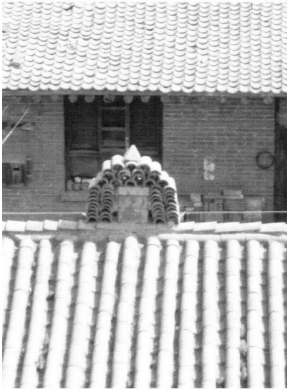
Figure 3.138. Using stacked tubular or flat roof tiles, the ridgeline of these dwellings is both functional and ornamental. Left, Pingyao shi , Shanxi; right, Langzhong shi , Sichuan. [RGK photographs 1996, 1993, respectively.]
