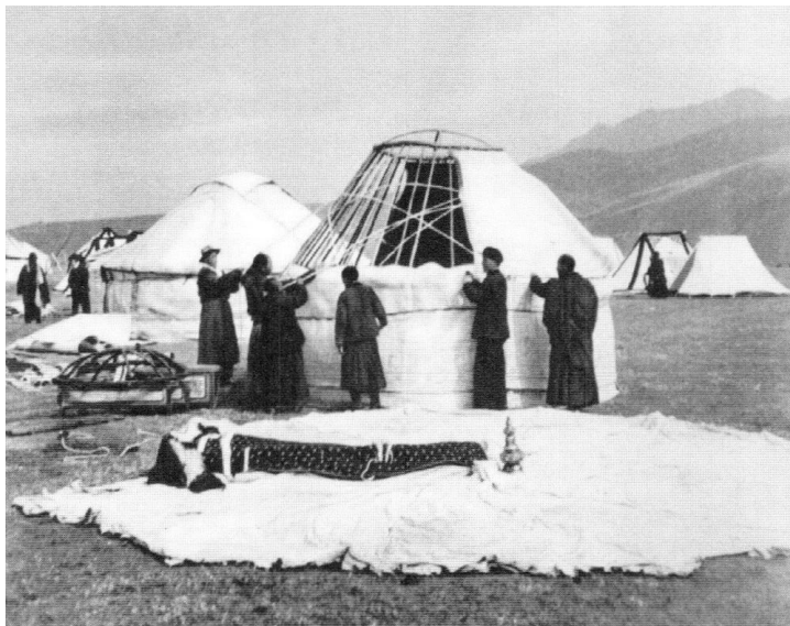
Figure 6.29. Building a Mongol ger involves first assembling the wooden framework, then wrapping it with felt panels that are strapped together with cords. Inner Mongolia. [Source: Zhongguo kexueyuan 1957, 75.]
