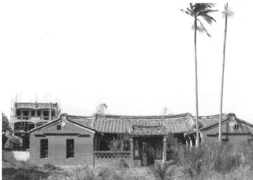
Figure 2.35. The courtyard contained within this inverted U-shaped sanheyuan is defined by a low wall, which is entered through a central gate. A new three-story dwelling rises beyond the dilapidated and abandoned traditional farmhouse. Zhanghua xian , Taiwan. [RGK photograph 1993.]
