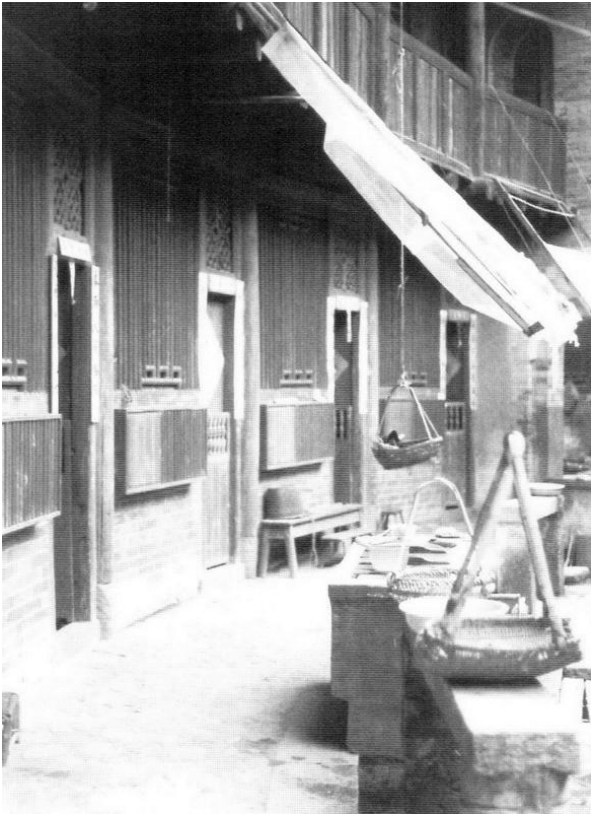
Figure 5.76 (top left). Each of the ground-level units along the outer wall is entered through an individual doorway. The units are apportioned equally and are similar in size. Zhenchenglou, Hongkeng cun , Hukeng xiang , Yongding xian , Fujian. [RGK photograph 1990.]
