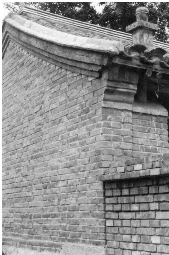
Figure 3.93. Two different brickwork bonds are seen here. Built of fired brick, the gable wall is composed of stretchers—courses with staggered tight joints. The low courtyard wall extending forward from the dwelling, however, is composed of an “English bond”—alternating courses of headers and stretchers. Huairou xian, Beijing. [RGK photograph 1987.]
