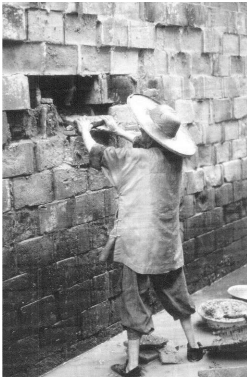
Figure 3.95. As individual bricks in a kongdou wall become dislodged, they can be repaired relatively easily if replacement bricks are available. Here, the worker is pounding earth into some of the open cavities between the thin bricks in order to strengthen the wall. Bihu zhen , Lishui xian , Zhejiang. [RGK photograph 1987.]
