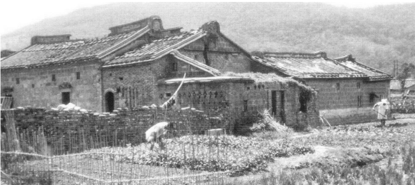
Figure 3.142. “Horseback,” or “saddle,” style ridges [ mabeixing ] maintain a low slung curved ridgeline like the “swallowtail” style but lack the upward sweep at the ends of the roof ridges. Instead, each of the upper gables is an elevated geometric shape. Shilin zhen, Taipei, Taiwan. [RGK photograph 1965.]
