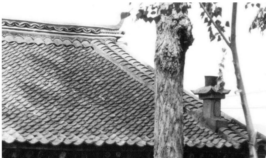
Figure 3.159. Scalelike in appearance and function, the tile surface sheds water rapidly. Huairou xian , Beijing. [RGK photograph 1987.]
