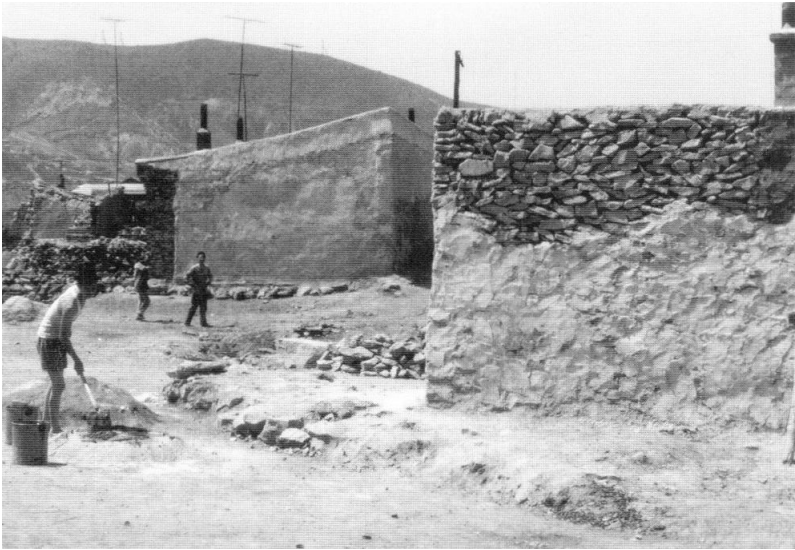
Figure 3.103. Along the margins of the Great Wall in northern Shanxi and northern Hebei, where soils are thin and wood is lacking, simple single-sloped-roof structures made of small stones are common. To finish the surface and prevent the penetration of cold air and moisture, the stone is coated with a lime-and-mud plaster. Datong area, Shanxi. [RGK photograph 1985.]
