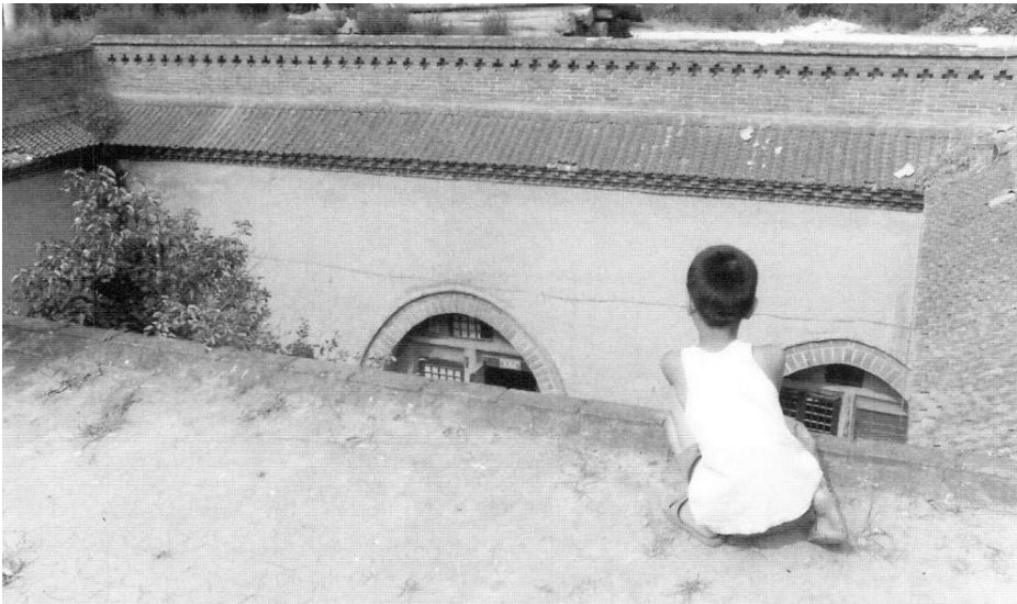
Figure 4.80. Only 10 centimeters high, this low parapet minimizes the amount of surface dust that can blow down into the courtyard. Faced with brick and constructed with a sloping band of “roof tiles” to keep rainwash from the walls, this upper wall treatment provides major protection. Houwang cun , Pinglu xian , Shanxi. [RGK photograph 1996.]
