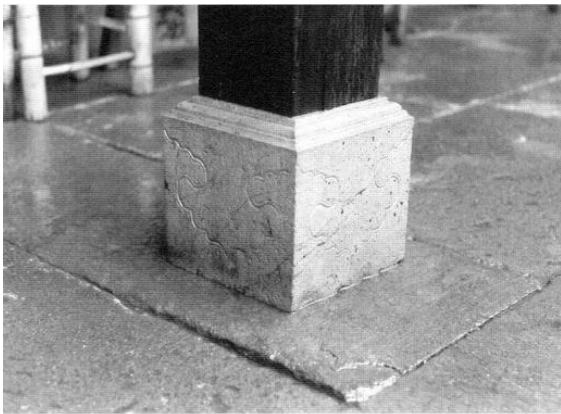
Figure 3.13 (above). Supporting a wooden pillar holding up a roof overhang, this simple stone base rests on a thin piece of square stone set into the earthen floor of this modest dwelling. A matching base along the wall is just beyond the pig's head. Shuitou xiang , Cangnan xian , Zhejiang. [RGK photograph 1988.]
