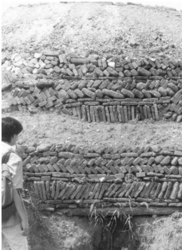
Figure 3.89. Zhuanyao , or “brick kilns,” vary from place to place, although they share many common characteristics. Most are dug into the ground, lined with stone blocks, covered with earth and old bricks, and entered either from the front or above. Near Guilin, Guangxi Zhuang Autonomous Region. [RGK photograph 1985.]
