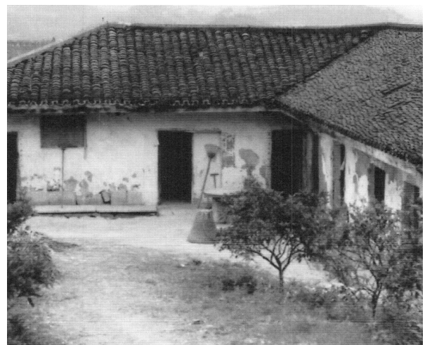
Figure 5.7 (middle right). Without an eaves overhang wide enough to shade the dwelling and shed rainwater away from the foundation and walls, this rectangular dwelling in the eastern part of the province has many similarities to northern prototypes, including being built directly on the ground. Its depth and width, its loose tile roof, and its siting near a windbreak grove of bamboo, however, reveal some attention to subtropical conditions. Near Chongqing, Sichuan. [RGK photograph 1983.]
