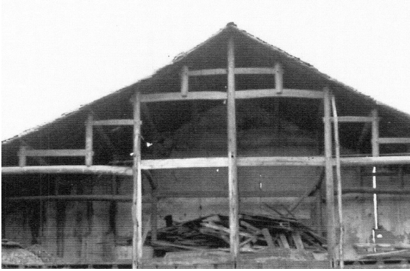
Figure 3.25 (above). In the process of being demolished, the internal chuandou frame of this two-story structure with a loft is apparent. Five thin pillars run from the ground to the roof purlins and are assisted by six shorter posts that do not reach the ground but are instead tied to principal load-bearing pillars by mortised and tenoned tie beams. Lubu cun , Shuidong xiang , Lishui xian , Zhejiang. [RGK photograph 1988.]
