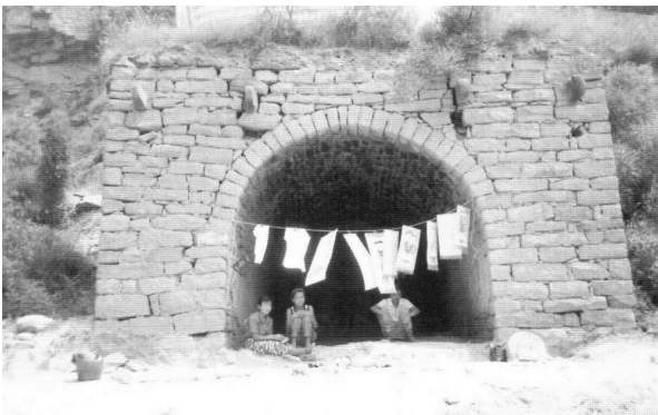
Figure 3.111 (above). On the western margins of Shanxi province that drain into the Huanghe River, there is a virtual absence of building materials except for sandstone and compacted loessial soil that can be cut into blocks. Cavelike structures constructed of rough stone blocks line terraces in Hukou, Jixian, Shanxi. [RGK photograph 1996.]
