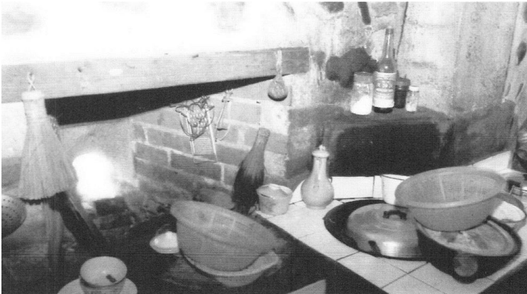
Figure 5.102. No longer needed for surveillance or for shooting rifles, this gun port has been reconfigured as an exhaust for a small stove. Southern Jiangxi. [RGK photograph 1993.]
