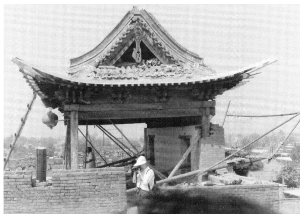
Figure 4.48 (bottom left). One of several pavilions that are perched atop the tall building blocks along the north side of Cao manor. With rooflines more akin to palaces than the dwellings below, the pavilions create prospects for enjoying the scenery and catching the breeze. Beiguang, Taigu, Shanxi. [RGK photograph 1996.]
