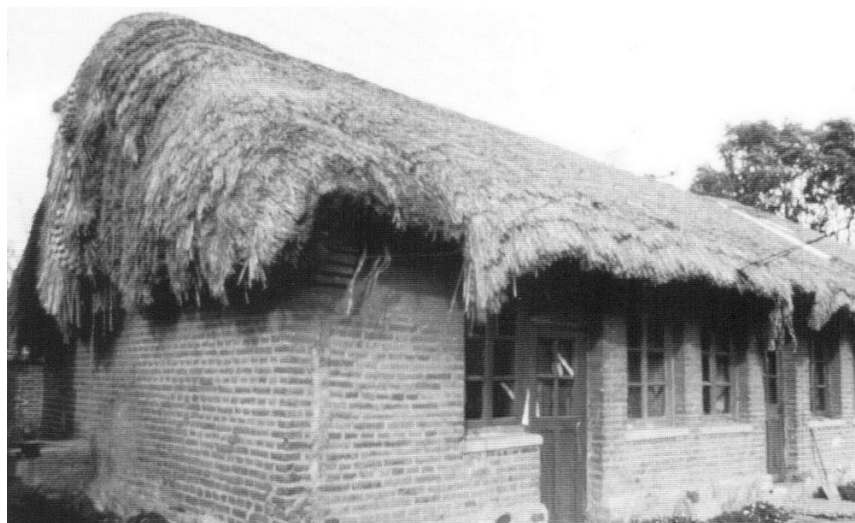
Figure 3.147. Thatched roofs are sometimes added to new brick dwellings in northeast China, a temporary solution until additional resources become available for a tile roof. Jinjiawan, Dongling qu , Shenyang, Liaoning. [Original photograph used with the permission of Elizabeth Leppman 1994.]
