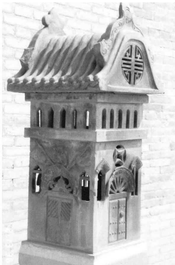
Figure 4.39. An elaborate heating system in the Qiaojia manor necessitates a large number of high chimneys, some of which are elaborately ornamented with architectural and propitious motifs. Qiaojia dayuan, Qixian, Shanxi. [RGK photograph 1996.]
