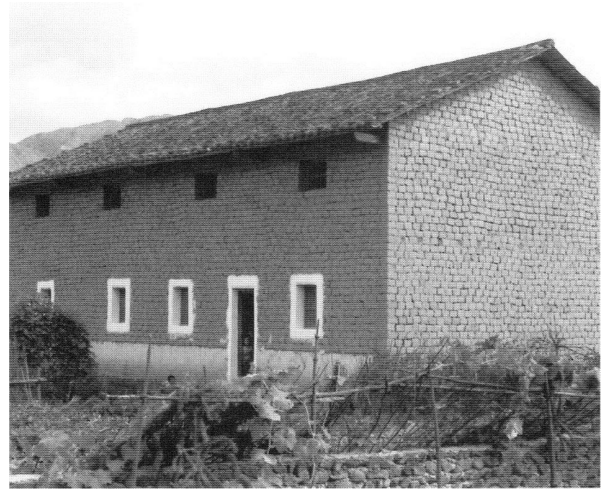
Figure 3.82. The weighty adobe brick walls are mere curtain walls in this large dwelling, as a chuandou frame is lifting the roof structure. Guanxi xian , Longnan xian , Jiangxi. [RGK photograph 1993.]
