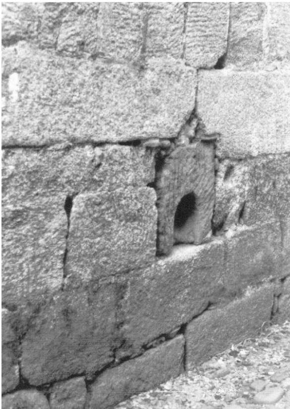
Figure 3.10 (top right). Raised a half-meter above ground level to protect the dwelling from heavy rains characteristic of this area of southeastern China, this mortared stone foundation also provides sufficient support for the heavy walls of fired brick around the outside as well as those used to form the inner walls. Near Guilin, Guangxi Zhuang Autonomous Region. [RGK photograph 1985.]
