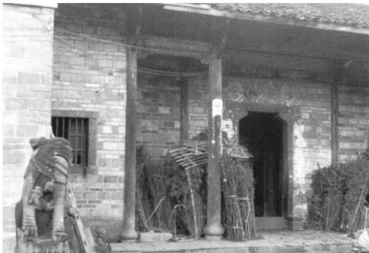
Figure 5.92 (left). Interior structures are made of high-quality fired bricks with an abundant use of wooden columns and beams as well as clay tiles, all of which echo building norms elsewhere in China. [RGK photograph 1993.]
