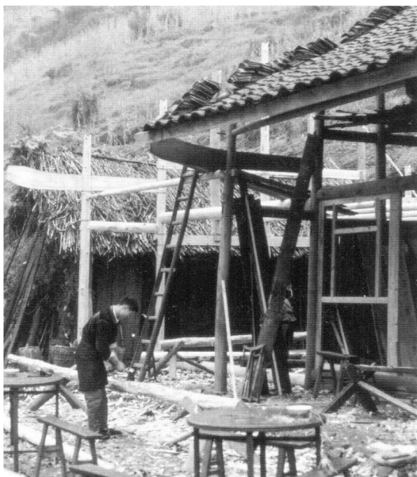
Figure 3.31 (top left). Completed in a series of modular segments, each of the front-to-back and side-to-side building elements is tied together with wooden members. As this photograph demonstrates, the heavy tiled roof surface is completed well before the enclosing curtain walls are raised. Foothills of Emeishan, Sichuan. [RGK photograph 1984.]
