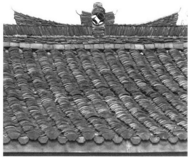
Figure 3.138. Using stacked tubular or flat roof tiles, the ridgeline of these dwellings is both functional and ornamental. Left, Pingyao shi , Shanxi; right, Langzhong shi , Sichuan. [RGK photographs 1996, 1993, respectively.]
