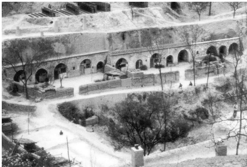
Figure 4.52. Shaved to shear verticality, this cliff face was tunneled to create thirteen yaodong of varying heights, widths, and depths. The excavated earth was used to form a level terrace and tamped to form a low wall around a courtyard. To inhibit deterioration, a brick and stone facade and an overhanging cap were added. Lishixian, Shanxi, 1982. [Original photograph used with the permission of Arthur J. Van Alstyne.]
