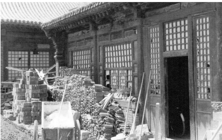
Figure 3.58. Each of the four structures surrounding this narrow courtyard of the Cao family is composed of wooden lattice panels and doors set between the columns. The square pattern of the lattice panels is papered on the inside. Caojia manor, Taigu, Shanxi. [RGK photograph 1996.]
