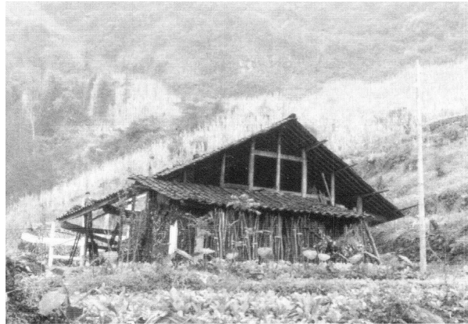
Figure 3.30. Viewed from the completed gable end, this large farmhouse has a chuandou framework comprising seven sturdy pillars that rise to support the roof purlins. Three center pillars are stabilized via a transverse tie beam high in the frame while four transverse tie beams beneath link the two additional pillars. Foothills of Emeishan, Sichuan. [RGK photograph 1984.]
