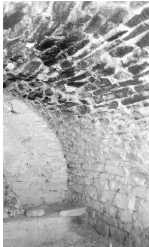
Figure 3.112 (left). Here, and elsewhere in the region, guyao structures are constructed of blocks of locally available stone that is held without mortar. Hukou, Jixi'an, Shanxi. [RGK photograph 1996.]
