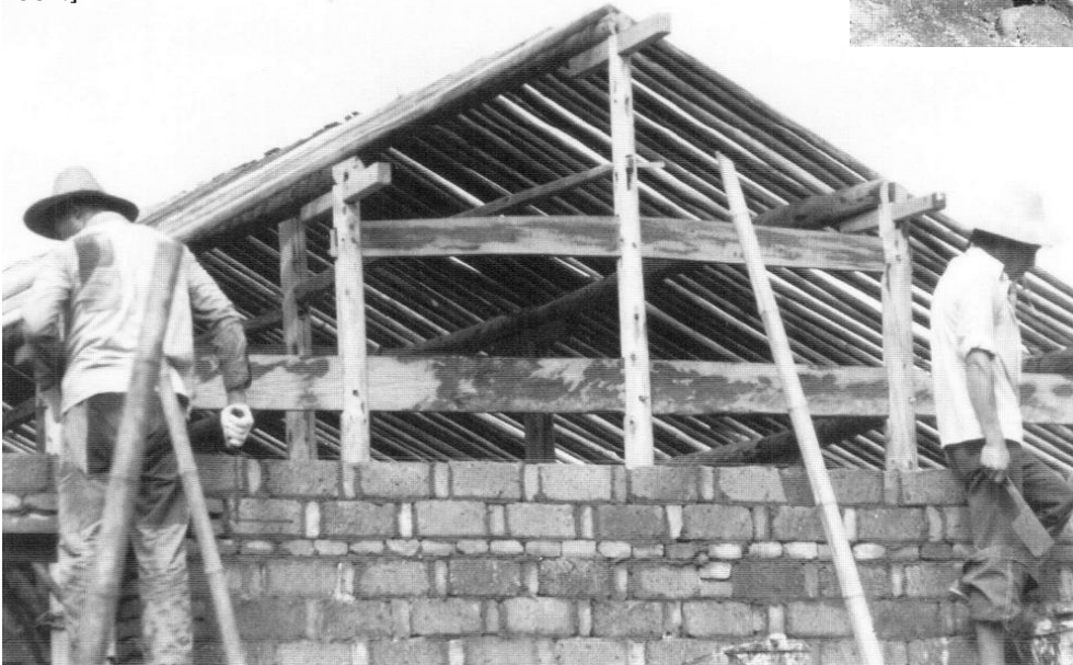
Figure 3.61 (bottom). These masons are raising a brick curtain wall around the outside of a load-bearing chuandou wooden framework that is supporting the roof structure. Changle cun, Zhuge xiang, Lanxi shi, Zhejiang. [RGK photograph 1987.]
