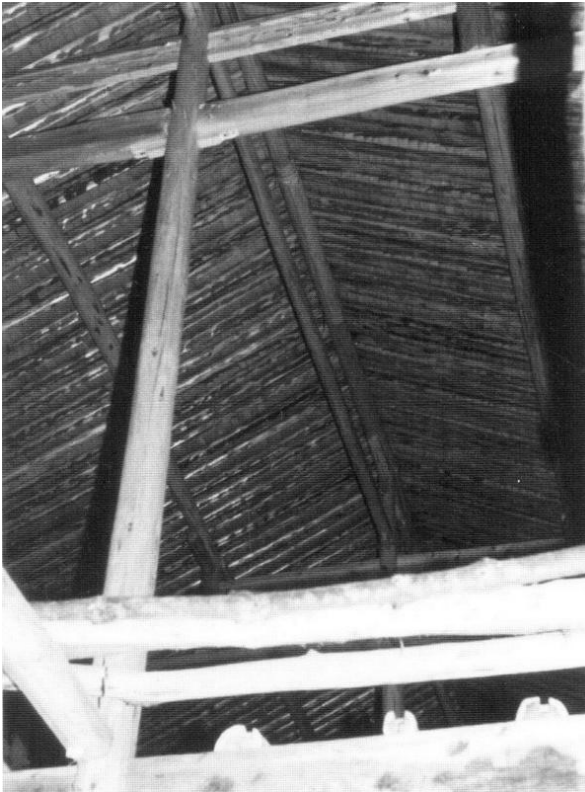
Figure 3.43. Reaching more than 8 meters from floor to ridgepole, this center column of a chuandou frame is a substantial and costly timber. Only the upper half of the timber column is visible. Near the bottom, floor joists have been added to make possible a second floor. Changle cun , Zhuge xiang , Lanxi shi , Zhejiang. [RGK photograph 1987.]
