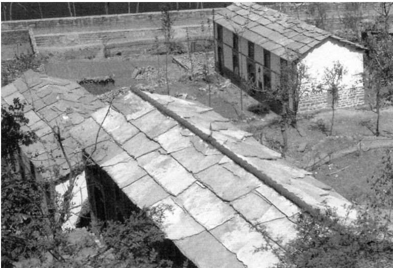
Figure 3.178. When available, large sheets of slate are used for roofing even new two-story dwellings. Northwestern Henan. [Original photograph used with the permission of Arthur J. Van Alstyne.]
