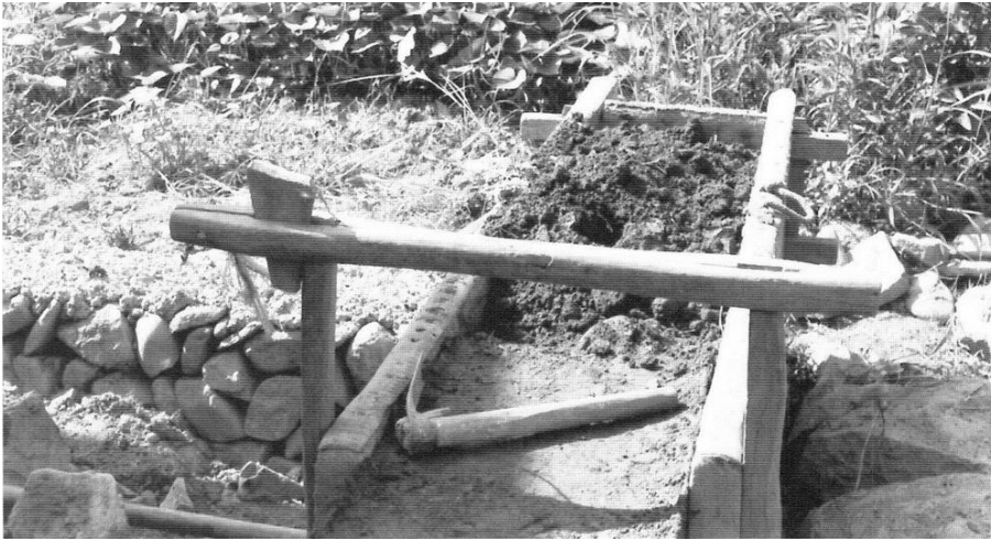
Figure 3.67 (left). Here one man adds the soil mixture while the other tamps it firmly. Shangshan cun , Yangcunqiao xiang , Jiande xian , Zhejiang. [RGK photograph 1987.]
