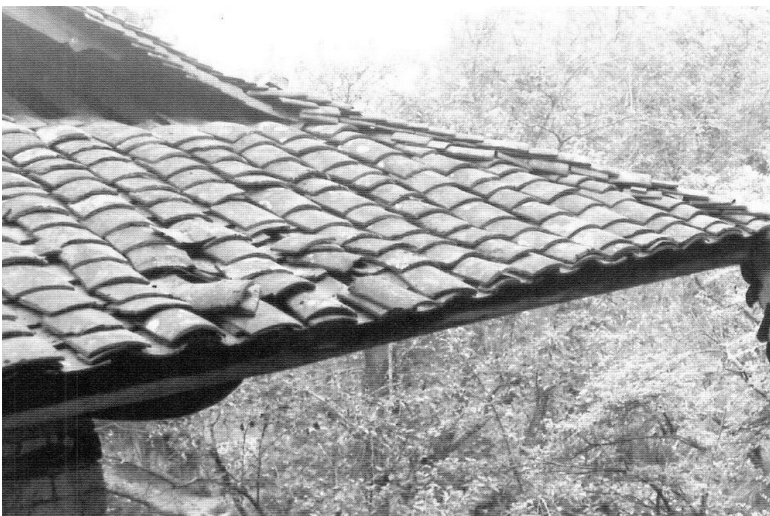
Figure 3.164 (bottom left). Large and slightly bent tiles of uniform shape and size are set on the roof of this Hakka fortress. Gaobei cun , Guzhu xiang , Yongding xian , Fujian. [RGK photograph 1990.]
