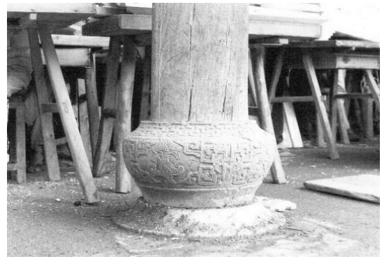
Figure 3.14 (above). Both the carved stone column base and pedestal beneath are set on a raised stone podium. Zhiyan xiang , Lanxi shi , Zhejiang. [RGK photograph 1987.]
