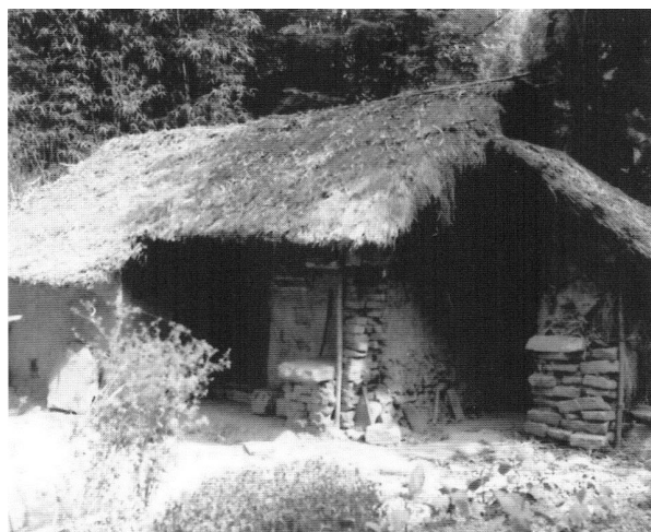
Figure 5.9. A dweller-built house of piled stone, adobe brick, and thatch, this modest dwelling is found atop a hill. The old owner maintains his own kitchen garden at the front door. Zhuangyuan cun , near Langzhong, Sichuan.
