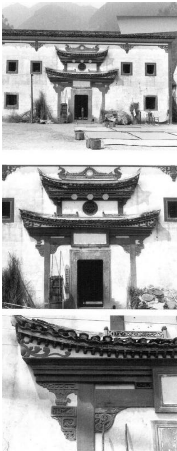
Figure 2.89. Built early in the twentieth century, conspicuous menlou dominate the facade of this tianjing -style dwelling. The carved brick and stone of this menlou imitate wooden structural and ornamental elements. The type of materials used is not apparent until one nears the gate. Maoping cun , Luci xiang , Tonglu xian , Zhejiang. [RGK photograph 1987.]
