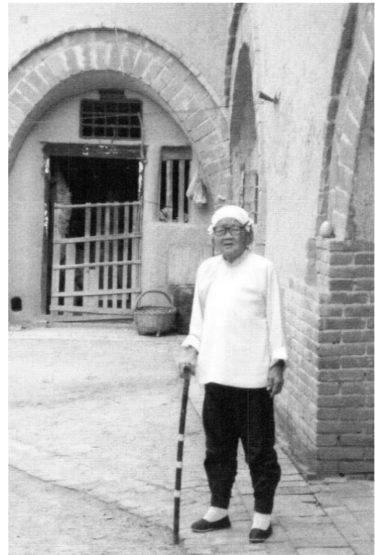
Figure 4.76 (bottom right). An arch of brick or stone is often used today in order to help stabilize the weakened wall where excavation has given shape to a room. Along the plane where two arches join, a pier adds further support. A path of brick rings the courtyard, and several shortcuts paved with brick cross it. Houwang cun , Pinglu xian , Shanxi. [RGK photograph 1996.]
