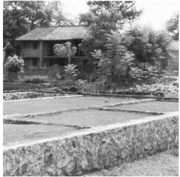
Figure 3.9 (top left). In this recent construction, footing channels were dug into the ground and filled with stone of various sizes in order to create a firm and deep base for a structure that will be built on grade. Xishansi cun , Lingdong xiang , Lanxi shi , Zhejiang. [RGK photograph 1988.]
