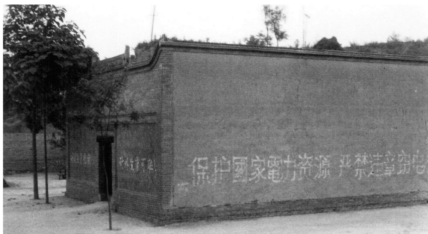
Figure 4.24. The long, high blank wall comprises the back of one of a pair of xiangfang whose roofs slope inward to the interior courtyard. Entry is through a central gate in the southern wall and leads to a three-jian-wide zhengfang . Fenghuo xiang, Liquan xian, Shaanxi. [RGK photograph 1991.]
