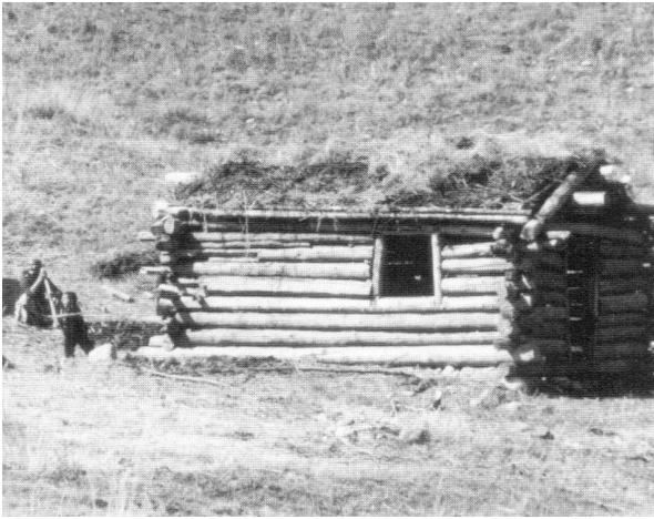
Figure 3.118. Rather crudely stacked jinggan , or “well frame” single-room log houses, are built by Kazak herders to supplement their mobile yurts. Northern slopes of Tianshan, Xinjiang Uygur Autonomous Region. [RGK photograph 1984.]
