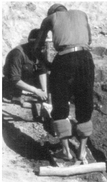
Figure 3.86. Thin bricks of coal dust and mud are formed in small molds. The hand-shaping of bricks in Xinjiang is accomplished with small rudimentary molds on level ground. The poor quality thin brick product is typically used only for low walls, foundations, and floors throughout northwestern China. Xinjiang Uygur Autonomous Region. [RGK photograph 1985.]
