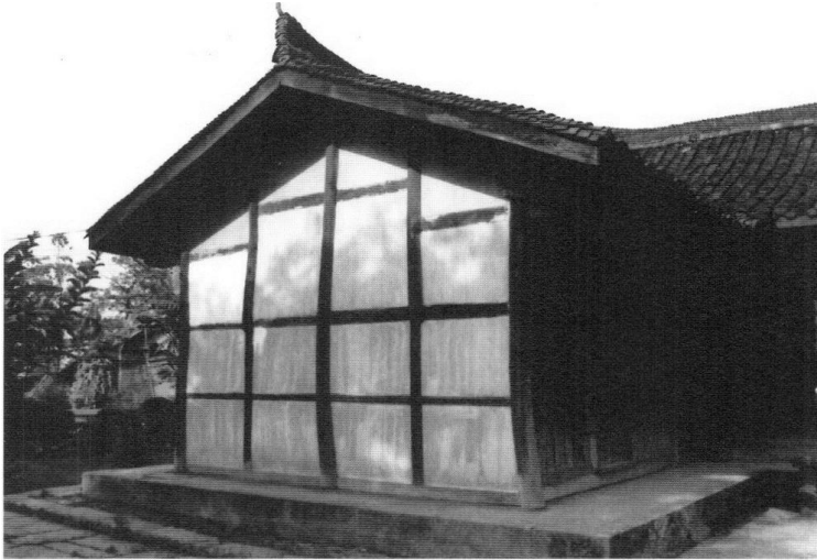
Figure 3.4. The stone podium beneath this open U-shaped sanheyuan extends beyond the drip line of the roof, thus leading water away from the lower walls. Shuangnushi cun, Wufeng xiang, Nanchong, Sichuan. [RGK photograph 1994.]
