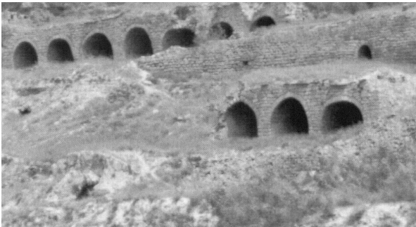
Figure 3.111 (above). On the western margins of Shanxi province that drain into the Huanghe River, there is a virtual absence of building materials except for sandstone and compacted loessial soil that can be cut into blocks. Cavelike structures constructed of rough stone blocks line terraces in Hukou, Jixian, Shanxi. [RGK photograph 1996.]
