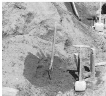
Figure 3.87. Similar to the tamping of earthen walls, bricks can be formed in releasable molds using the pressure of the feet or stone hand rammers. West of Lanzhou, Gansu. [RGK photograph 1985.]
