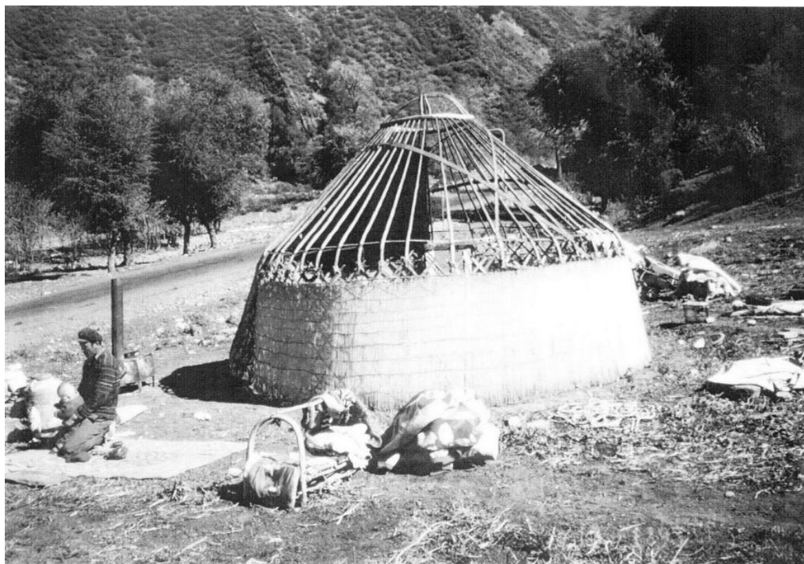
Figure 6.26 (bottom). Kazak tents, called ki-giz öy in Kazak, can be assembled and dismantled easily. The outer form is defined by a latticelike frame of pliant and braided willow saplings that can be stretched and rolled. Once the accordionlike frame is fully engaged, the frame is covered on the outside with layers of felt made of matted sheep hair and lashed tightly with cord made of sheep or cattle hair. Tianchi, Xinjiang Uygur Autonomous Region, 1994. [Original photograph used with the permission of Stanley Toops.]
