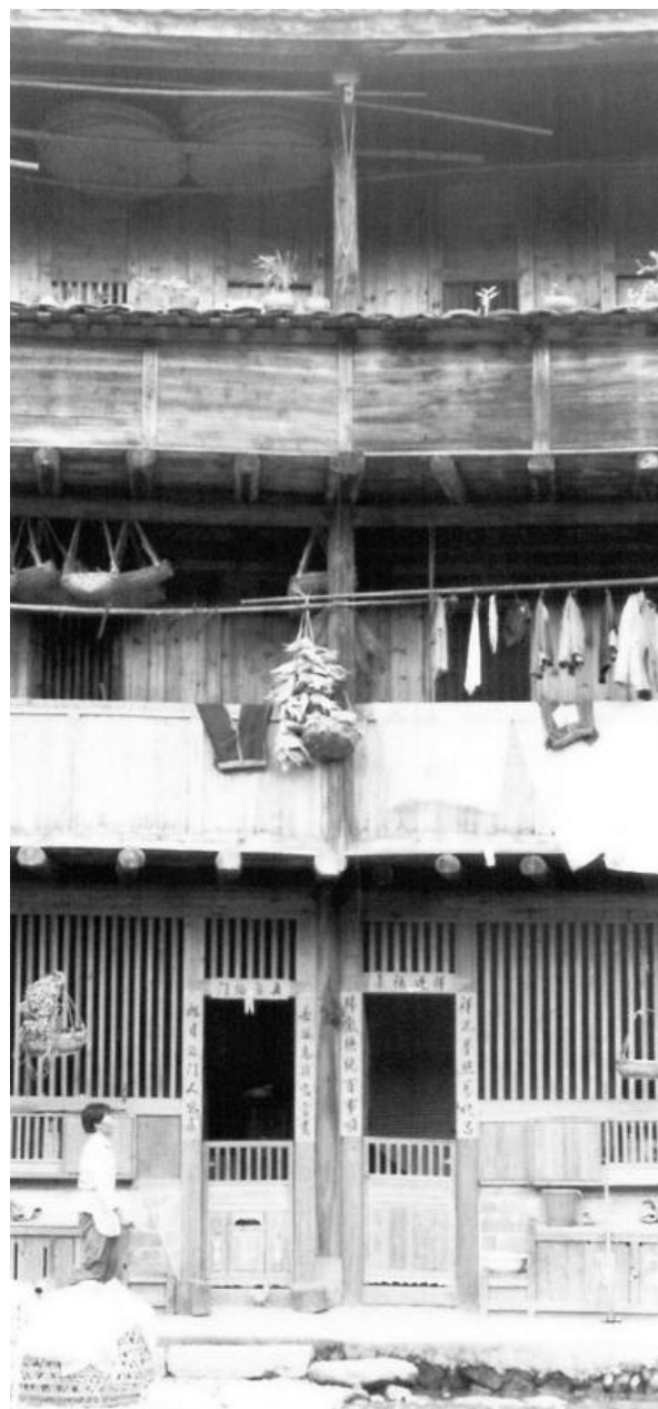
Figure 3.59. Although the exterior walls of Hakka and Hokkien fortresses are massive, the interiors are all made of wood. At whatever level, the space between the columns is filled with similar modular wooden open or closed panels. Hekeng cun , Shuyang xiang , Nanjing xian , Fujian. [RGK photograph 1990.]
