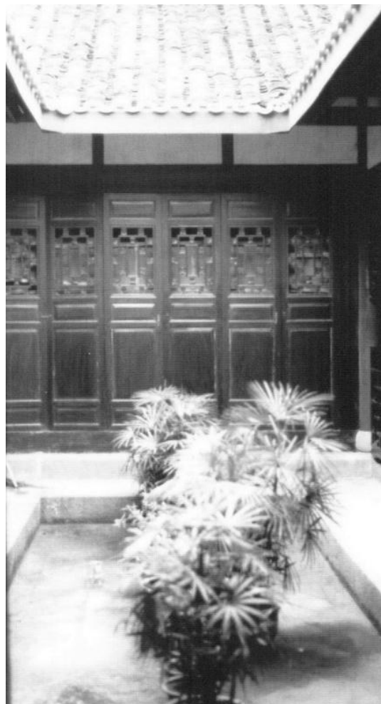
Figure 5.19 (right). From inside a room looking out across a small skywell, or tianjing , toward paneled doors that can be swiveled open or shut. The upper portion of each panel is made of carved lattice. Shuangjiang zhen, Tongnan xian, Sichuan. [RGK photograph 1995.]
