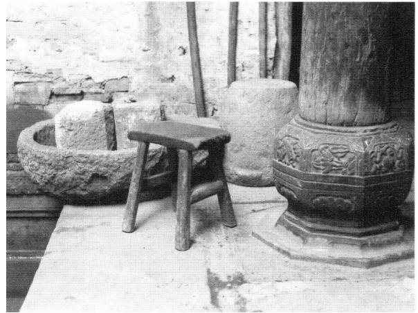
Figure 3.14 (above). Both the carved stone column base and pedestal beneath are set on a raised stone podium. Zhiyan xiang , Lanxi shi , Zhejiang. [RGK photograph 1987.]
