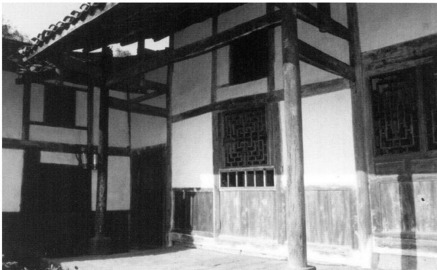
Figure 3.28. Mortise and tenon chuandou frames easily accommodate the extension necessary to project substantial eaves overhangs in areas of heavy rainfall. Sichuan. [Source: Liu Zhiping 1957, 295.]
