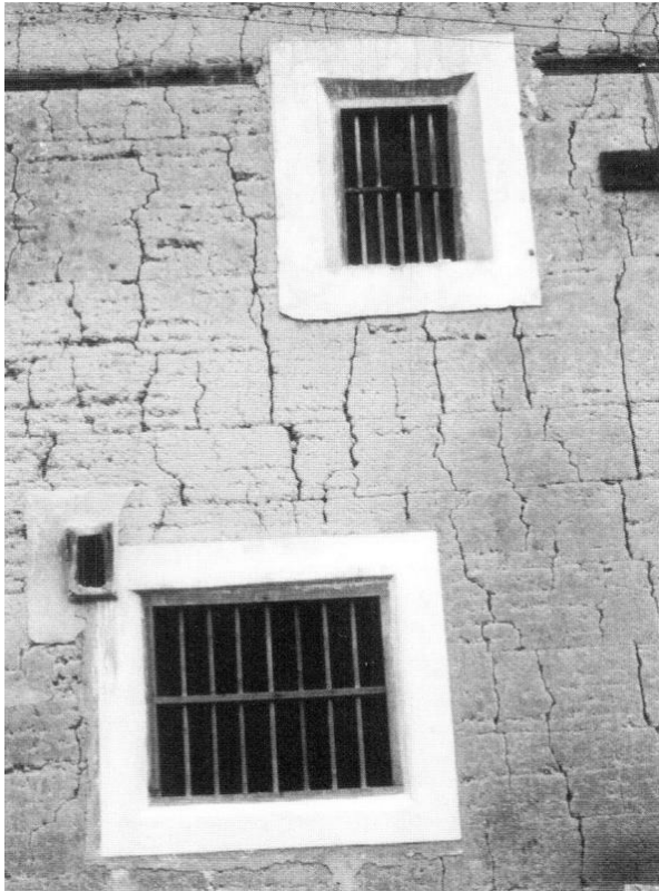
Figure 3.78. To increase ventilation, new window openings are sometimes cut into the thick lower walls of older structures. The rather random patterns apparently disregard the diminishing of structural stability. Nanjing xian , Fujian. [RGK photograph 1990.]
