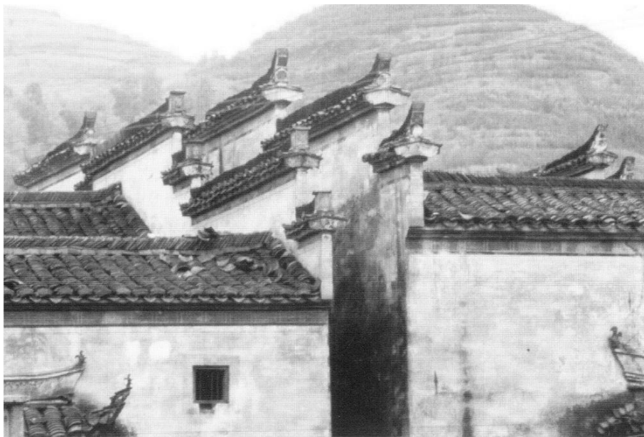
Figure 3.128. Matouqiang , or “horses’ head walls,” rise in steps above the roofline. Originating as firewalls, they came into wide use during the Ming period as fired bricks became relatively inexpensive. They are found on dwellings as well as temples, clan halls, and other buildings. Dafu xiang , Shexian, Anhui. [RGK photograph 1987.]
