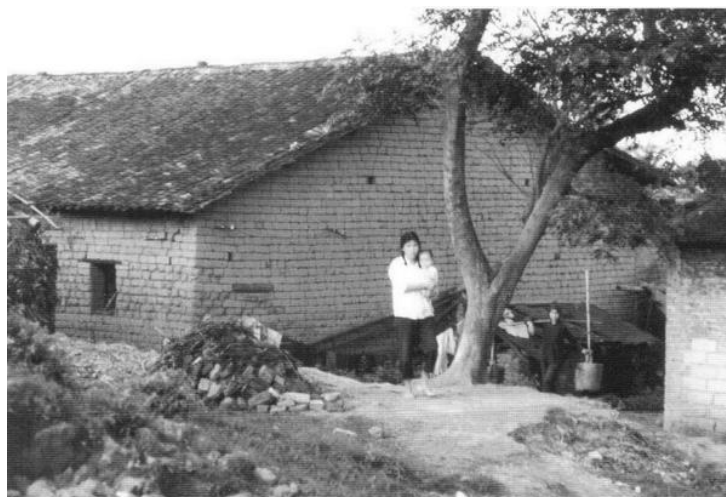
Figure 3.97. With increased resources, a village household has built a fired brick dwelling (bottom) that is essentially a duplicate of their adobe house (top). Guilin area, Guangxi Zhuang Autonomous Region. [RGK photographs 1984.]
