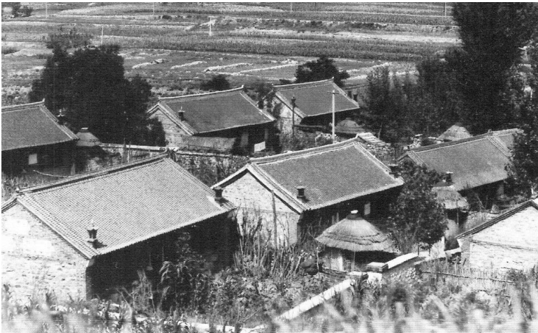
Figure 4.2. A cluster of dwellings made of stone in a nucleated village in northern Hebei province. Each danzuo pingfang dwelling faces south and has a walled courtyard at its front. Within the courtyard is a haystack, kitchen garden, and a latrine. [RGK photograph 1984.]
