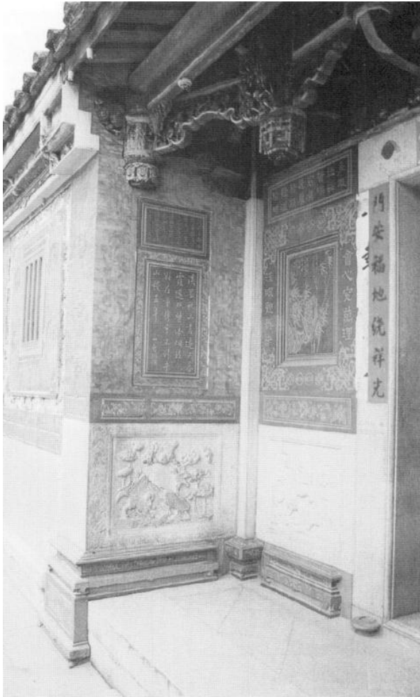
Figure 2.94. Recessed entries are called “mendou.” While many are not much wider than the doorway itself, others are broad. This entryway is heavily ornamented with carved wood, stone, and brick elements. Yang Amiao dwelling, Quanzhou, Fujian. [Source: Lu and Lu 1992, 34.]
