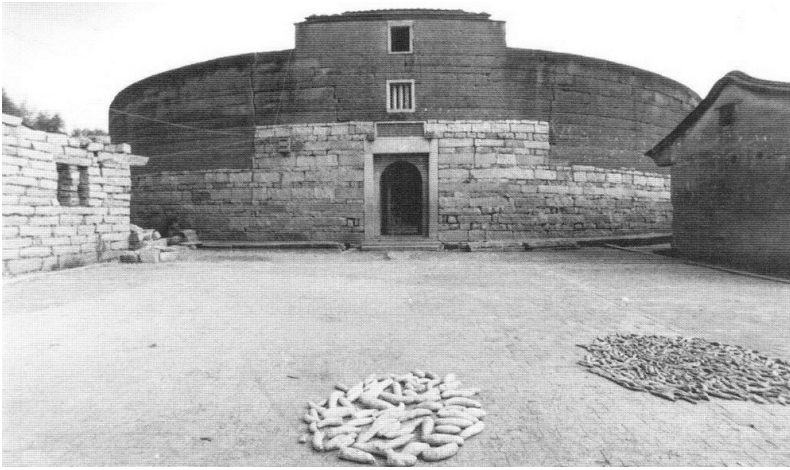
Figure 3.108. As seen around the front gate, substantial portions of the lower walls of Jinjianglou are constructed of cut stone slabs to increase the wall's strength. The gate leads into a second concentric ring of the structure. Jinjiang cun , Shentu xiang , Zhangpu xian , Fujian. [Original photograph used with the permission of Li Yuxiang.]
