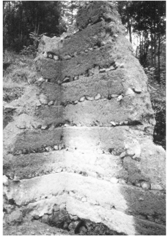
Figure 3.72. In this decaying wall, small stones and other substances are sometimes placed within the rising wall to stabilize it as well as to facilitate the drying of the various layers. Moganshan, Jiaxing xian , Zhejiang. [RGK photograph 1983.]
