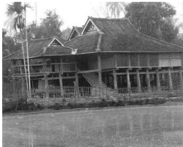
Figure 5.107. Zhulou were originally built of bamboo but are now usually constructed of sturdy wooden poles, as seen in this close-up. The floor is elevated above the ground, while space beneath is left unwallled. High roofs and porous walls of the enclosed portion allow air to circulate. Ganlanba cun , Jinghong xian , Xishuangbanna Dai Autonomous Prefecture, Yunnan. [Original photograph used with the permission of Zhu Liangwen.]
