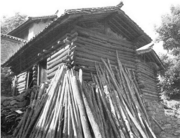
Figure 3.119. The Yi, as with other southwestern nationality minority groups, such as the Nu, Pumi, Drung, Lisu, and some Naxi and Tibetans, build some of their dwellings out of logs. Usually without windows, Yi log dwellings are rectangular, U-shaped, and L-shaped and are often built on hillsides on level stone foundations. Xi-aopenhe cun , Nanhua xian , Chuxiong Yi Nationality Autonomous District, Yunnan. [Original photograph used with the permission of Asakawa Shigeo 1992.]
