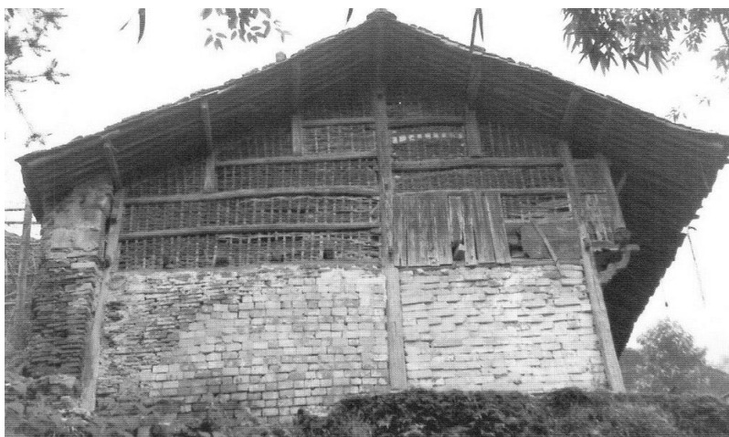
Figure 3.46. Split bamboo panels in various sizes and shapes are cut to fit the upper interpillar spaces where their light weight and porosity are advantageous. Wanyao cun , Zhuxi xian , Cangnan xian . [RGK photograph 1988.]
