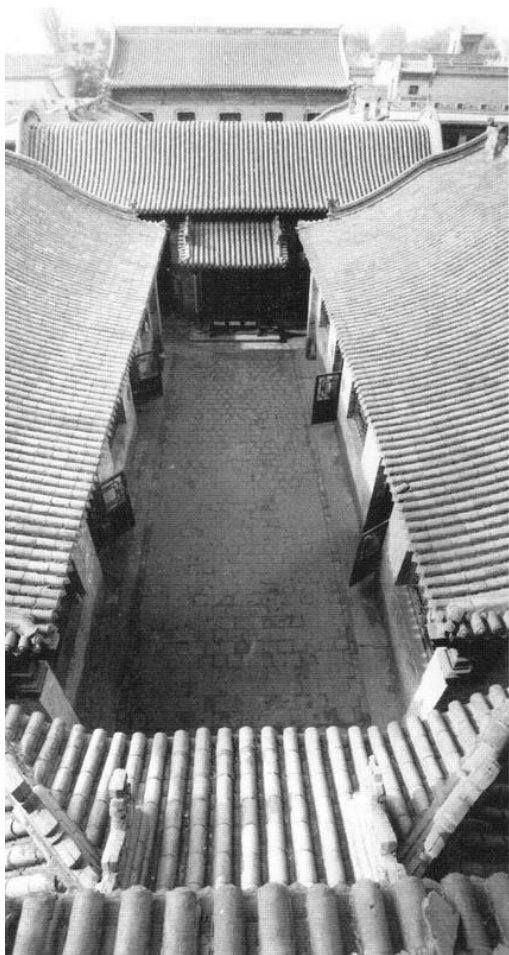
Figure 4.34 (above). View from the northernmost rooftop of the complex back across a narrow courtyard to the guoting , or “transitional hall,” that leads inward from another narrow courtyard. All roof slopes drain toward the stone-lined courtyards. Qiaojia dayuan , Qixian, Shanxi. [Original photo used with the permission of Li Yuxiang.]
