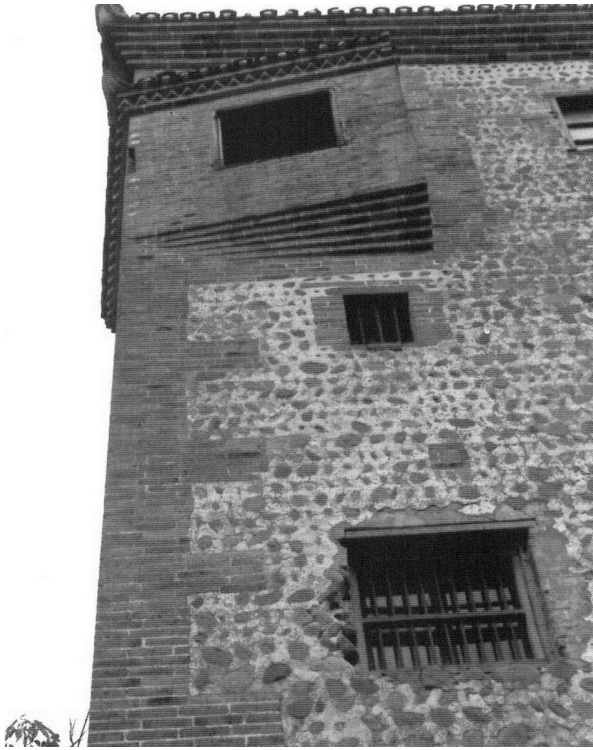
Figure 3.101. This multistory weizi fortress is framed in brick with a facing of stone and mortar infilling. On the interior is a wooden framework that serves to buttress the high walls. Shixing xian , Jiangxi. [RGK photograph 1993.]
