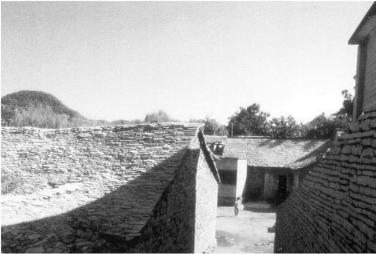
Figure 3.177. Overlapping slate fragments of many shapes and sizes are used as roof covering on this Buyi rock dwelling. Guizhou. [Original photograph used with the permission of Joseph Chuo Wang.]
