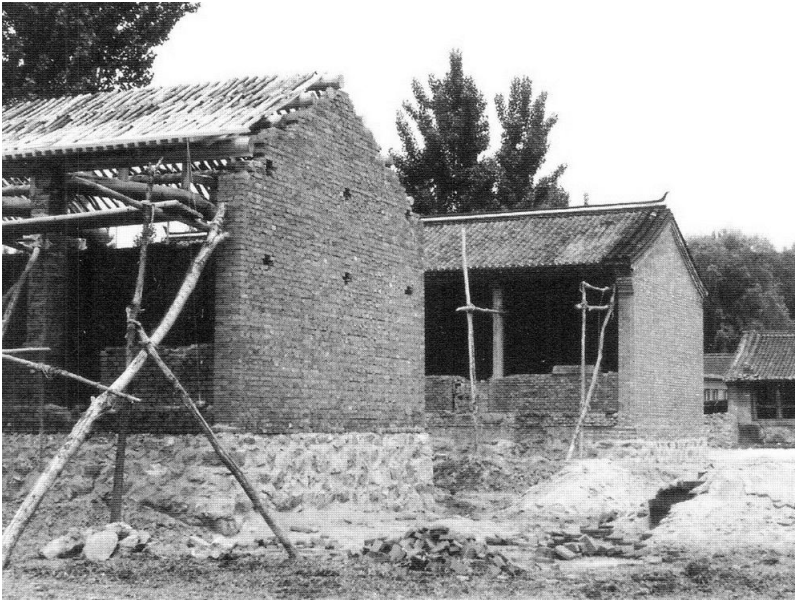
Figure 3.124. Two parallel dwellings show the load-bearing nature of the gable wall [ shanqiang or “mountain wall”] with the thick purlins resting directly on the wall. A small decorative detail accentuates the roof at this junction. Behind the two parallel dwellings is a structure that clearly has a yingshanding roof profile, with the upper triangular gable wall being flush with the end of the roof. This dwelling has the same roof details as the adjacent buildings. Huairou xian, Beijing. [RGK photograph 1987.]
