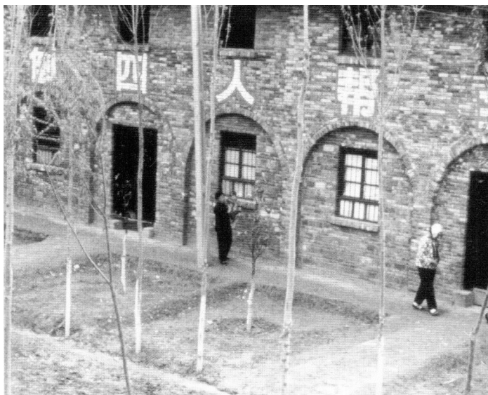
Figure 4.92 (bottom). These newly built two-story brick residential blocks resemble kaoshan yaodong found in the vicinity. The "smashing of the Gang of Four" upon the death of Chairman Mao in the fall of 1976 is marked by the slogan on the wall. Fenghuo, Liqun xian , Shaanxi. [RGK photograph 1977.]
