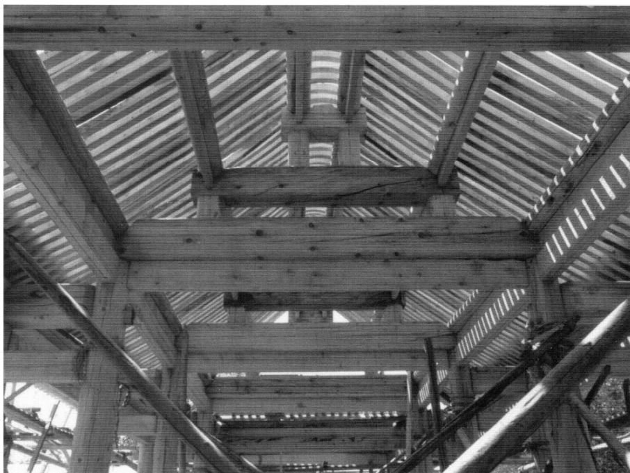
Figure 3.20. The massive timbers used in this structure include all common elements of a tailiang framework except that, instead of a single ridgepole, a pair of ridgepoles are used in order to make possible a slight roll to the crown of the roof. Xuanwumen Park, Beijing. [RGK photograph 1984.]
