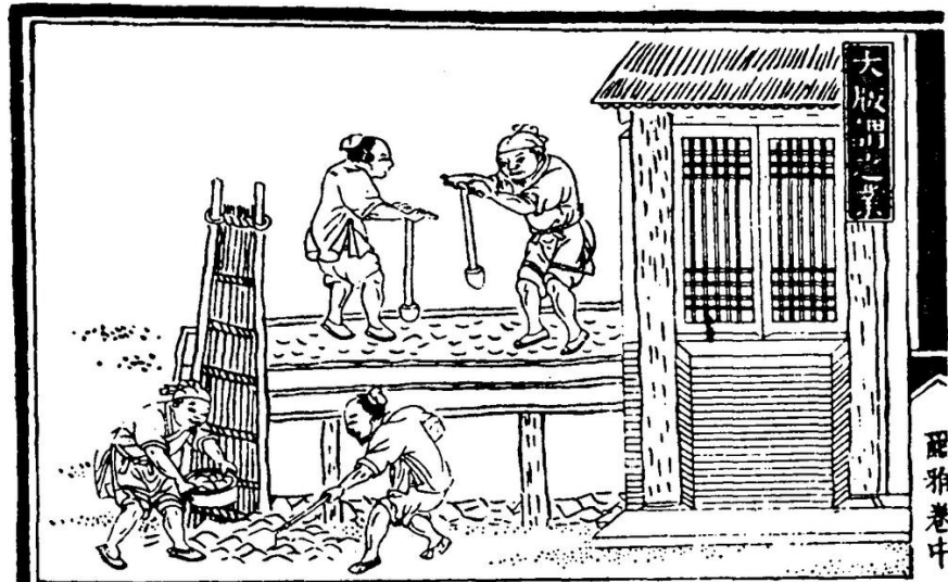
Figure 3.63. Seventeenth-century drawing of the tamped earth method of raising a wall. Walls of this type are called hangtu walls. [Source: Er ya , juan 2, 6b. After Needham 1971, 39.]
