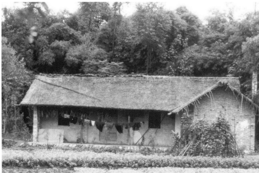
Figure 5.13. This L-shaped variant of a basic Sichuan dwelling has a steeply pitched roof that overhangs the walls and is constructed of a mixture of adobe and fired brick. Western Sichuan. [RGK photograph 1983.]
