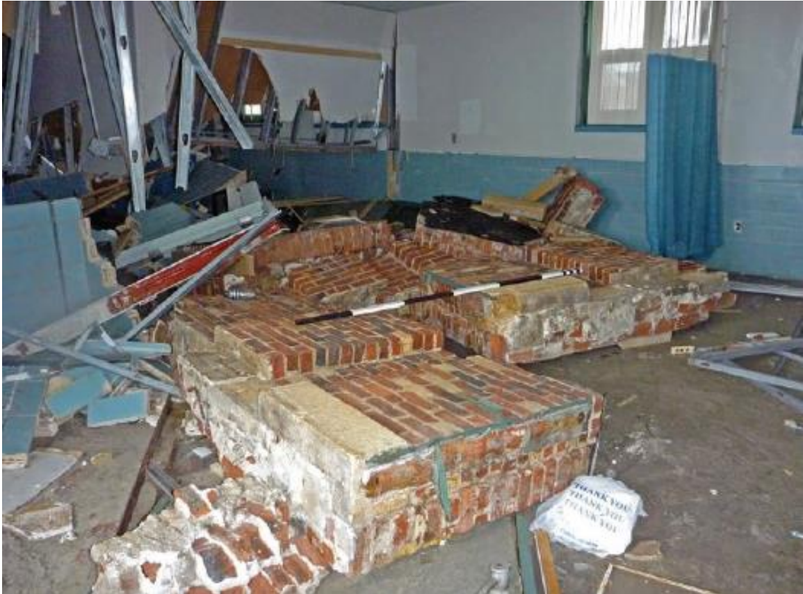
Figure 29 Solid Brick Wall Destroyed from Storm Surge Source FEMA P-942 p7-14
