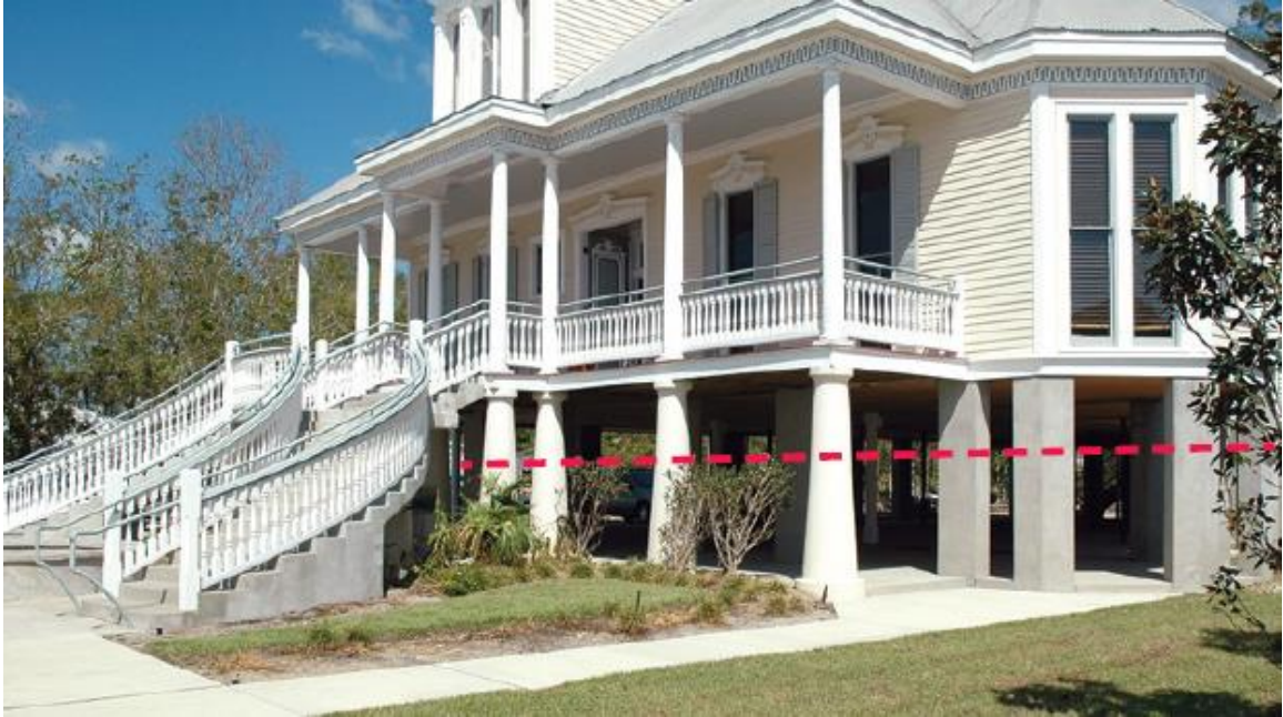
Figure 24 Properly Elevated and Anchored Building Source FEMA-549 p379
