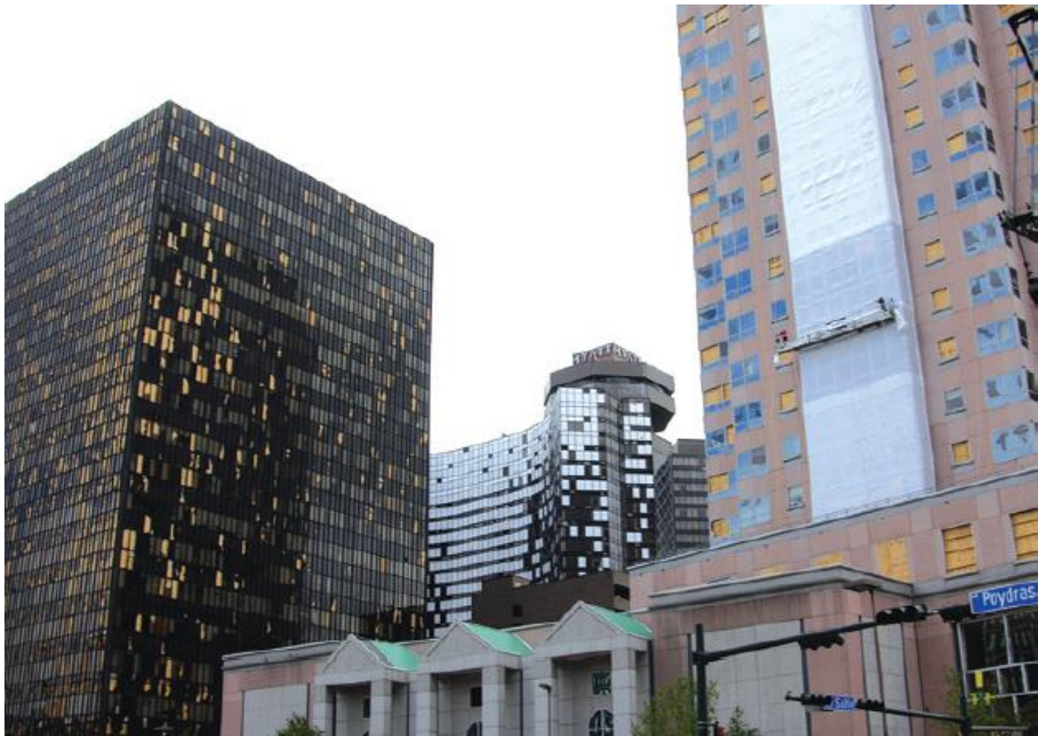
Figure 22 Windborne Debris from Roof Top Aggregate Damaged Glazing Source FEMA-549 p107
