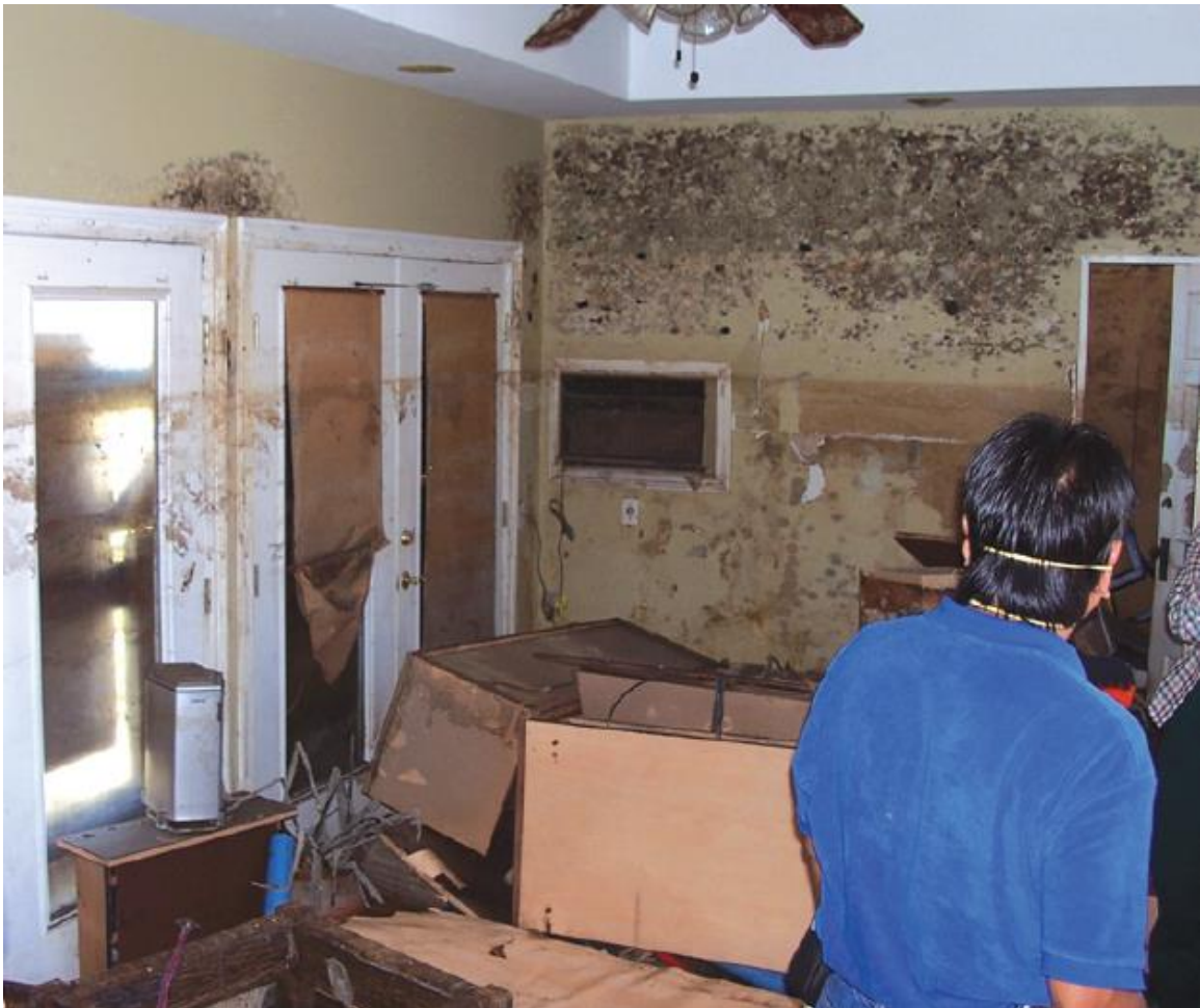
Figure 18 Mold Damage After Flood Waters Receded Source FEMA-549 p95
