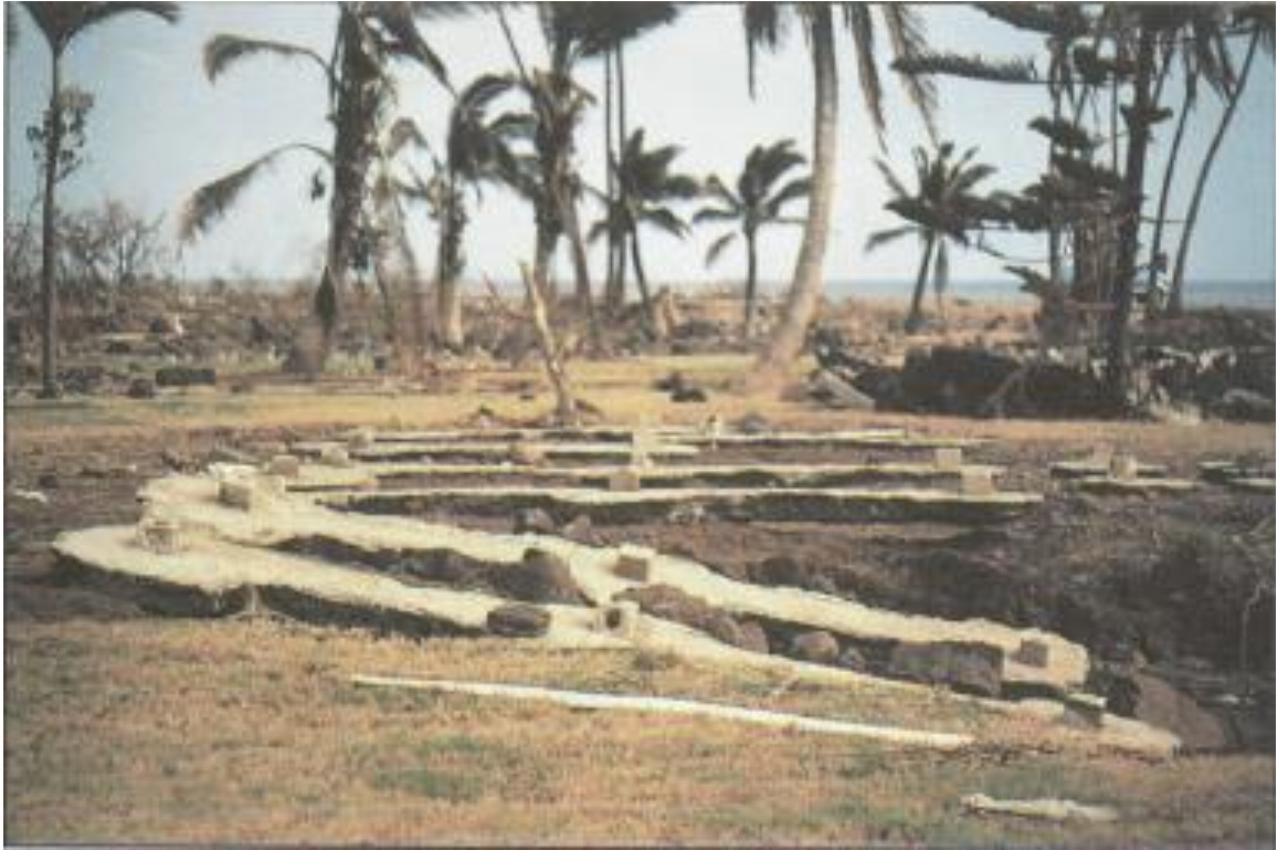
Figure 11 Poipu Beach Improper Foundation Source FIA-23 p40
