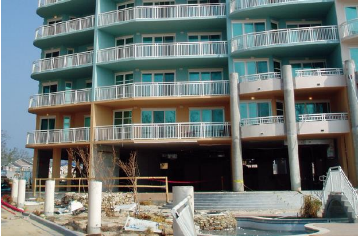
Figure 20 First Level Destroyed from Wave Action Source FEMA-549 p101
