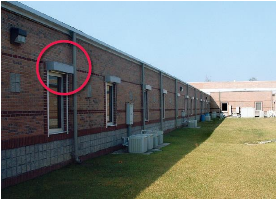
Figure 23 Storm Shutters Protected Glazing Source FEMA-549 p381
