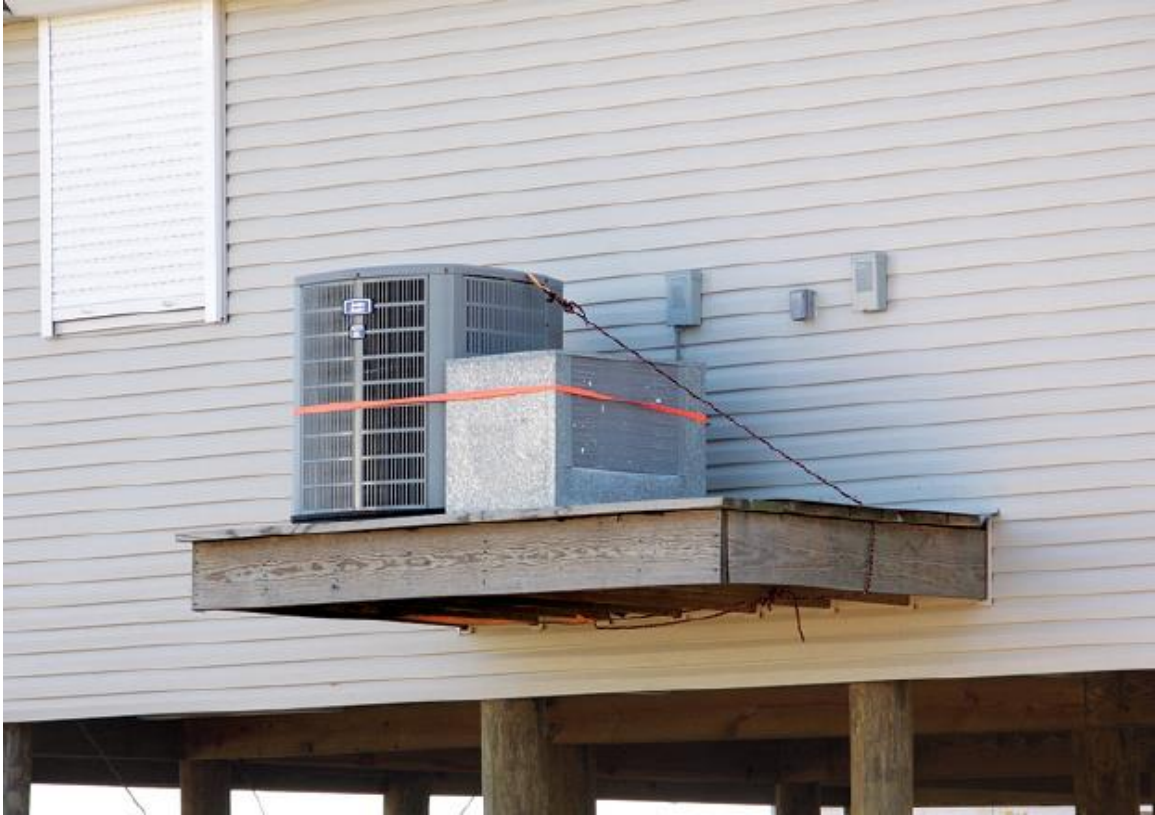
Figure 25 Elevated HVAC and Power Systems Protected from Flood Waters Source FEMA-549 p384
