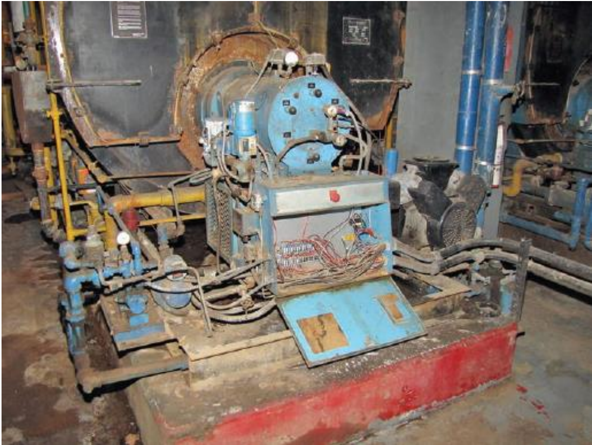
Figure 28 Boiler in Basement Damaged Due to Flooding Source FEMA P-942 p4-22
