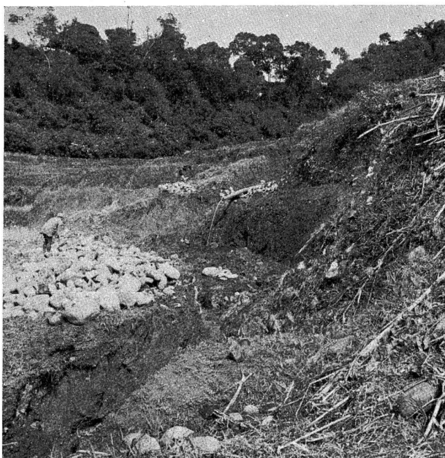
Plate II Ifugao rice pond terrace under construction.
