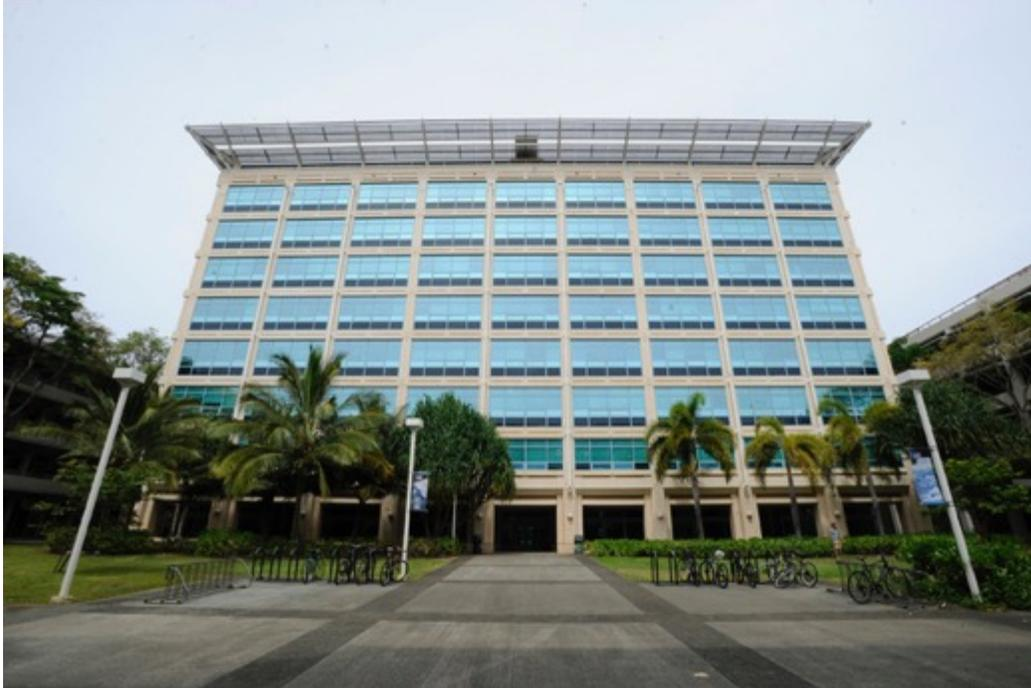
**Image 3** The Pacific Ocean Science and Technology (POST) building on UH Manoa Campus. It is poured reinforced concrete with reflective film on the windows. The external UBLOX GNSS receiver did not always obtain a position while it was installed in the North, South, and East facing windows. It was never able to obtain a position while it was installed in a West Facing window.
