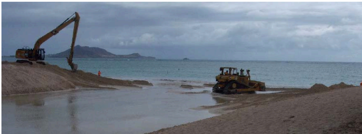
Figure 6: To establish connection between Kailua Bay and Kaelepulu Estuary, heavy equipment is needed to move the naturally accreting sand. Photo Credit Bob Bourke, 2016
