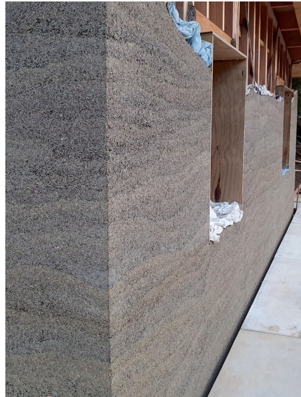
Figure 6.4 Hemp concrete infill exterior wall. Image Source: Alex Sparrow, The Hempcrete Book.
