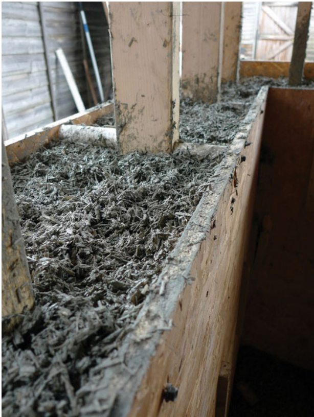
Figure 6.3 Hemp concrete infill form. Image Source: Alex Sparrow, The Hempcrete Book.
