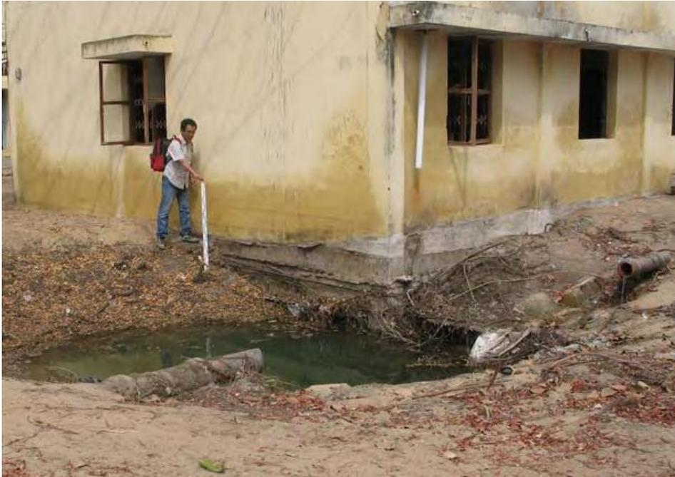
Figure 68: Failure of a sewage line due to scour
