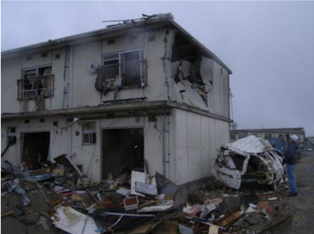
Figure 64: Debris impact damage in buildings, Natori
