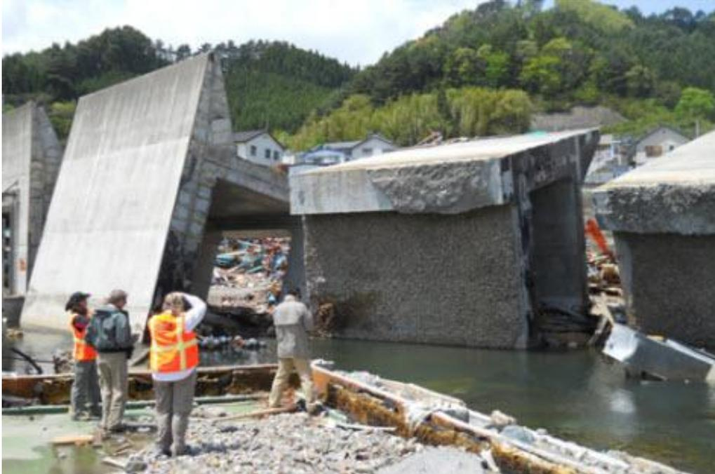
Figure 66: Overturned tsunami wall, Kohirahama.
