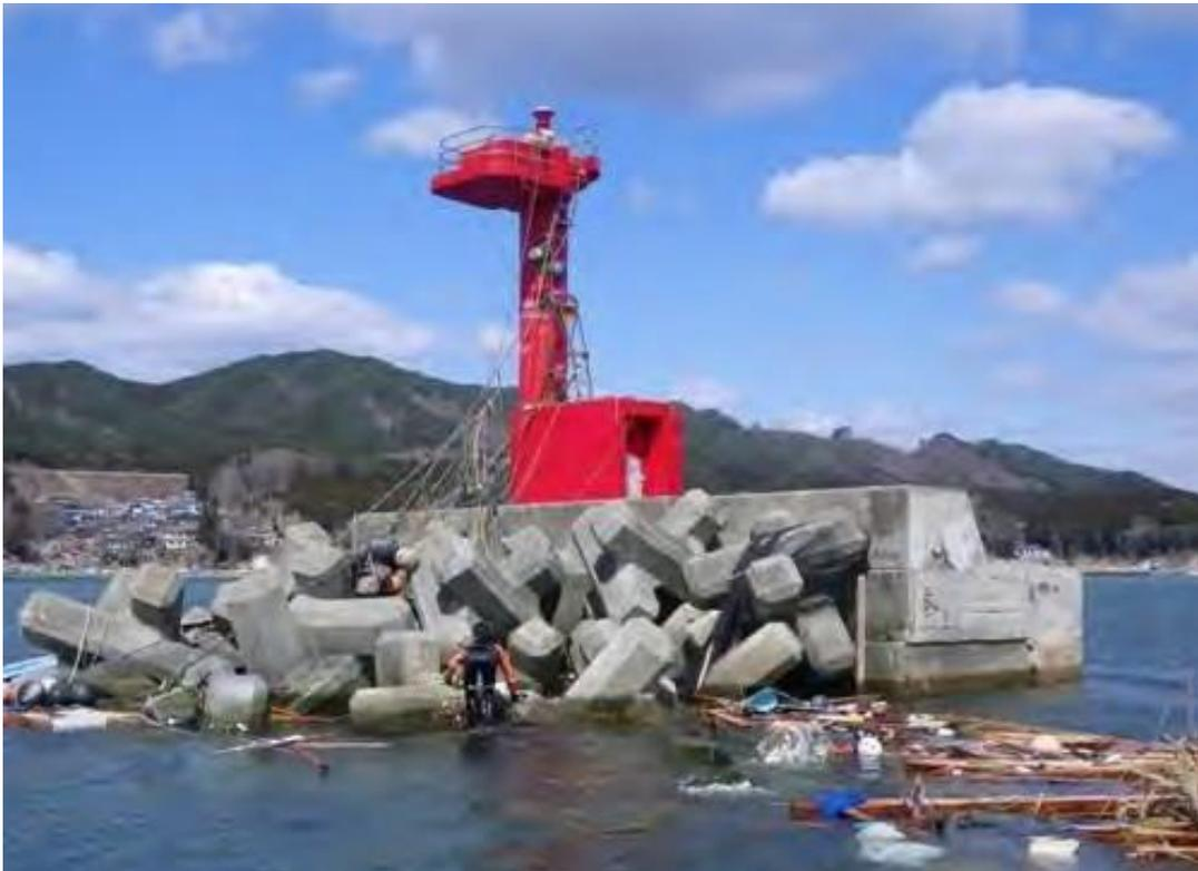
Figure 63: Collapsed Funakoshi East Breakwater
