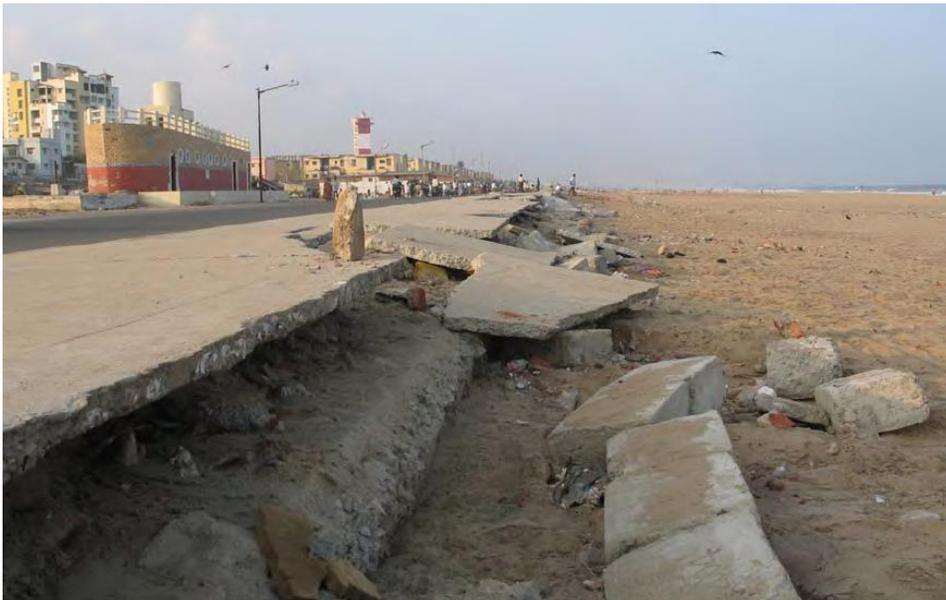
Figure 69: Collapsed concrete waterfront due to scour, Chennai
