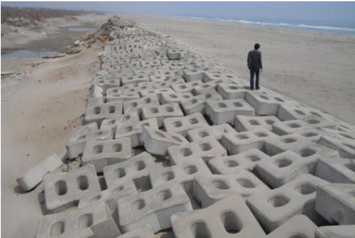
Figure 62: Failed section of Coastal Revetment
