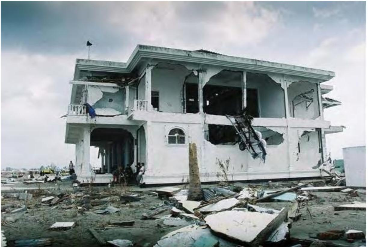
Figure 70: Concrete building after tsunami flood, Banda Aceh
