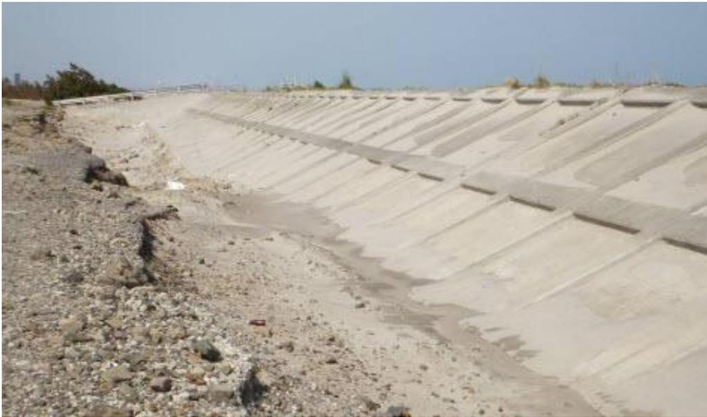
Figure 65: Scour in Sendai's Seawall
