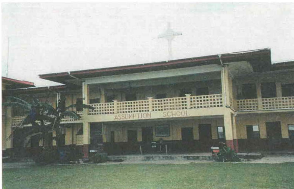
Figure 22. Assumption Convent, above the Elementary School.
