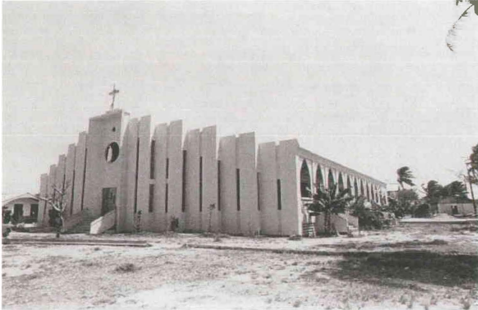
Figure 56. Assumption 1960s. TTPI photo archive #2783-11.
