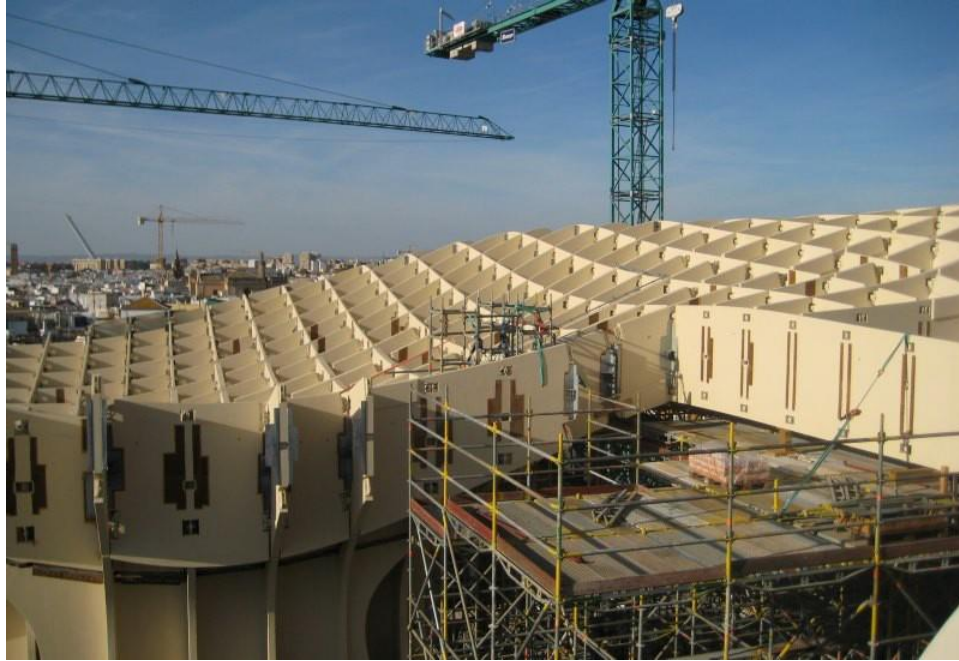
Figure 2.24: Construction of Metropol Parasol
