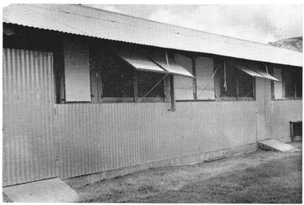
FIGURE 13. Muslin on movable frames on brooder house. (Courtesy Hawaii Agricultural Experiment Station.)
