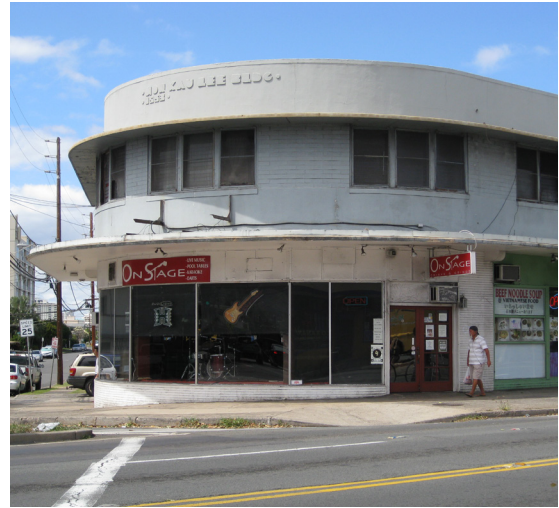
Overhang at On Stage building
