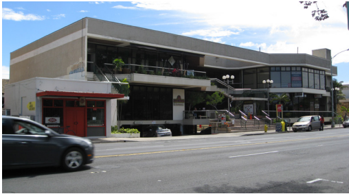
Under ground parking structure
