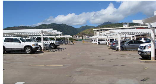
Parking on rooftop at Safeway
