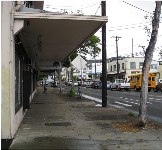
Overhang shading sidewalk on Kapahulu Avenue
