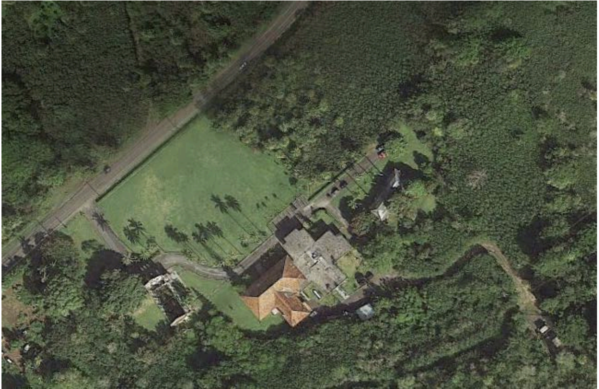
Figure 19.1: Aerial photograph of the property showing existing building structures.
