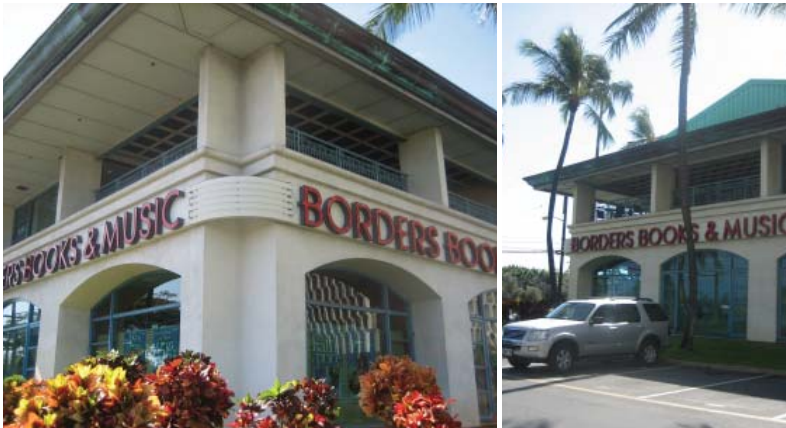
FIGURE 56 Borders second floor outdoor balcony Sanpei 02.15.08
