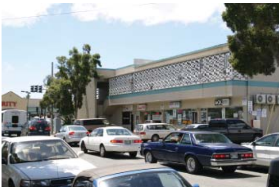
Selected Site Halekauwila Street
