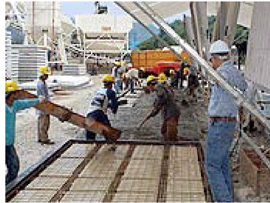
Figure 38 and 39 – Pouring waffle-crete forms (Left), Erecting the Wall Panel (Right). Source: Waffle-Crete International Inc.
