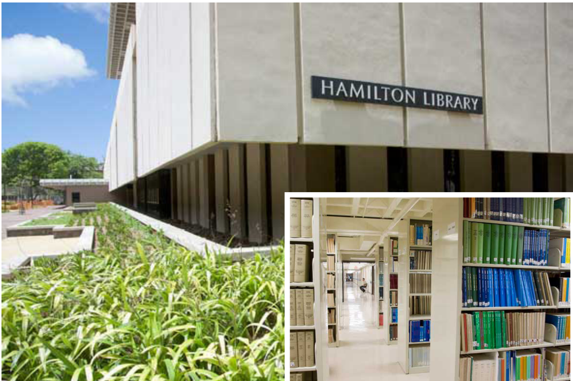
[Figure 43 & 44: Hamilton Library newly renovated exterior and interior basement level.]
