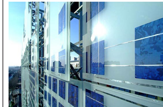
[Fig. 86 & 87: Exterior glass curtain wall treatment example and solar powered glass curtain wall system.]
