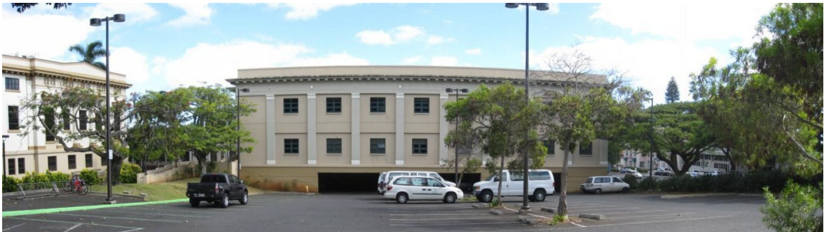
[Figure 64: North façade from parking lot.]
