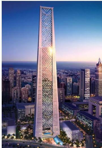
Figure 7.3 – DIFC Lighthouse Tower. 165
