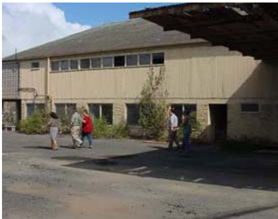
Figure 5.55 – Sand Island Reuse Facility: A Non-Profit Agency. 141
