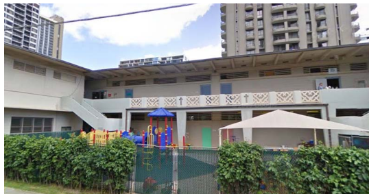
Figure 4.14: Exterior of the Waikiki Community Center with Enclosed Spaces
