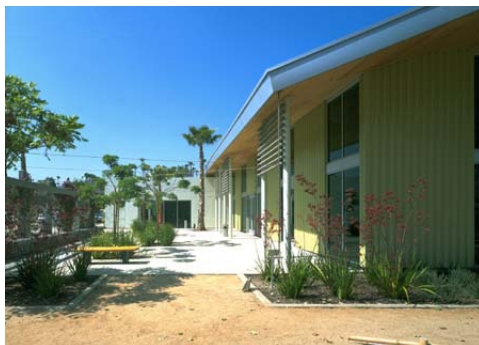
Figure 4.2: Plummer Park Community Center Exterior
