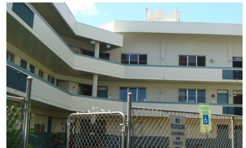
Figure 4.21: Enclosed Spaces and Hallways of the Mo'ili'ili Community Center
