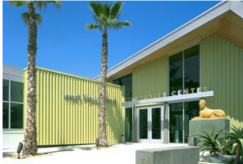
Figure 4.1: Plummer Park Community Center Entrance
