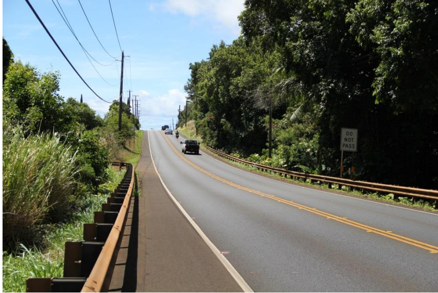
Figure 221: West Bound on Kaumualii Highway. Fronting the site there are no sidewalks or crosswalks. The white painted marking on the road separates pedestrian right of way from vehicular right of way. Photo by Author
