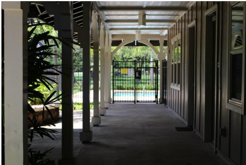
Figure 241: View of the community pool. The heated pool is utilized by residents and their guests. The pool is located adjacent to the exercise room. One resident commented because of her problem with her incontinence, she does not use the pool.
