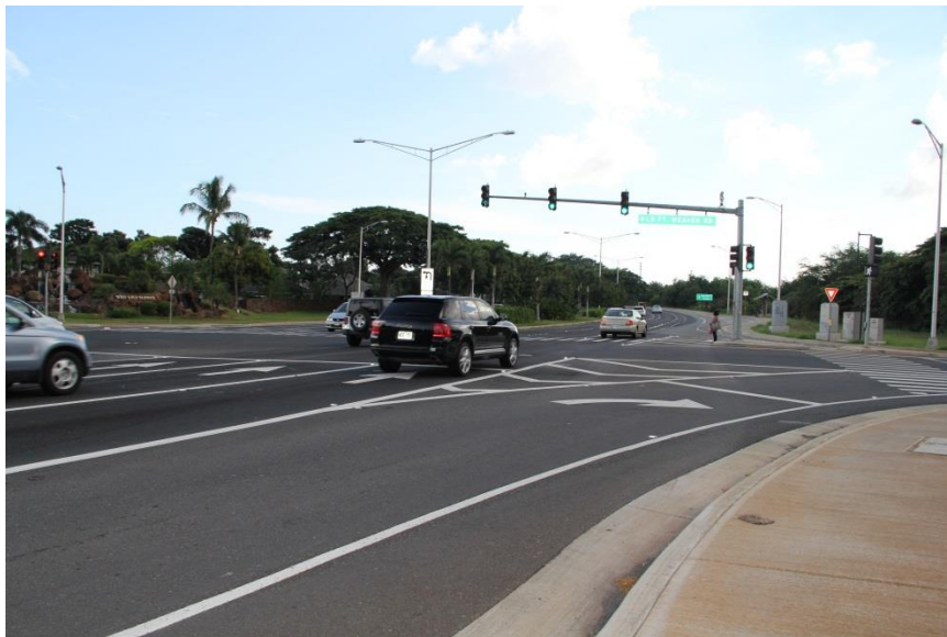
Figure 211: Old Fort Weaver Road intersects with Fort Weaver Road, the main vehicular artery into Ewa and the surrounding areas. Although this busy eight lane intersection is equipped with curb cuts, crosswalks, and traffic lights, it may be a challenge for the segment of the elderly population with mobility issues. Photo by Author
