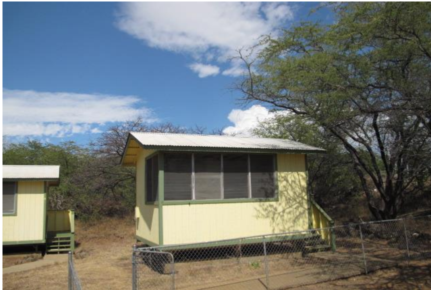
Figure 132: Typical Single Unit Photo by Author
