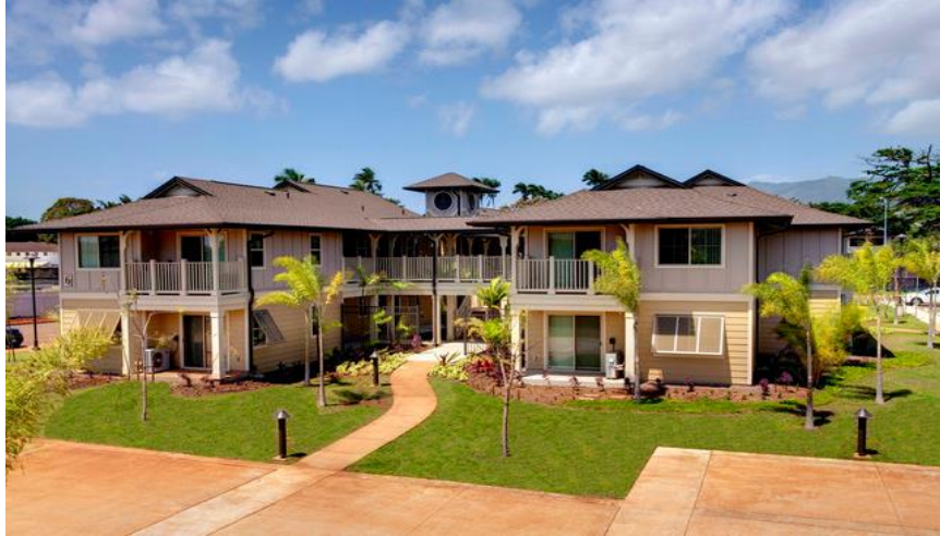
Figure 71: Typical Cluster, Exterior View 114
