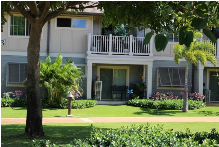
Figure 253: Wheelchair accessible apartment units are located on the first floor. As people age, their visual depth perception changes, which can make it difficult to judge distances. Concerns for wheelchair bound residents have been expressed as the patio does not have physical cues to aid these residents from falling off their patio.
