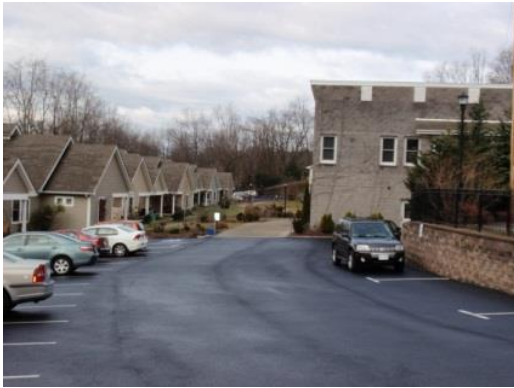
Figure 35: View of the east parking lot
