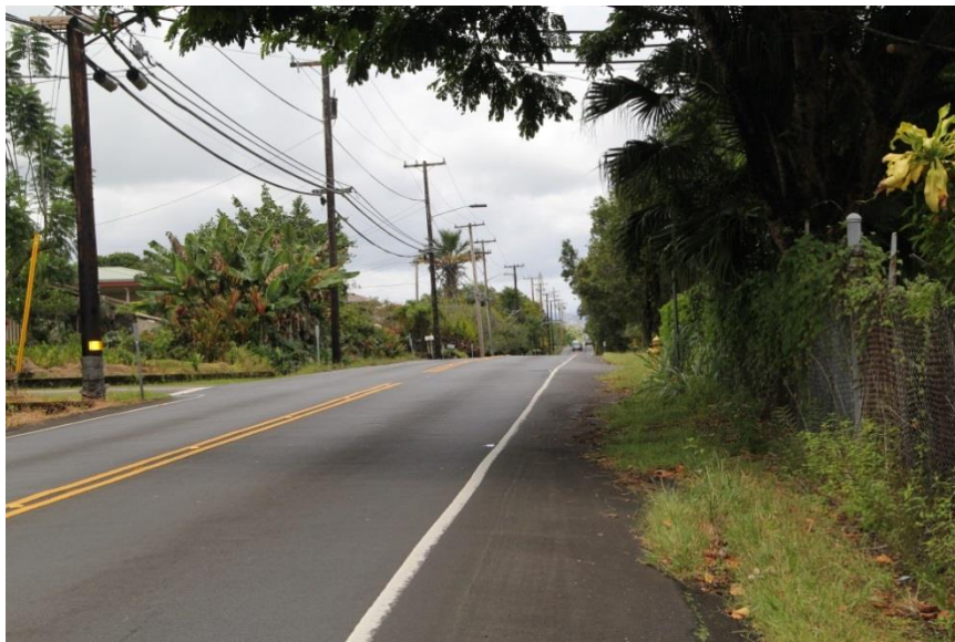
Figure 231: West bound on Haihai Street. Haihai Street is a 2 lane road that runs directly in front of the site. The pedestrian right of way has no sidewalk and is separated only by the white painted marking. The street is on an incline. Photo by Author
