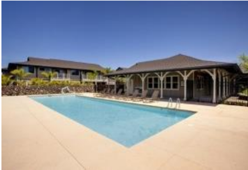
Figure 237: Many of the survey participants noted that the community center, which houses a fitness center, swimming pool, hair salon, learning center, dining room, and conference room is an area that fosters community at the facility. 358
