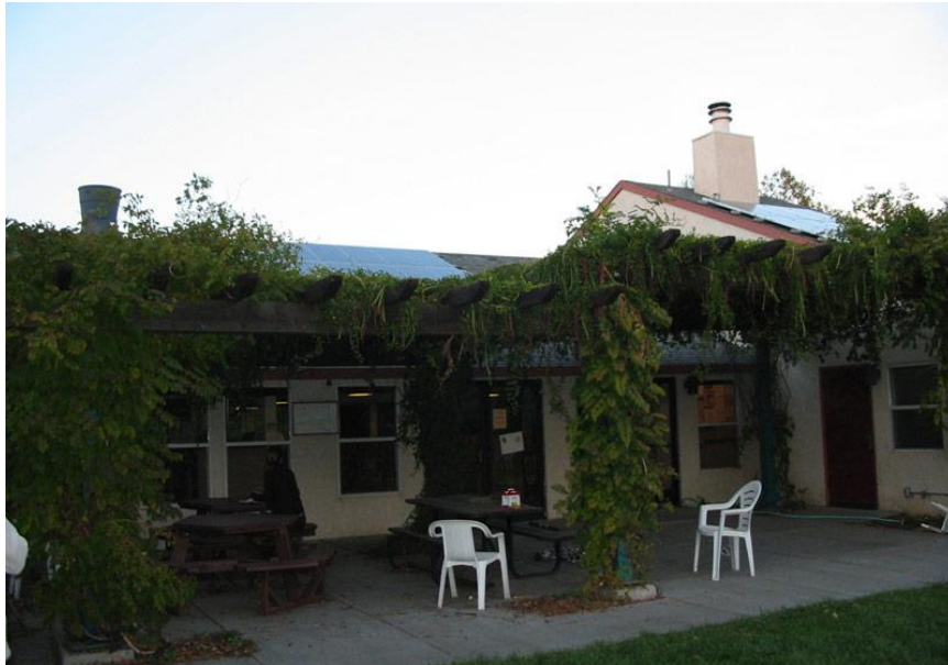
Figure 14: Muir Commons Cohousing Community, located in Davis California, is the first intergenerational cohousing community to be built in the United States. The community, completed in 1991, is built on 2.9 acres and consist of 26 units. Architects Charles Durrett and Kathryn McCamant, who built the community, did extensive research on cohousing in Denmark. 36
