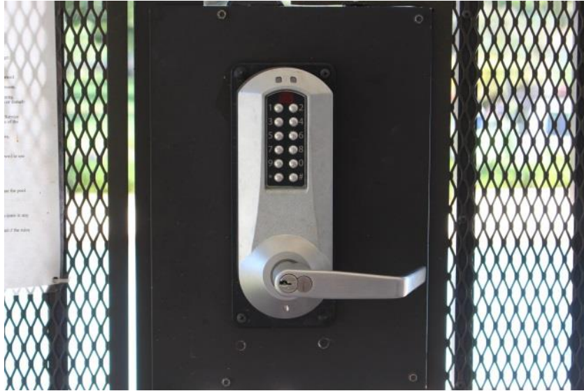
Figure 245: Coded key lock shown above is found on all gates at all entrance points into the residential building units. Some residents feel a false sense of security as strangers are inadvertently allowed into the interior courtyard areas of the building.
