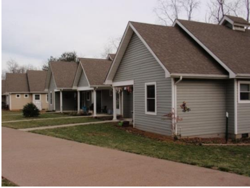
Figure 159: Shown here is a typical single story attached residential units.
