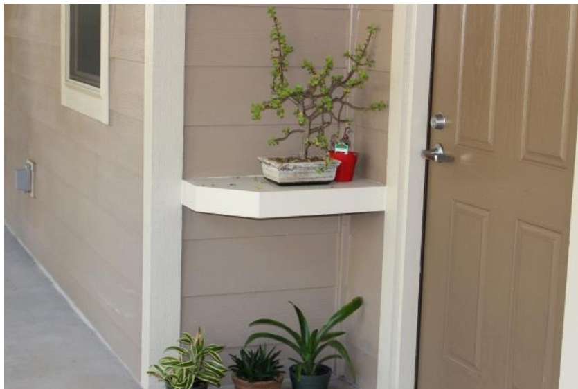
Figure 246: Seniors have found that the two features in this image have made their life easier. 1) The shelf serves as a resting place for bags, groceries and other items before bringing it into the home. 2) The entrance door locks are keyed to prevent inadvertent lockouts by residents.
