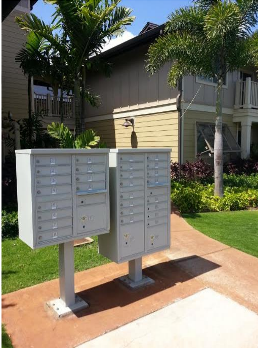
Figure 239: There are several community mail centers located at throughout the property. The one shown here is located at the back of the property. 359
