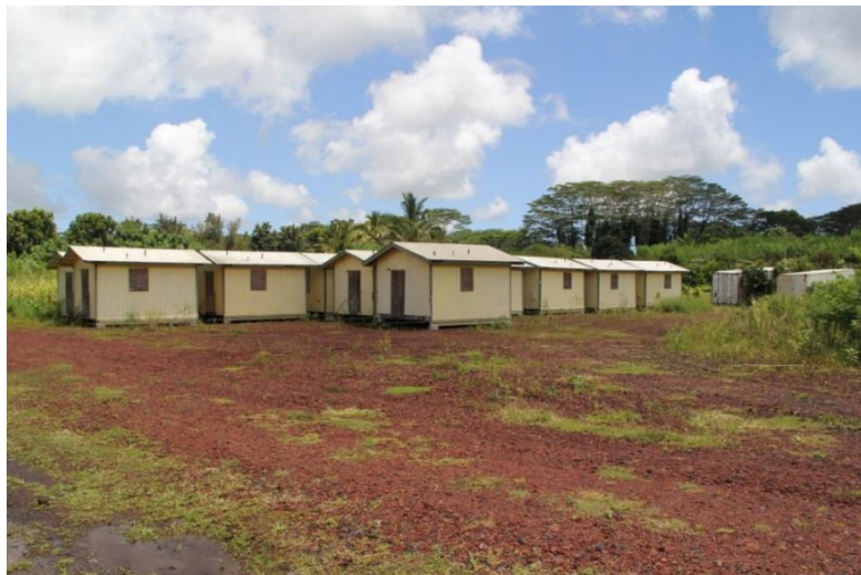
Figure 141: The units were moved from Kawaihae to Pahoia and are staged on site as the project awaits permitting.
