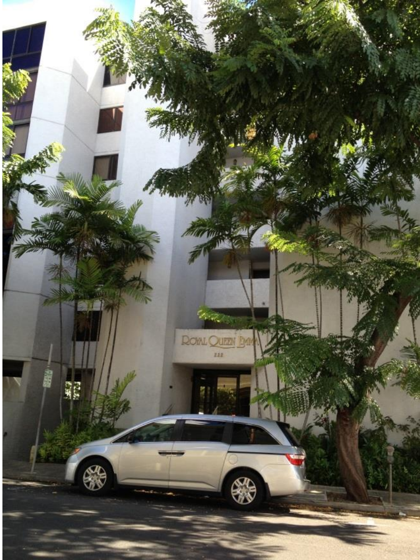
Figure 195: The Royal Queen Emma condominium is located adjacent to the site. This 7-story mixed-use residential and business complex has 24 units. Photo by Author
