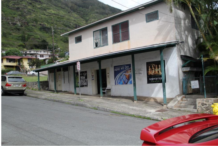
Figure 180: New Valley Store, a mini convenient store, located at 2119 Kauhana Street, is 0.06 miles north from the site. Photo by Author
