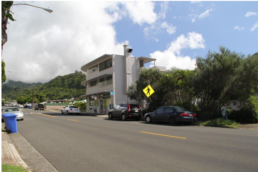
Figure 179: At the corner, adjacent to the project site, is a low rise apartment complex with a laundry center located on street level. Pedestrian crossing signs and curb cuts are found at this intersection of Kauhana Street and Palolo Avenue. Photo by Author
