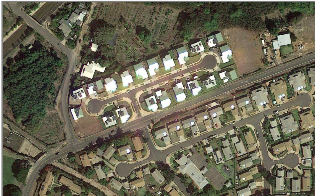
Figure 9: Kaupuni Village, is located in Waianae on the island of Oahu. The Department of Hawaiian Home Land's Net-Zero Energy, LEED Platinum project consist of nineteen single-family homes. The community is the nation's first low-income affordable housing project to achieve this certification. 13
