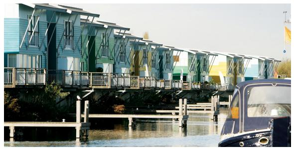
Amphibious houses on the Maas River with cellars that act as floatation devices. When water level rises, the building rises with it, sliding up two steel posts. (Courtesy of Dura Vermeer)
