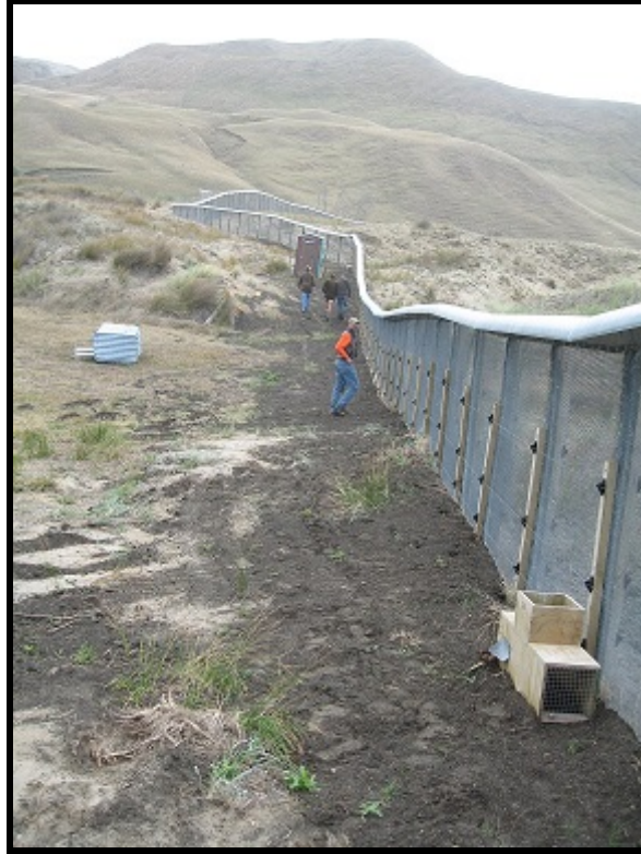
Figure 6. Small mammal pest proof fencing in New Zealand showing the basic structure and its use to enclose very large areas.
