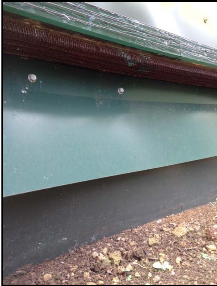
Figure 9. Angle barrier installed directly below cut mesh
