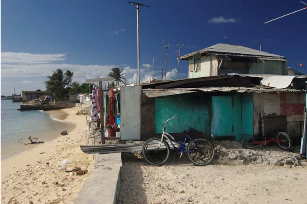
Photo 2. Plywood housing along the lagoon at Ebeye. Photo by Greg Dvorak.
