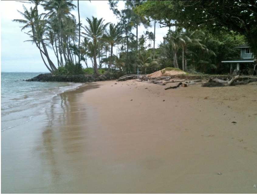
Figure 2.6. Flanking erosion at Makalii Point (photo location shown in Figure 2.5; photo date, March 15, 2011). Note that beach has been lost fronting the armoring in the background. Accelerated erosion of the beach in the foreground is attributed to flanking effects of the armoring in the background. Though the shoreline is receding, a beach remains along the foreground area in the absence of coastal armoring.
