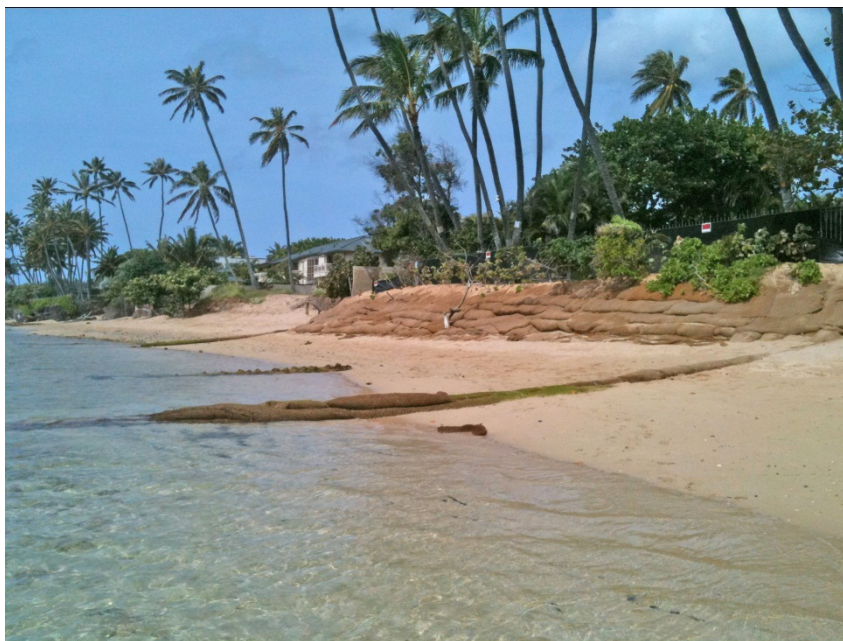
Figure 2.10. Flanking erosion and temporary armoring (sand bags), west Kahala Beach (location shown in Figure 2.8; photo date, March 21, 2011).
