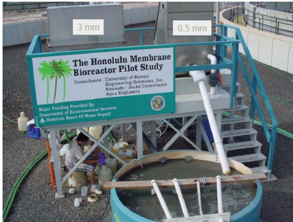
Figure 2.2 Bench-scale and pilot MBRs headworks and feed tank at Honouliuli WWTP
