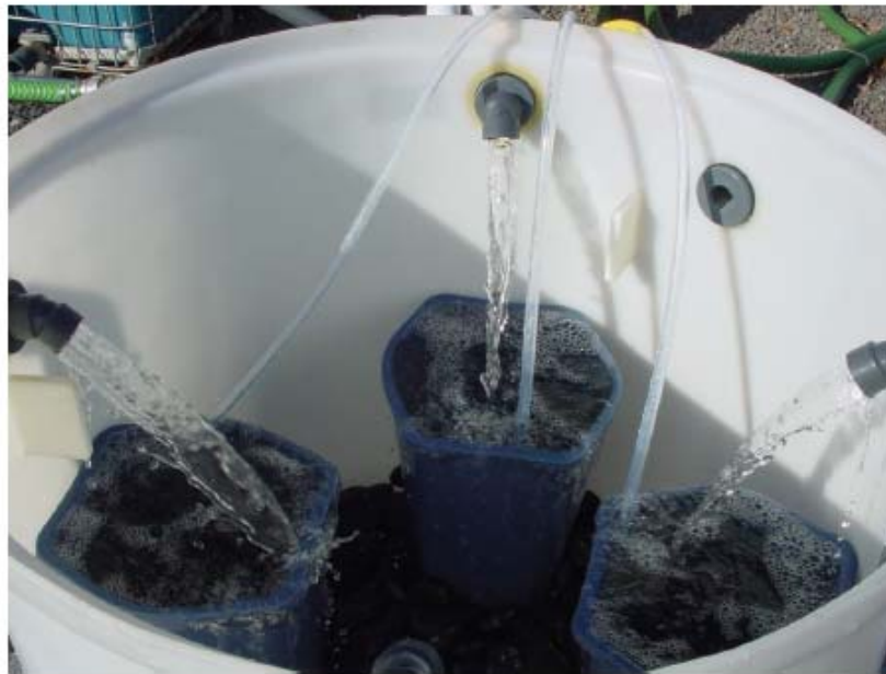
Figure 2.4 Pilot MBRs common effluent tank at Honouliuli WWTP
