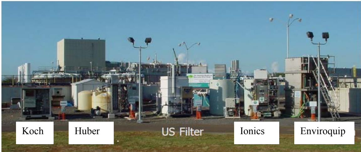
Figure 2.3 Pilot MBRs at Honouliuli WWTP
