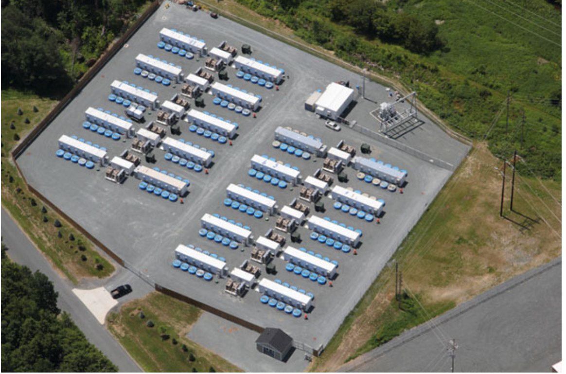
Figure 1.7. Beacon Power's 20MW flywheel energy storage facility in Stephantown, NY [41]
