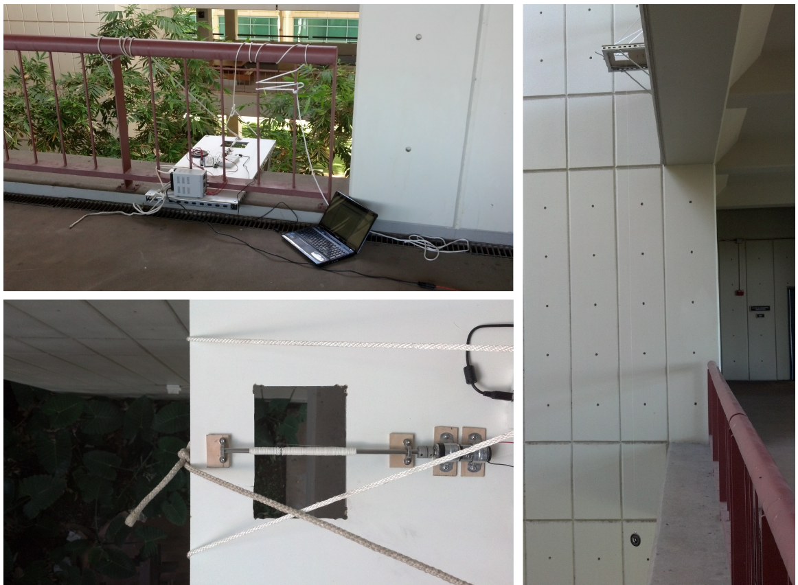
Figure 5.3. The drop test setup in the Holmes Hall Atrium.
