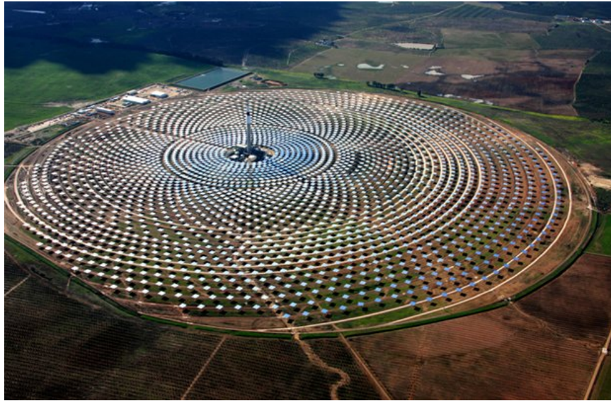
Figure 1.8. The Gemasolar CSP plant which utilizes thermal energy storage to increase availability of electricity production [47]
