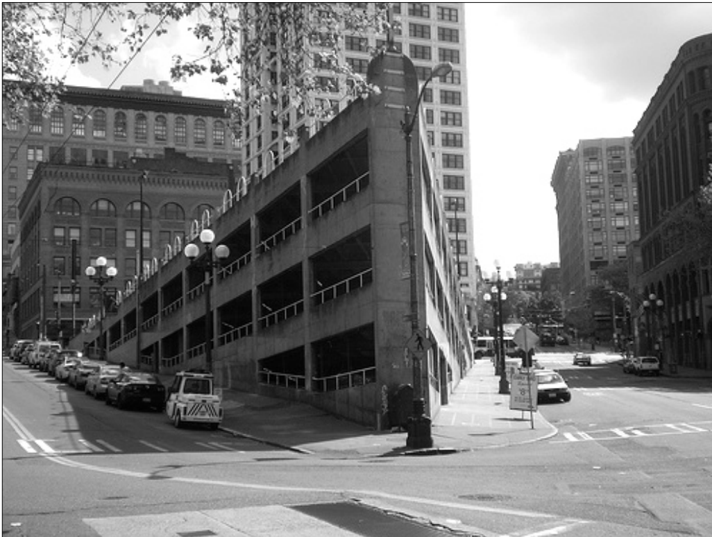
Figure 37. "Sinking Ship" parking garage that replaced Hotel Seattle after its demolition in 1962. (Image courtesy of WSDOT)
