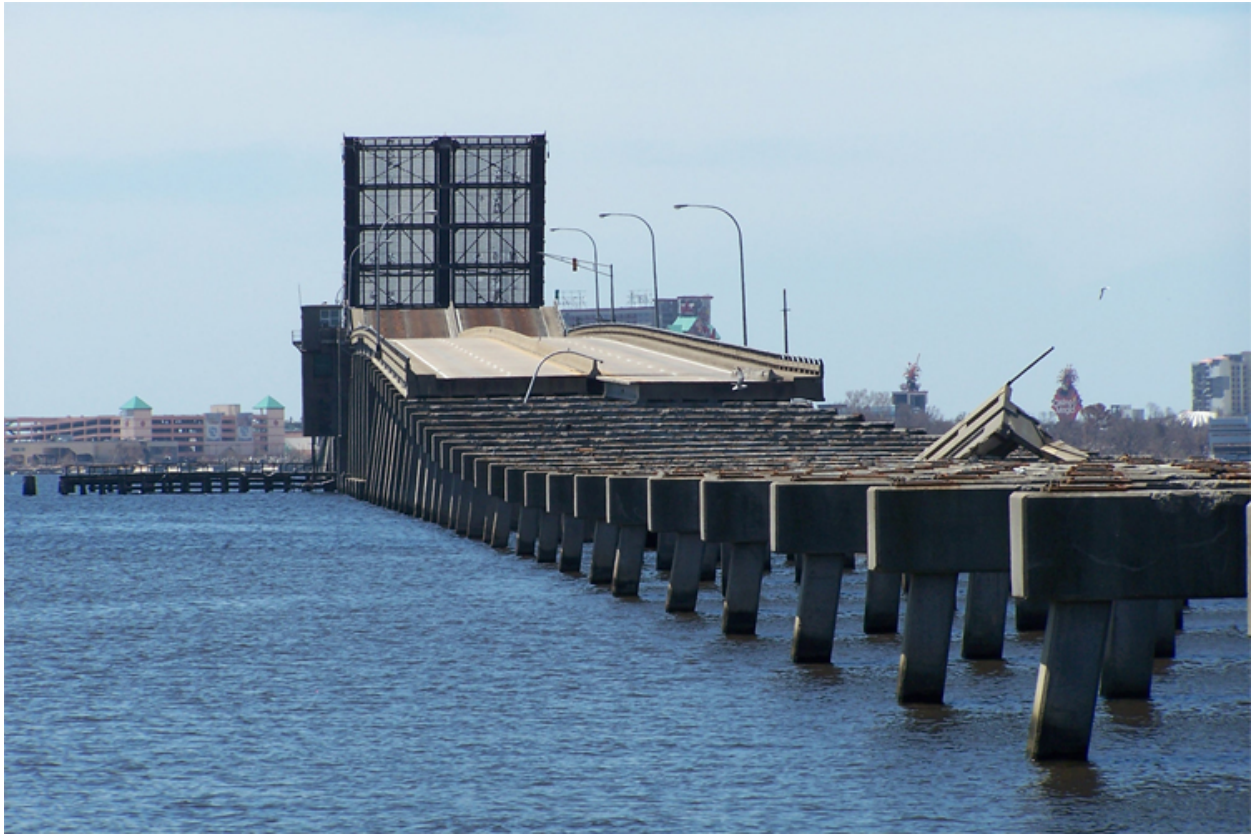
Figure 1.1: The US 90 Biloxi Bay Bridge was damaged during the 2005 Hurricane Katrina. The bridge spans were lifted off piles except at the higher elevations near a navigation channel, which received much less damage. Photo: J. O'Connor (for MCEER).
