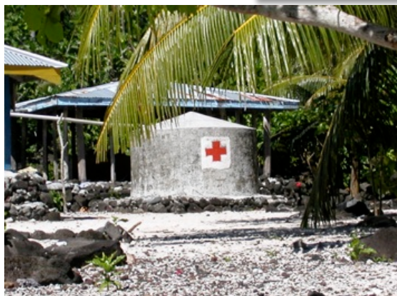
Water tank donated by the aid from Switzerland.
