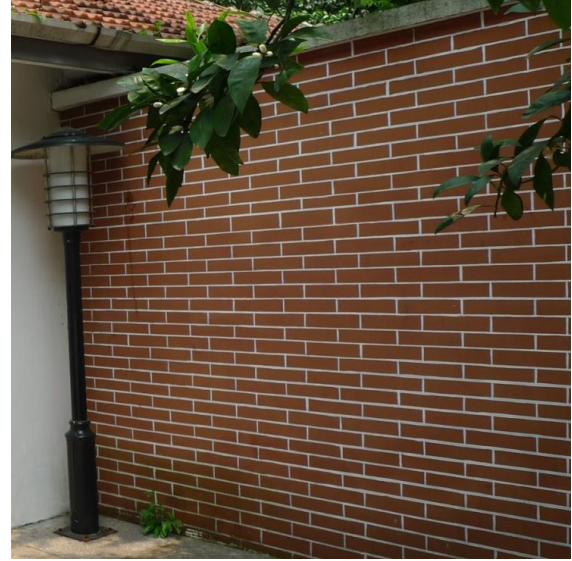
Figure 2-24: The Brick Wall with White Stucco Coating and painting.
