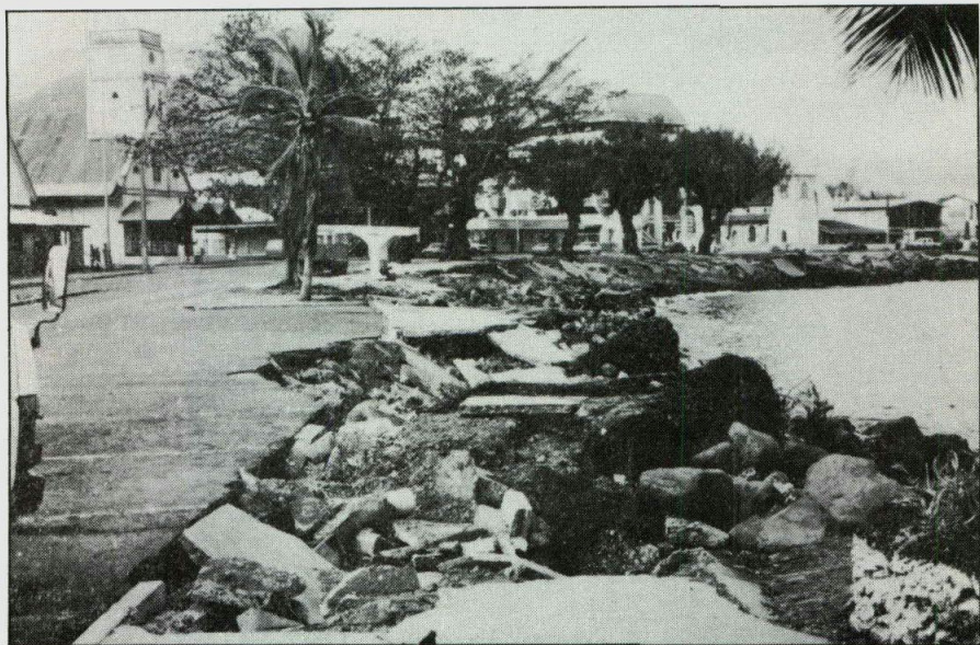
Plate 3. Damage caused by storm waves to Apia waterfront in Western Samoa during Tropical Cyclone Ofa in February 1990. Photo by author.
