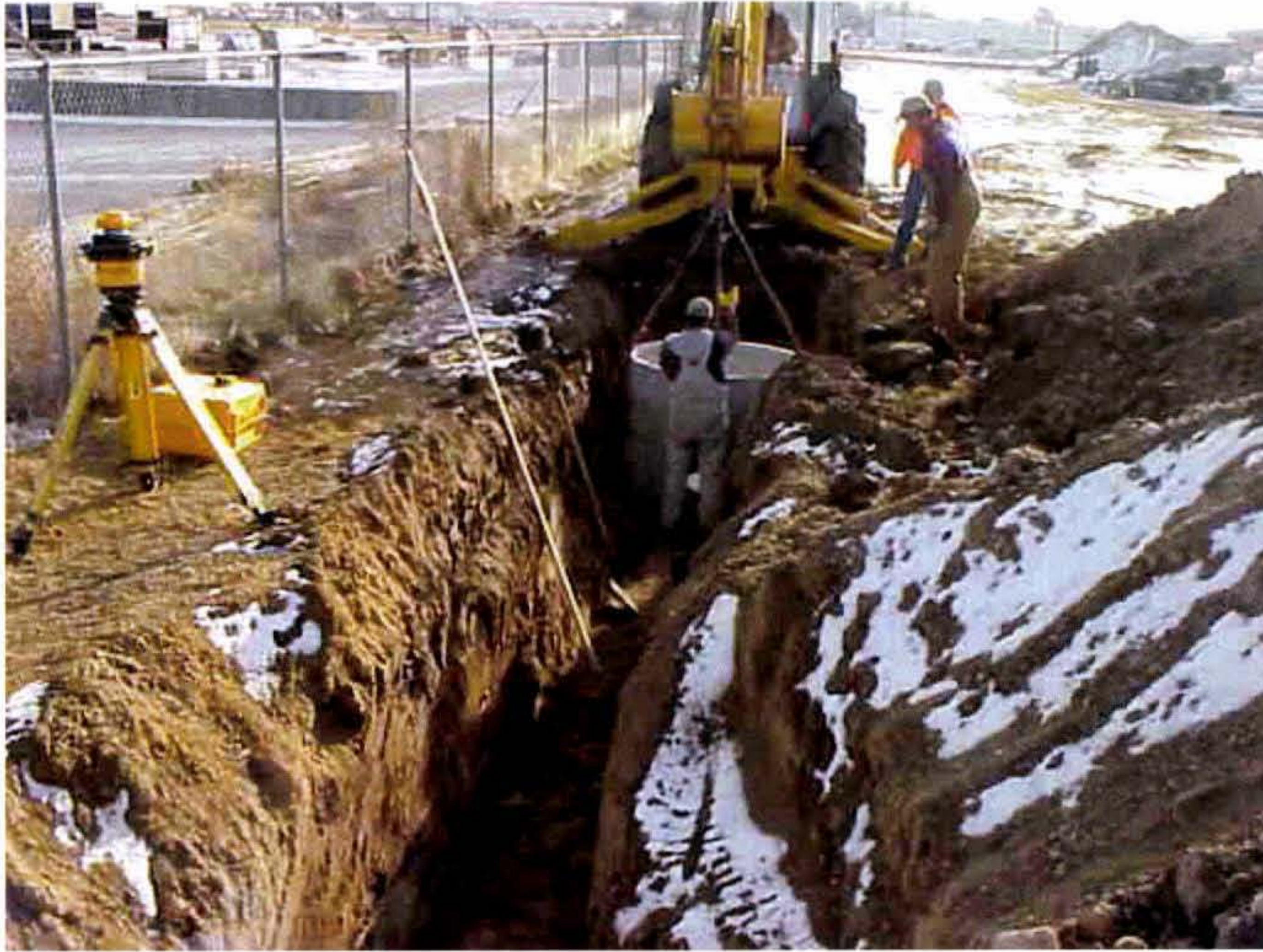
Trenching for storm drain at Cloverdale maintenance yard.
