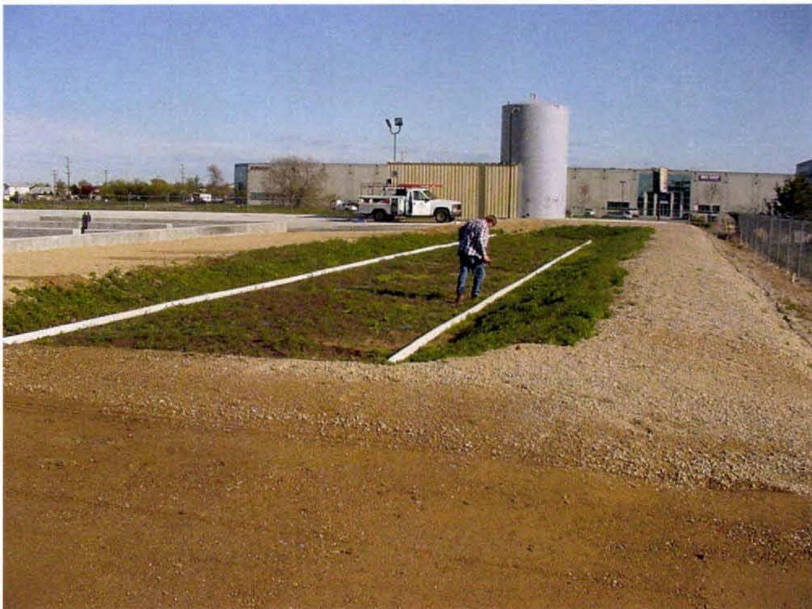
Completed sand filter
