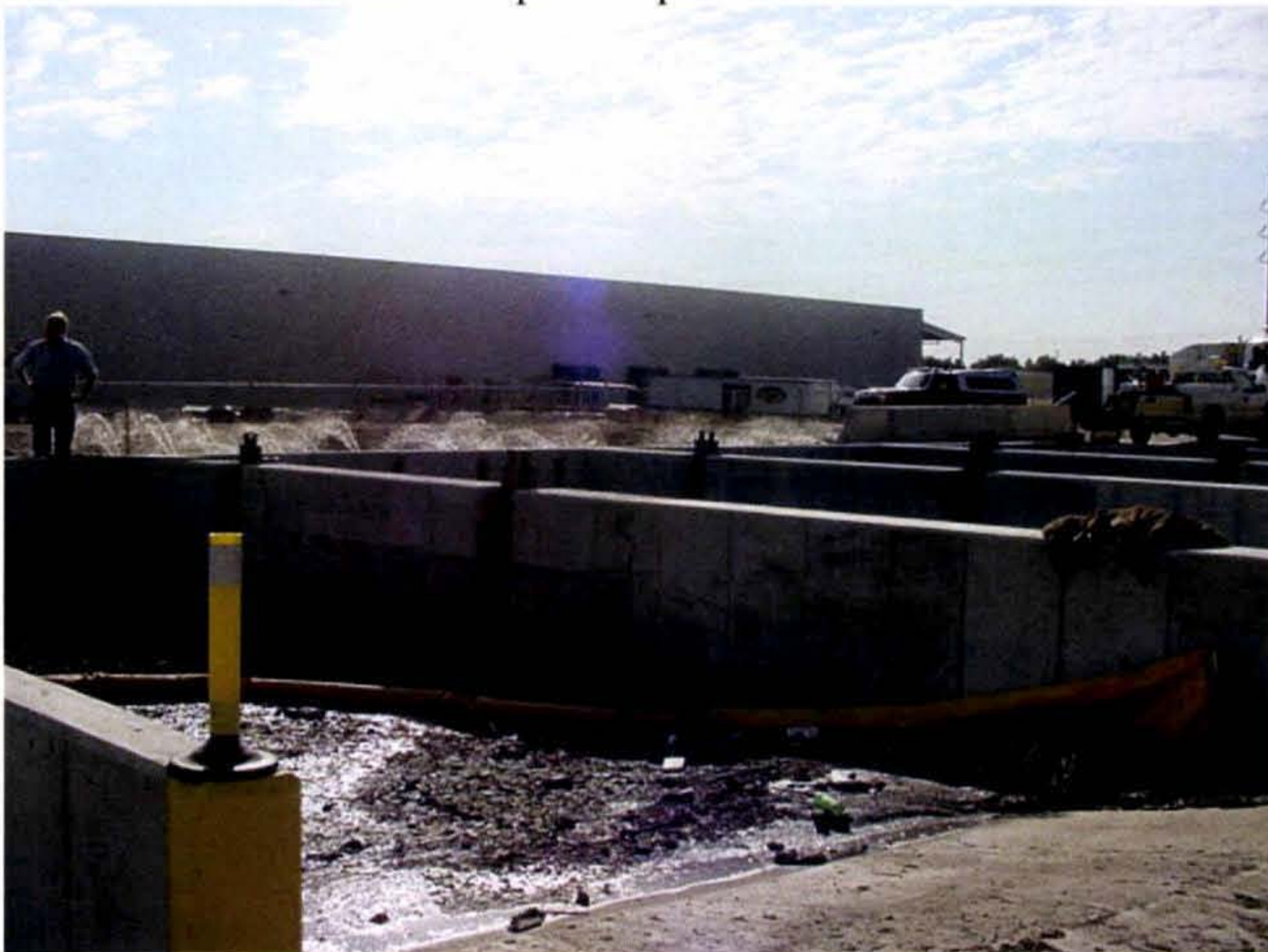
Sediment basin in operation
