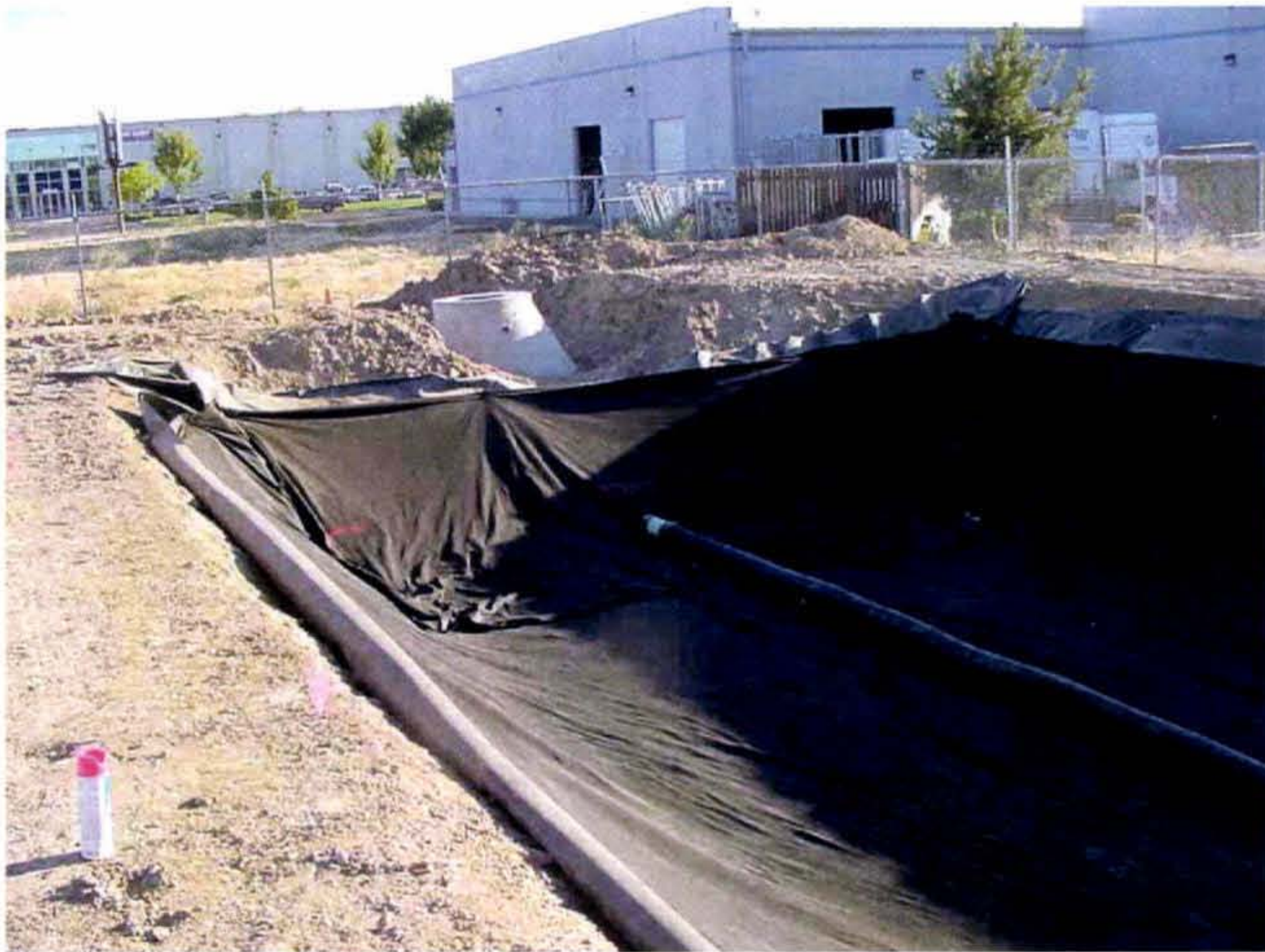
Sand filter construction
