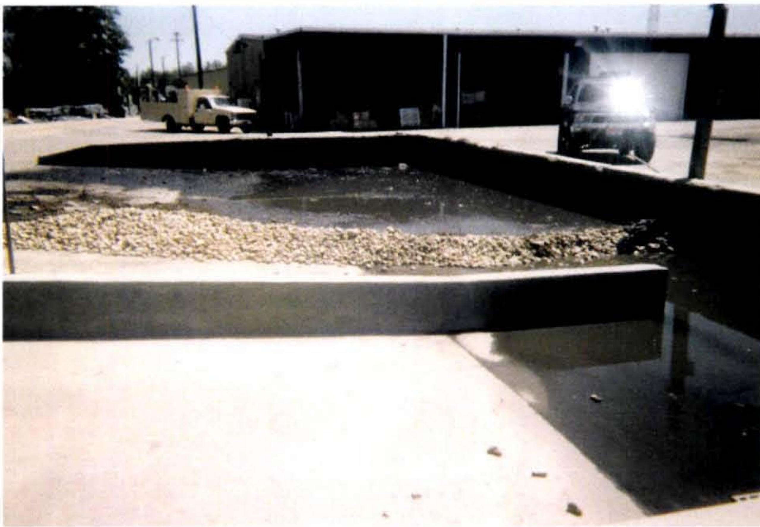
Figure 3.5 - Decant Basin at ACHD's Adams Street Facility (photo taken facing East)
