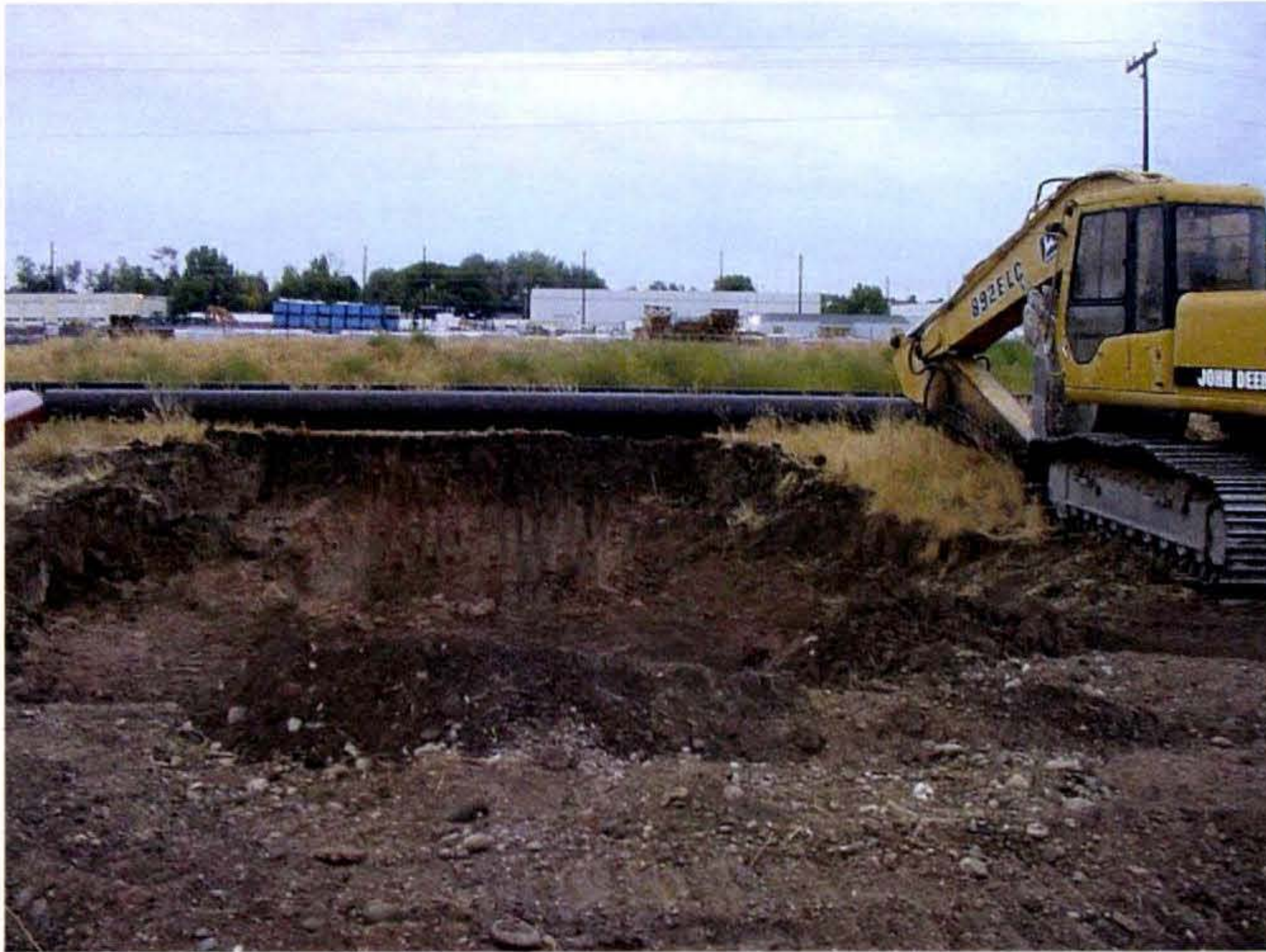
Outfall construction under Union Pacific Railroad tracks
