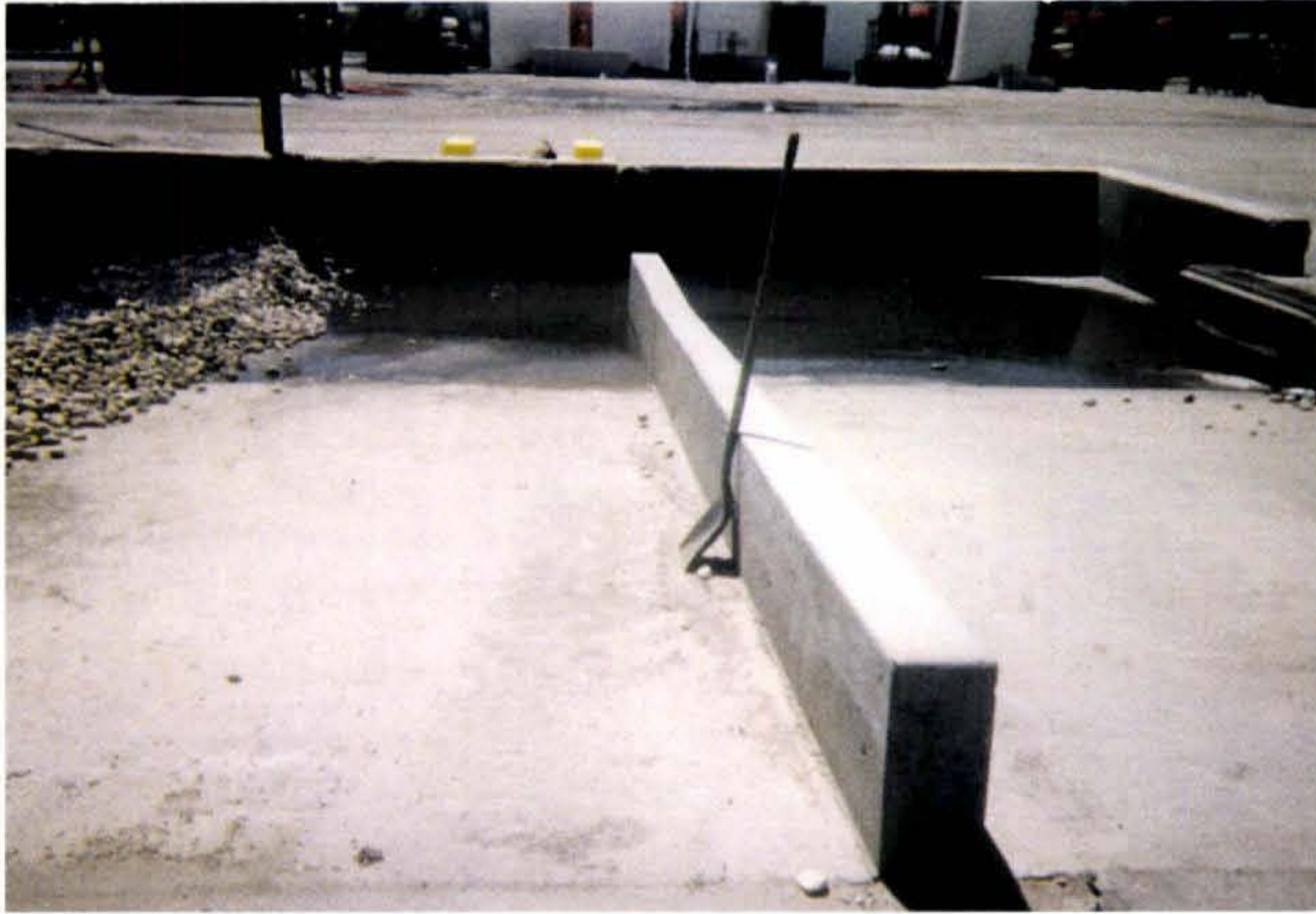
Figure 3.4 - Decant Basin at ACHD's Adams Street Facility (photo taken facing South)
