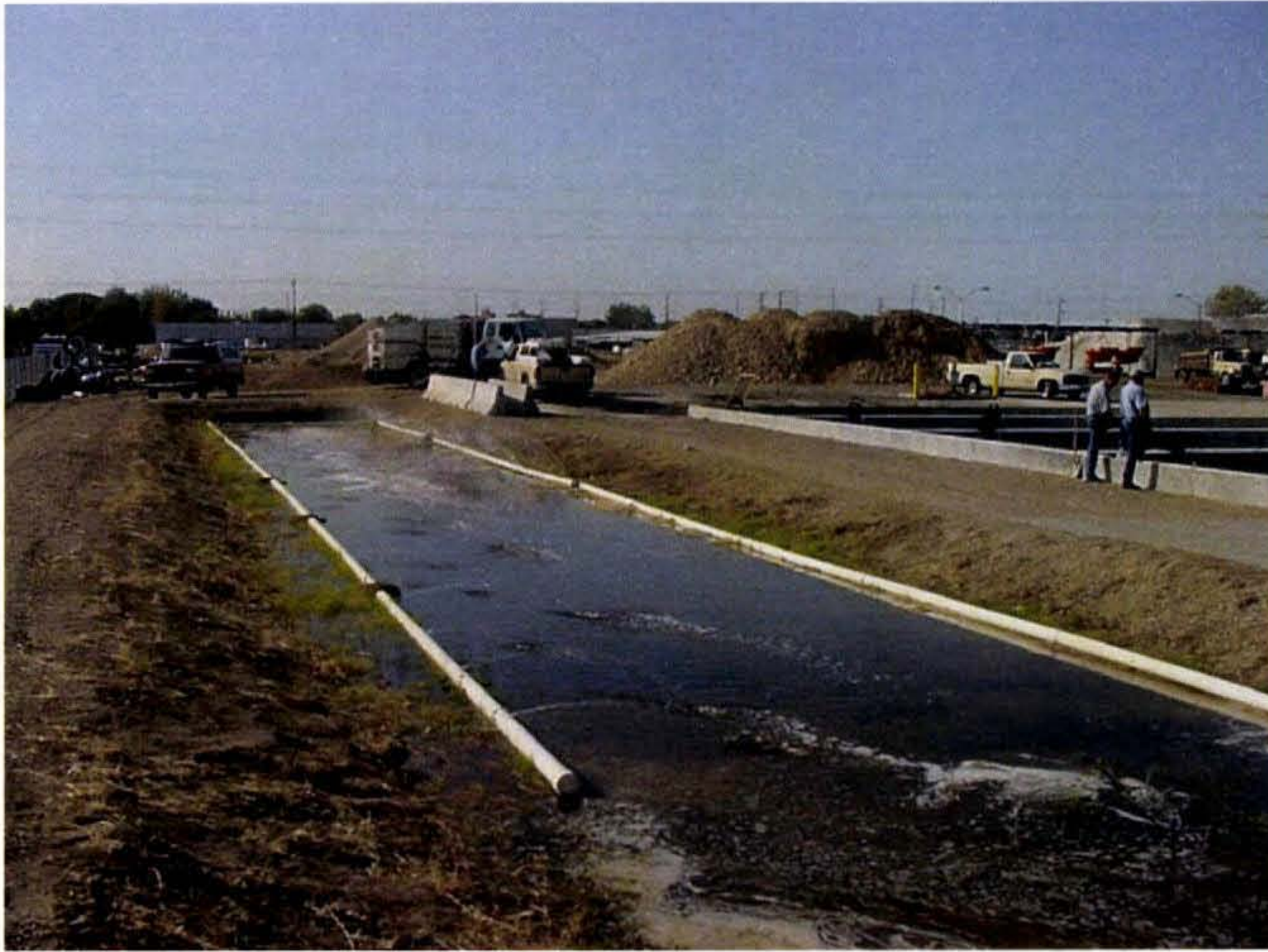
Sand filter in operation
