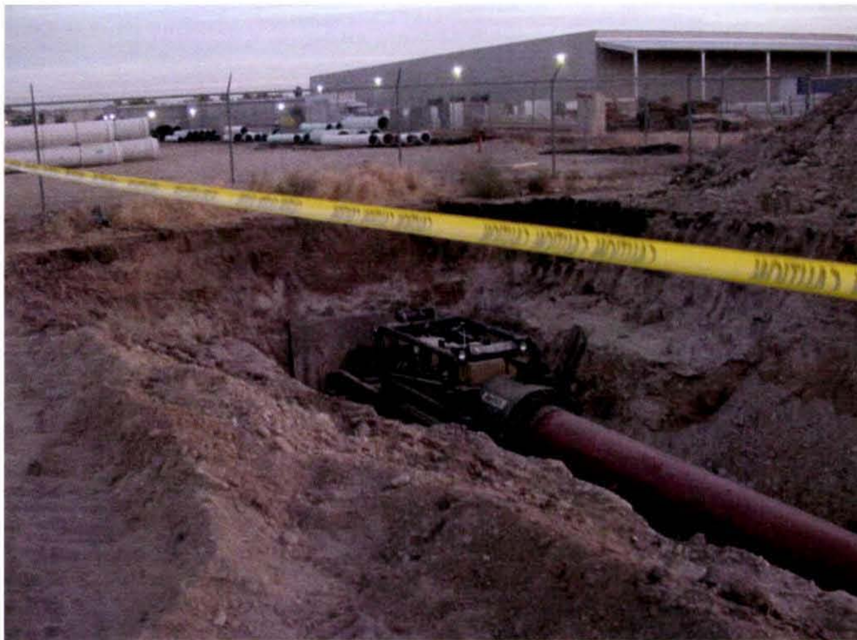
Outfall construction under Union Pacific Railroad tracks
