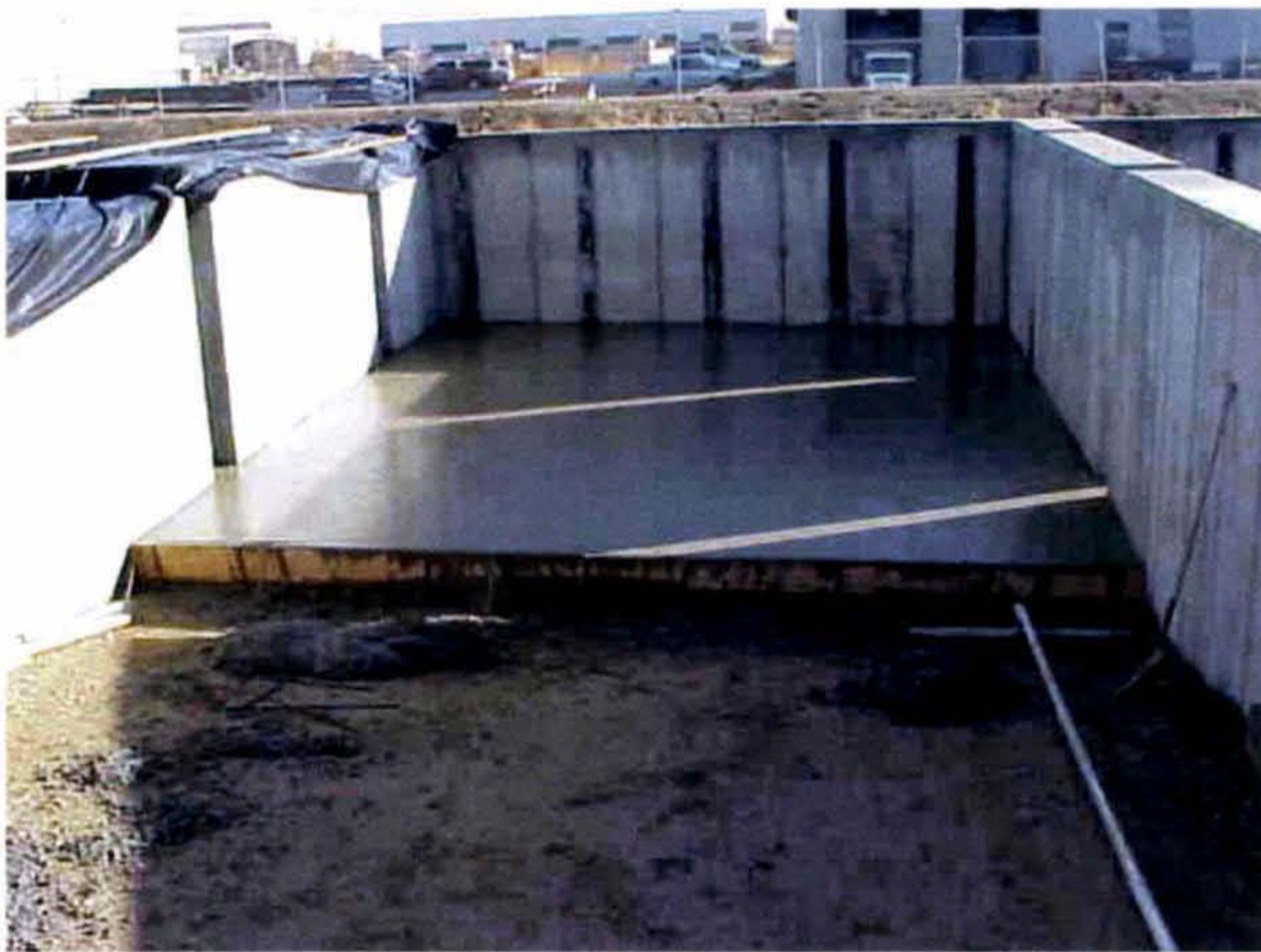
Sediment basin construction
