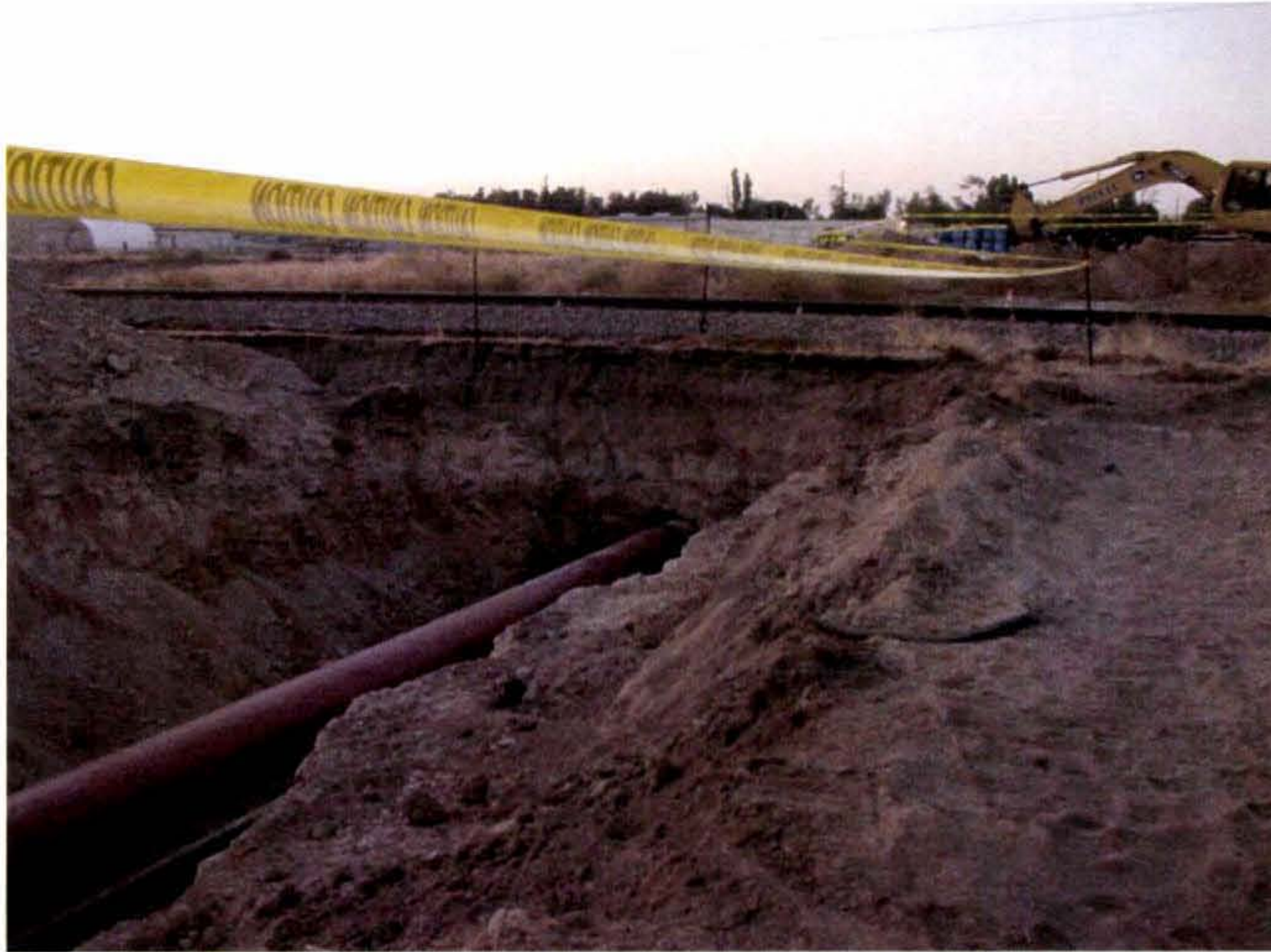
Outfall construction under Union Pacific Railroad tracks
