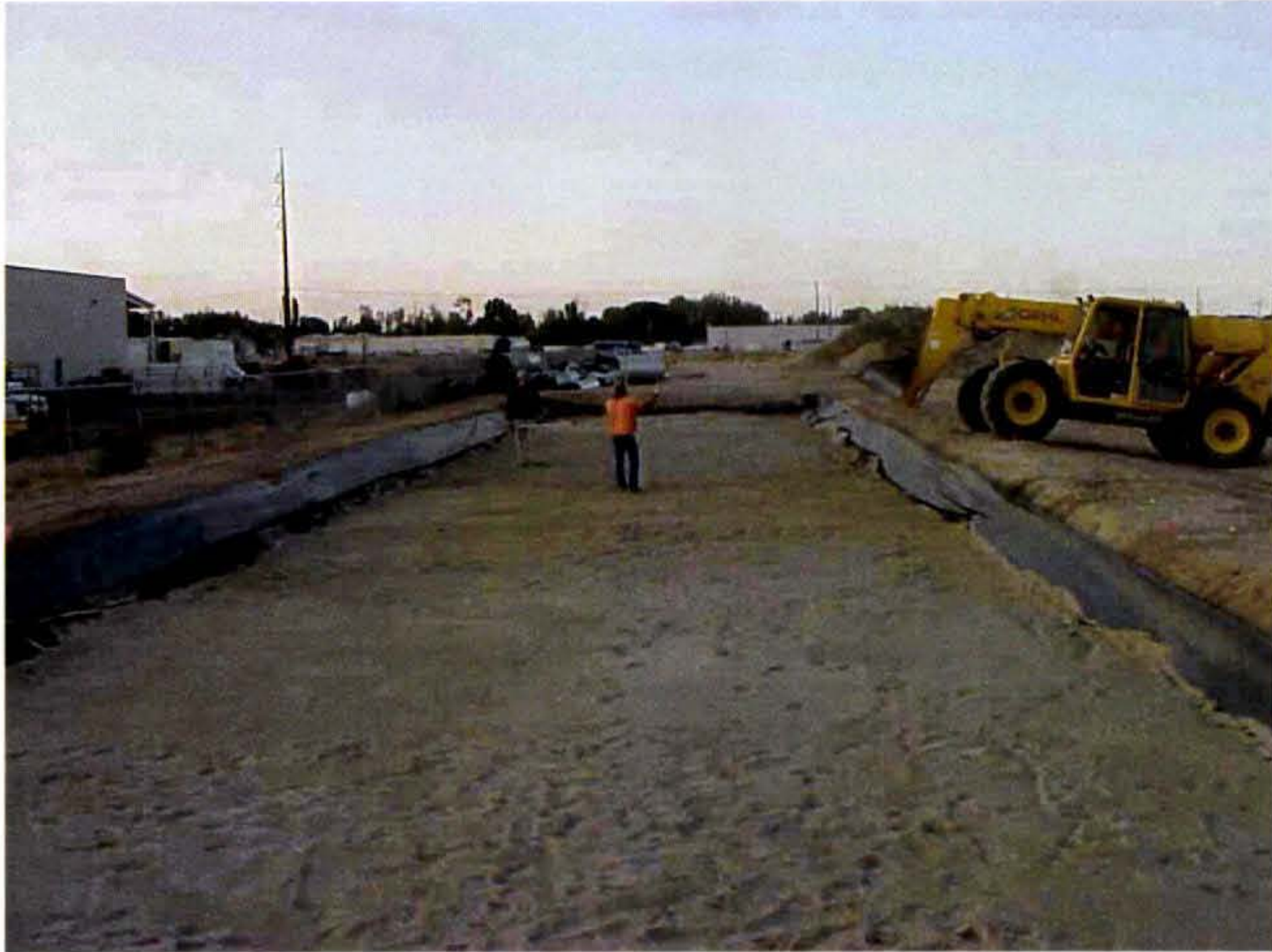
Sand filter construction
