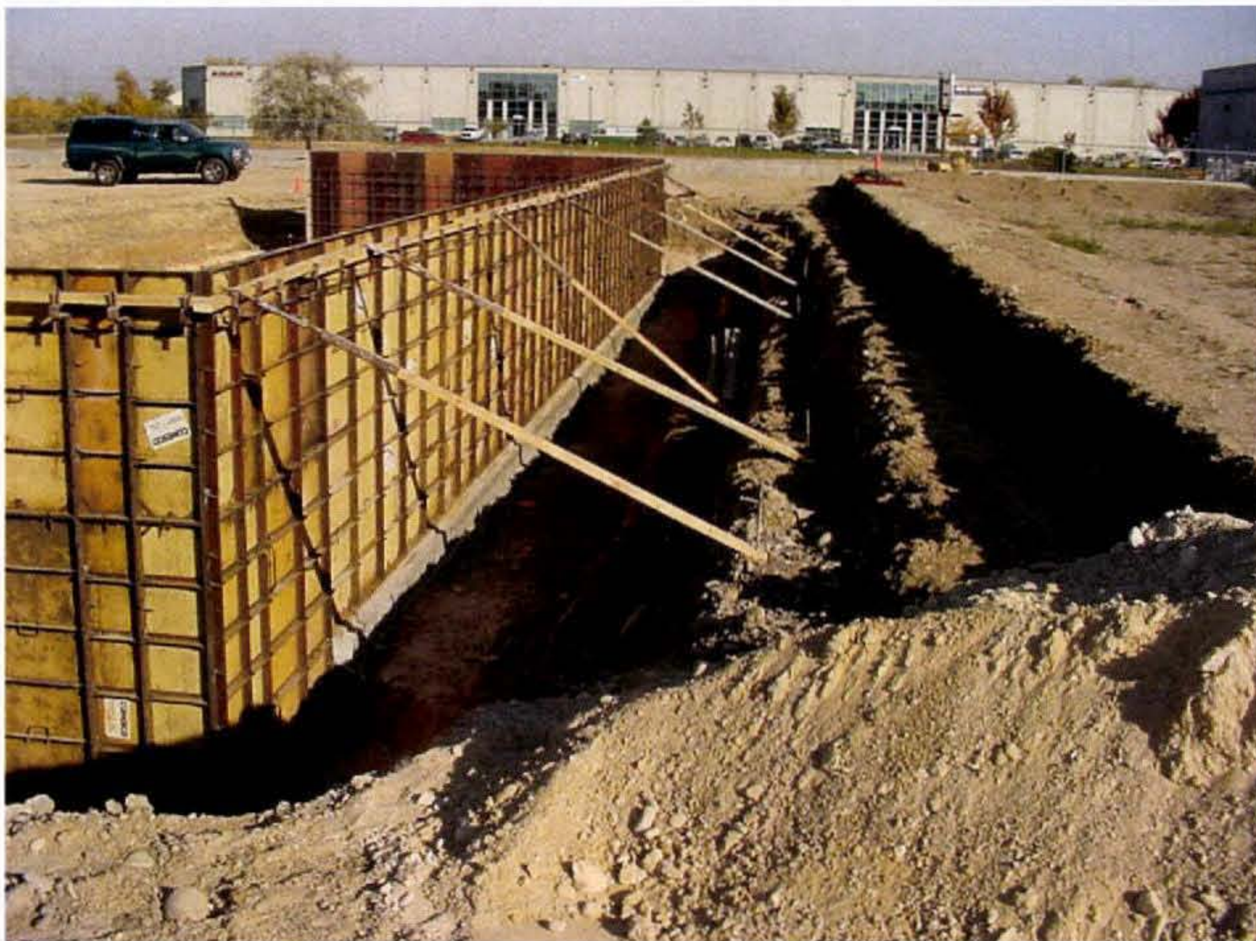
Sediment basin construction
