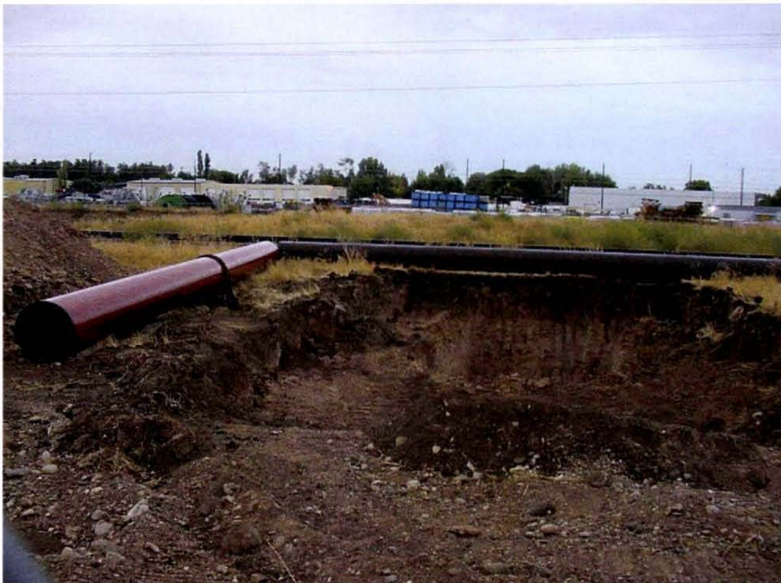
Outfall construction under Union Pacific Railroad tracks
