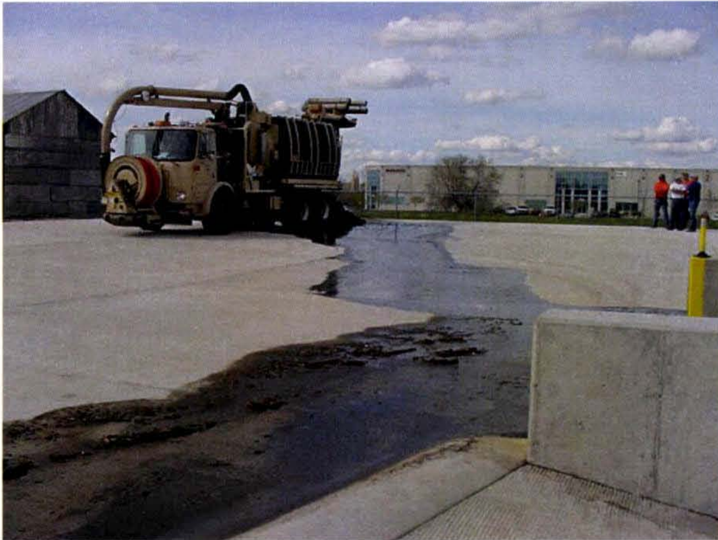
Sediment basin and concrete pad in operation
