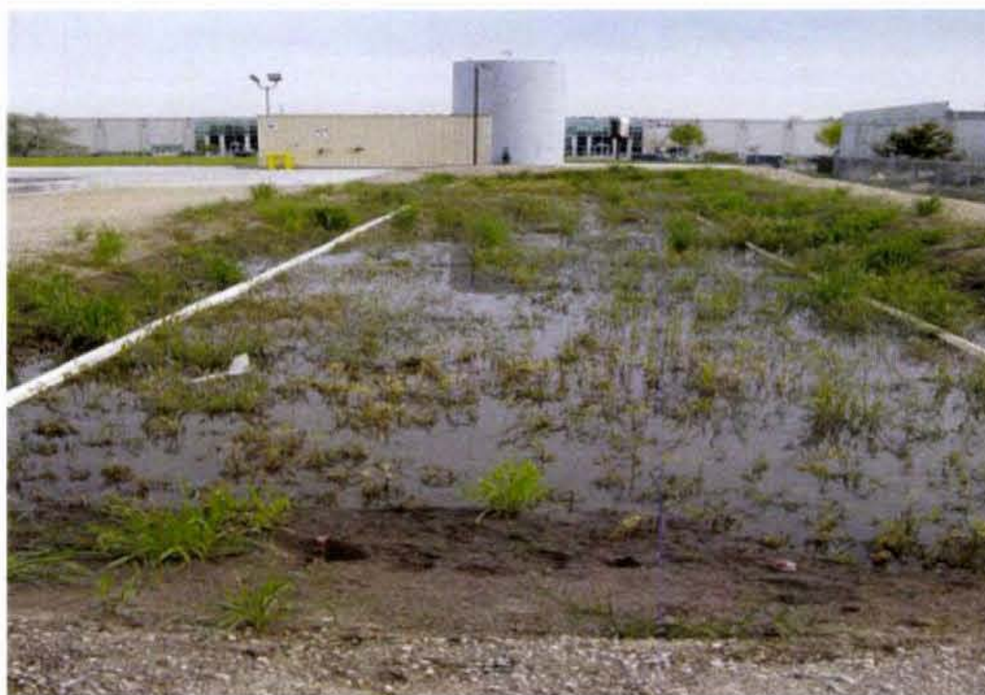
Figure 5.2: Sand filter with storage tank in background, photo taken facing North (photo by Monica Lowe/ACHD 2003)
