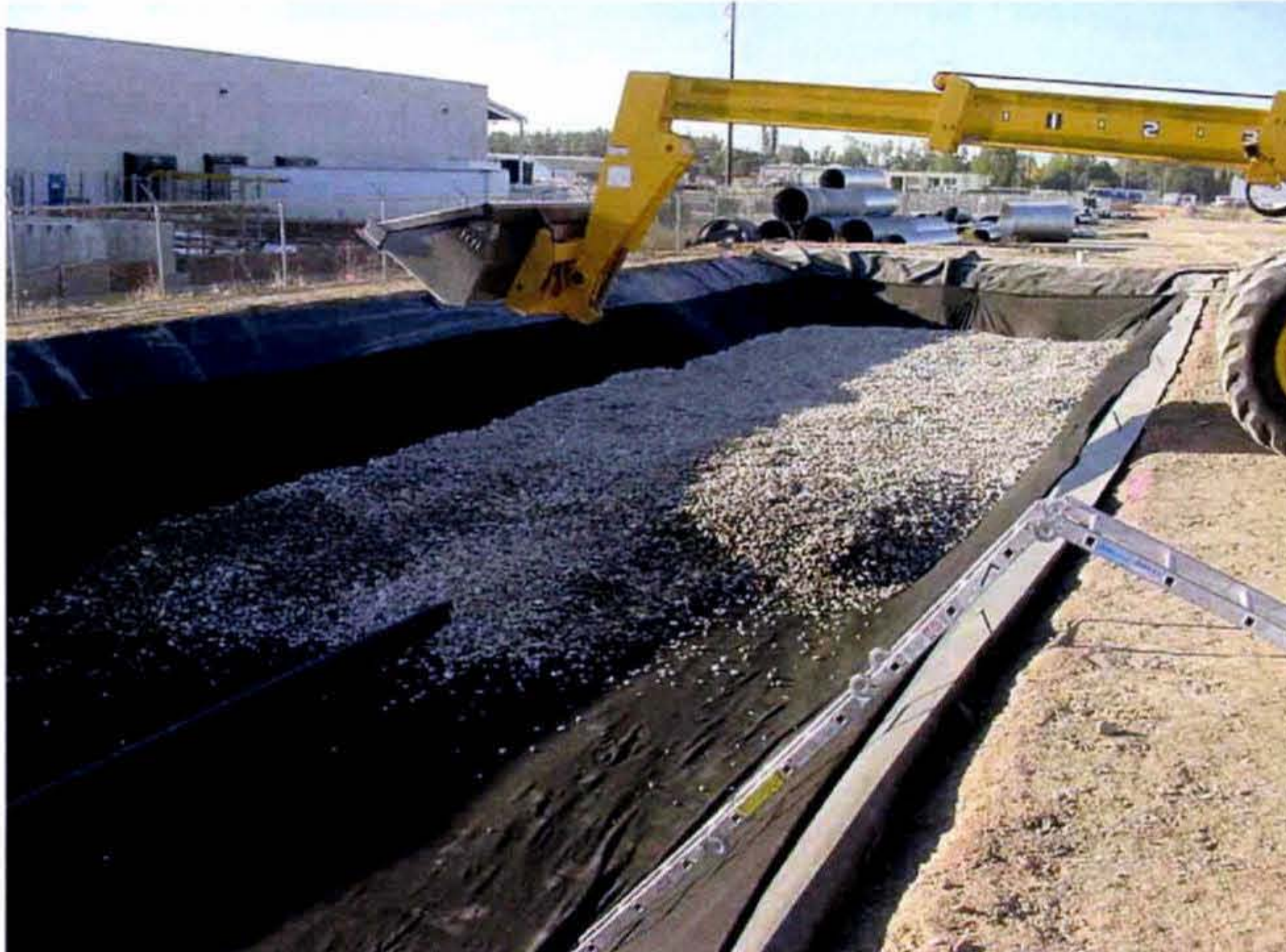
Sand filter construction
