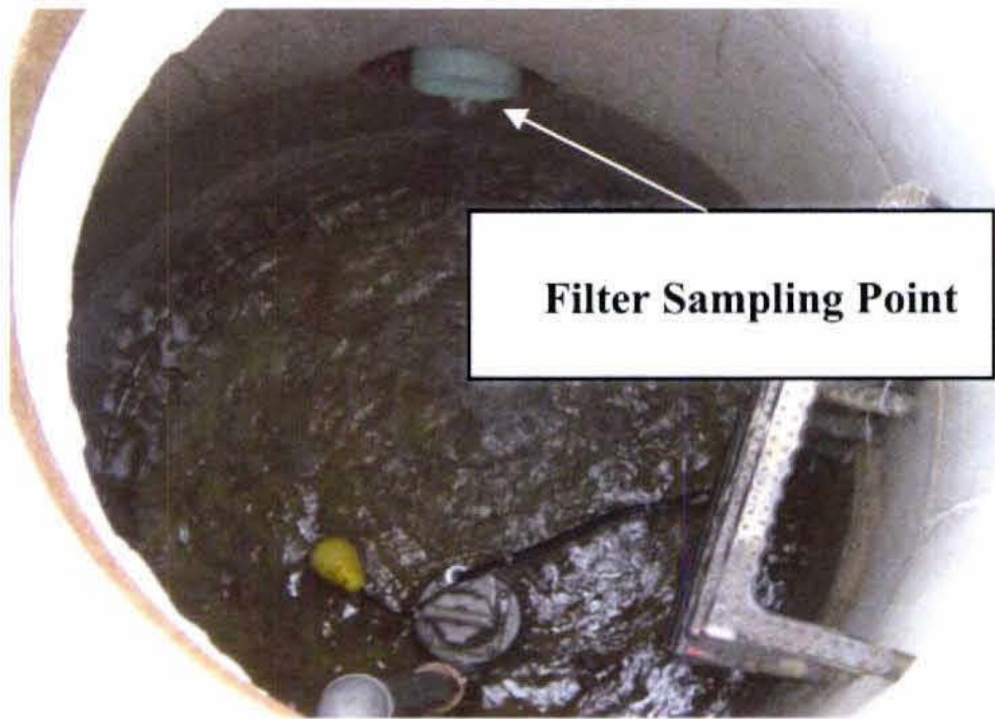
Figure 5.3: Filter sampling point, photo taken looking down with cover removed (photo by Monica Lowe/ACHD 2003)
