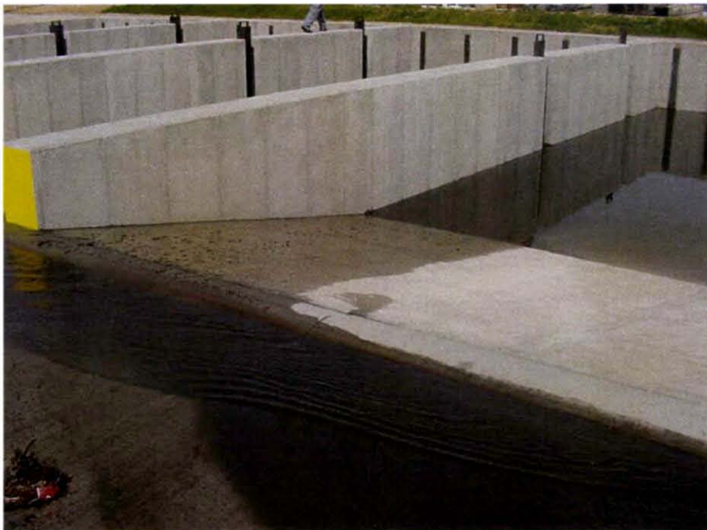
Sediment basin in operation
