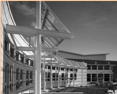
Figure 4.1 Fossil Ridge High School, exterior photo of photovoltaic shade devices. Photo credit: Architectural Record
