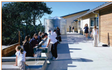
Figure 5.3 Image of the water catchment system and the sluice. Source: EHDD Architecture
