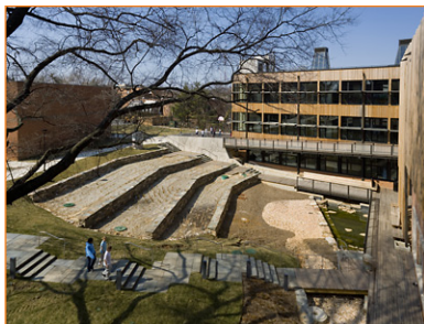
Figure 5.9 View of the Wetland Courtyard. Source: Kieran Timberlake Associates, LLP
