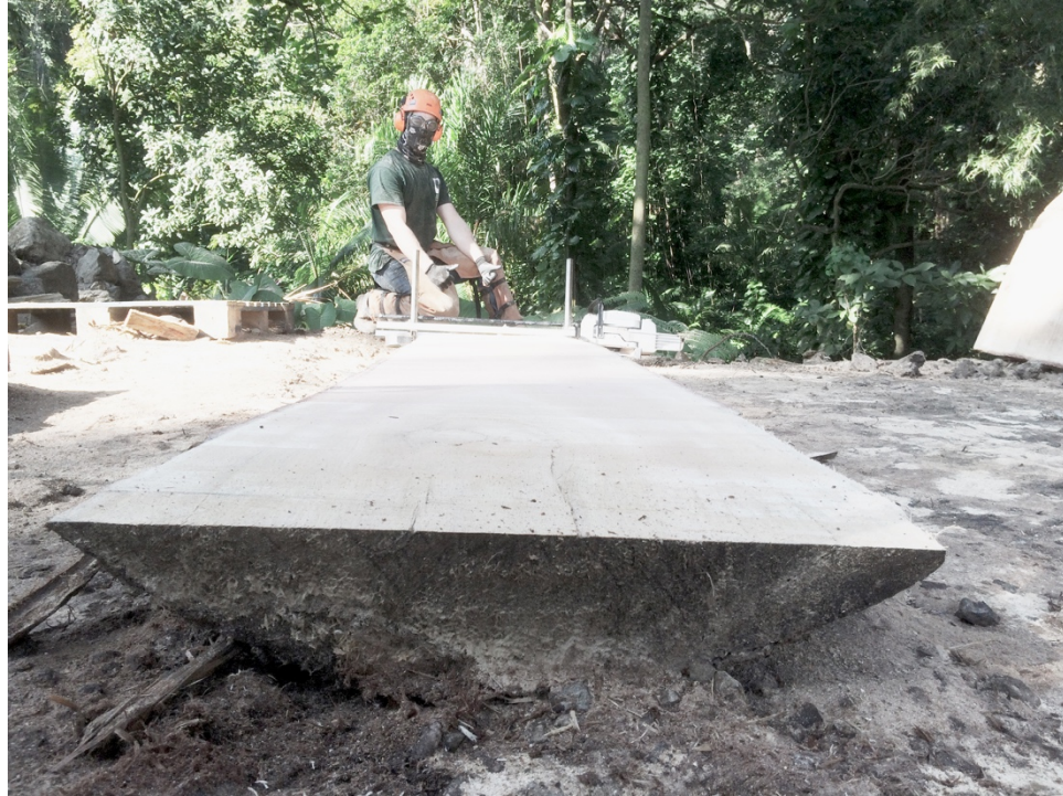
Figure 6.16 Day 5 [January 14, 2016] – Last 1.5” slabs
