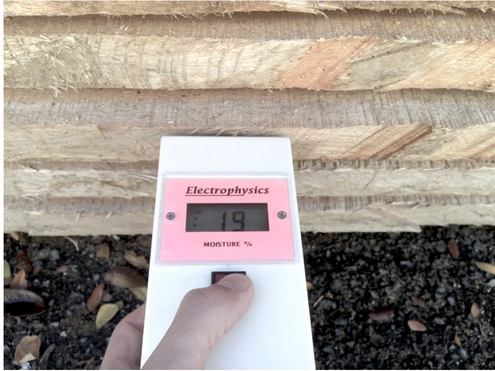
Figure 6.20 Moisture Check #2 [February 3, 2016] @ 19 + 2 = 21%
