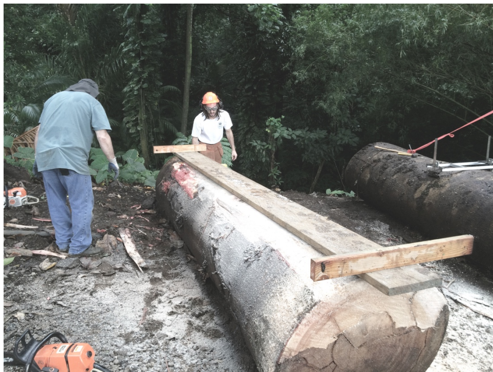
Figure 6.9 Day 1 [December 18, 2015] – Leveling first board
