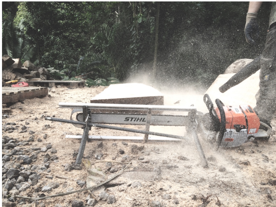
Figure 6.13 Day 3 [January 6, 2016] – Two 1.5” slabs milled
