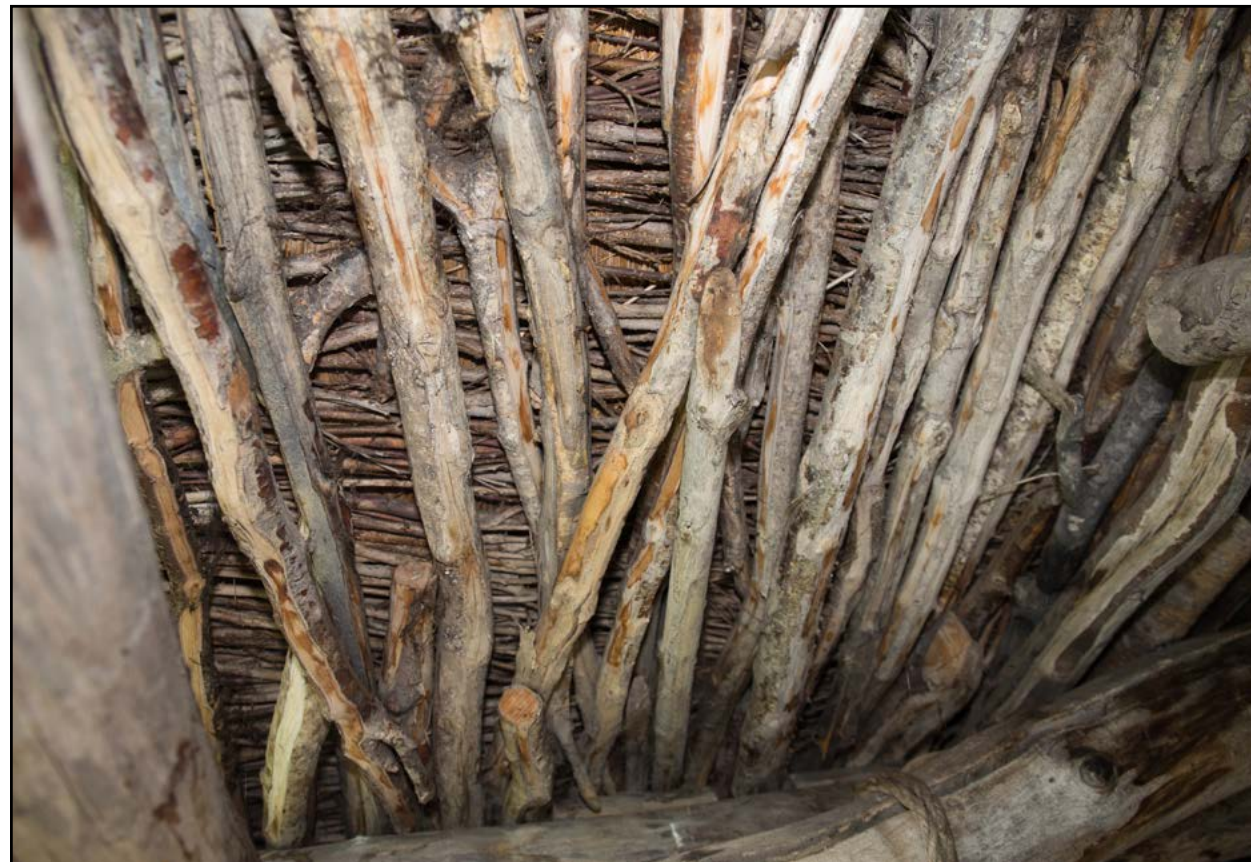
Figure 53. Interior of Gaga Arabuli's home, Barisako, Khevsureti. Roof detail with Rhododendron luteum Sweet webbing above oak and poplar frame.
