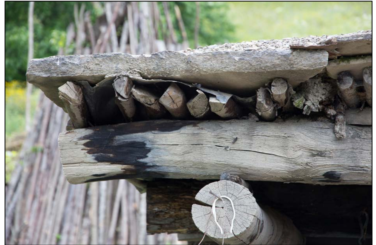
Figure 51. Traditional Khevsureti home of Gaga Arabuli, Barisako village, Khevsureti, Georgia. Roof detail of oak-poplar frame with schist tiles.
