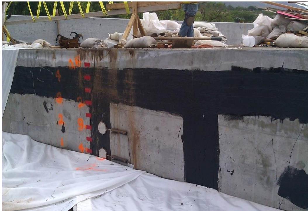
Figure 55 Fatback Cells Fastened to End Wall
