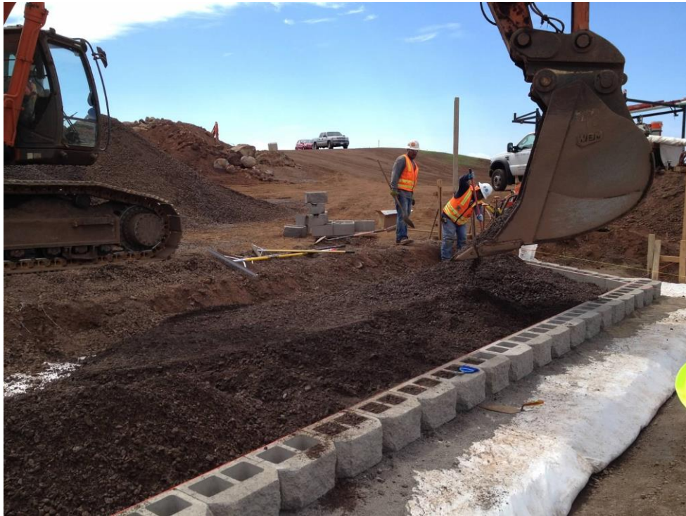
Figure 27 Backfill Placement on Abutment 2
