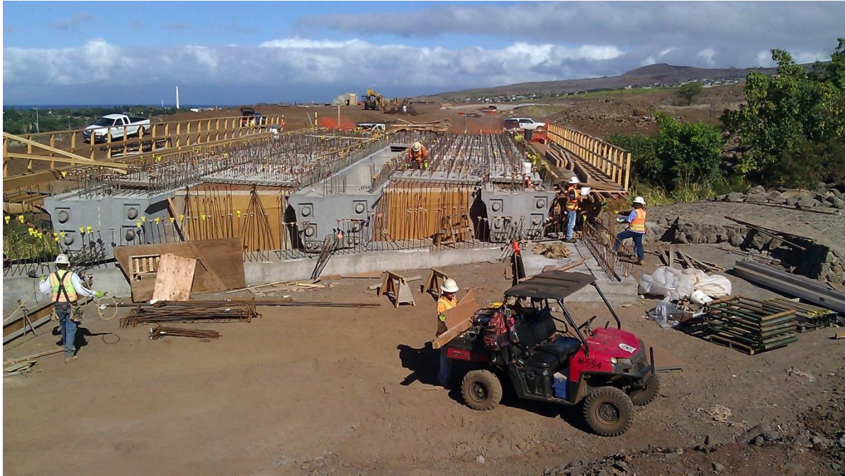
Figure 38 Placement of Precast Concrete Planks on Tub Girders
