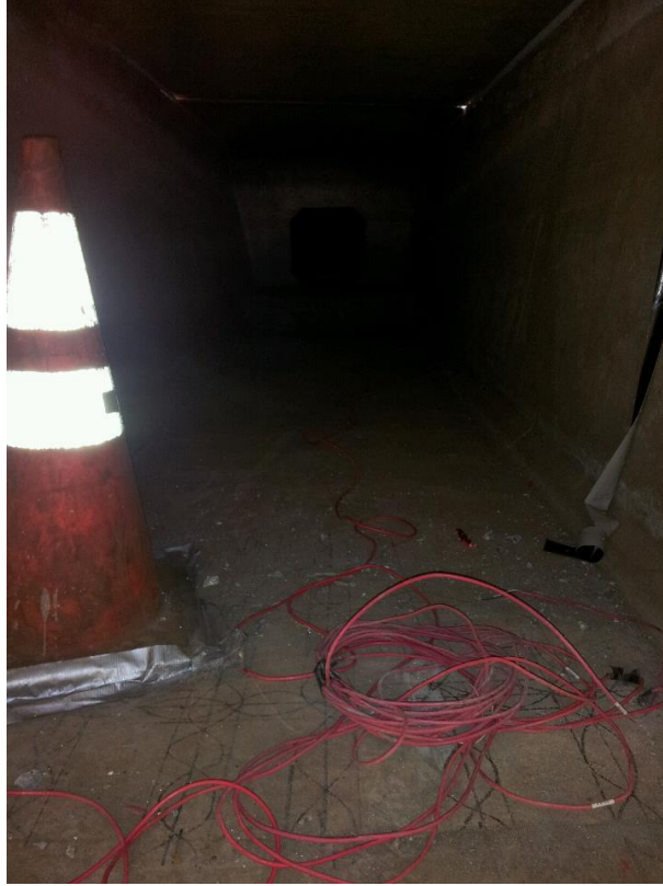
Figure 67 Strain Gage Cables Daylighting from the Floor of the Tub Girder
