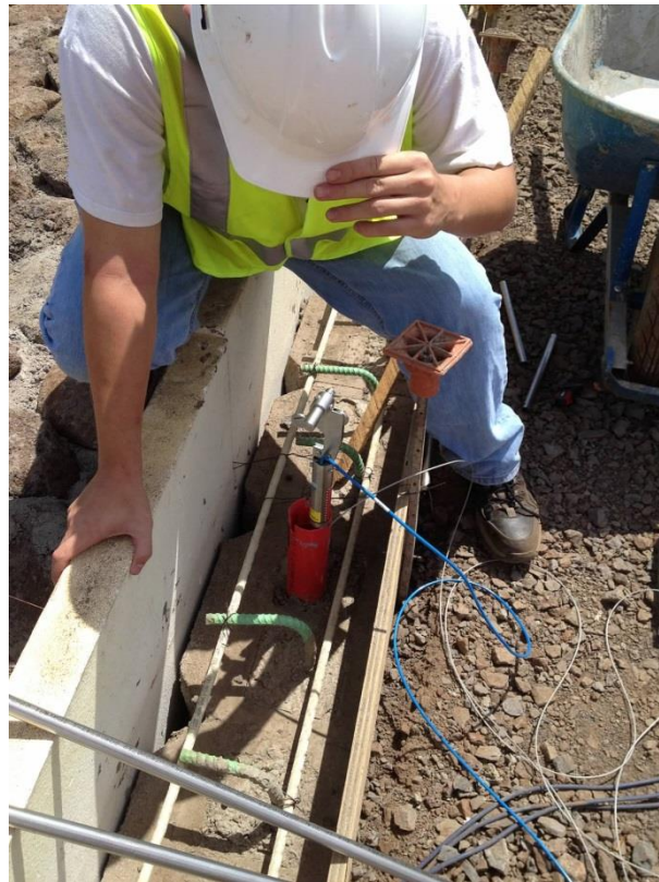
Figure 61 Inclinometers Installed into Glue-Snap Casing
