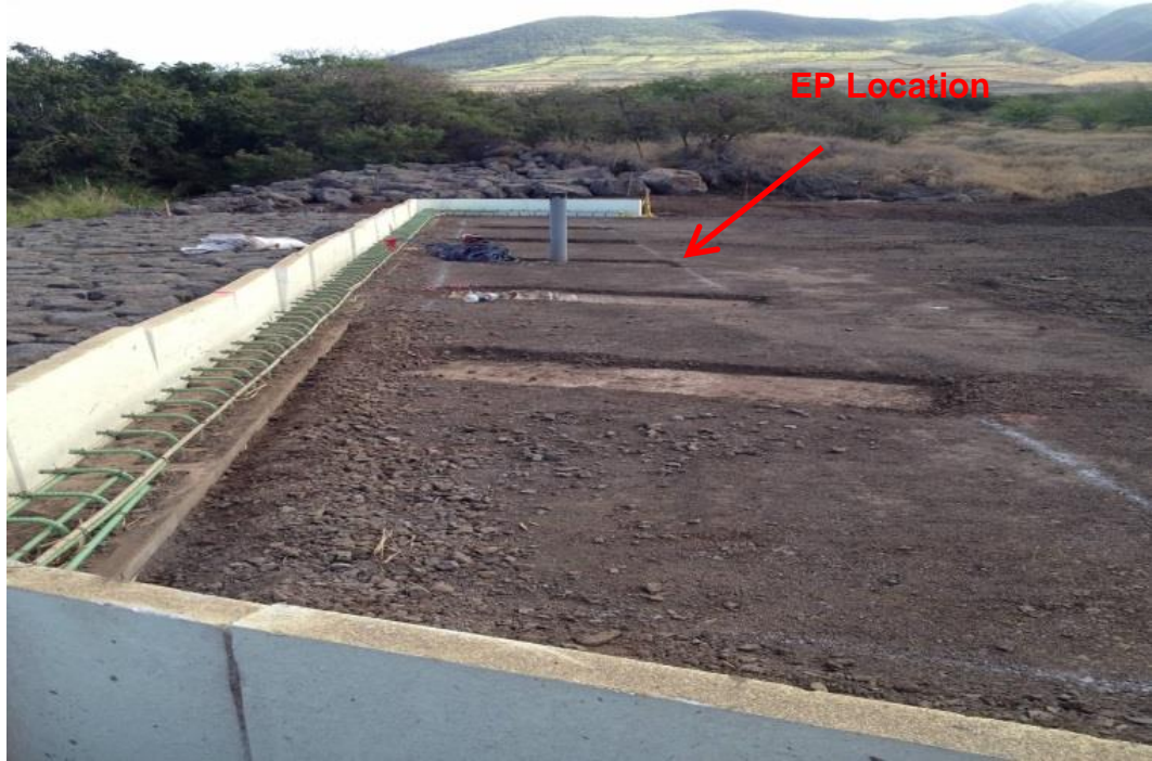
Figure 46 Shallow Hole for Earth Pressure Cells
