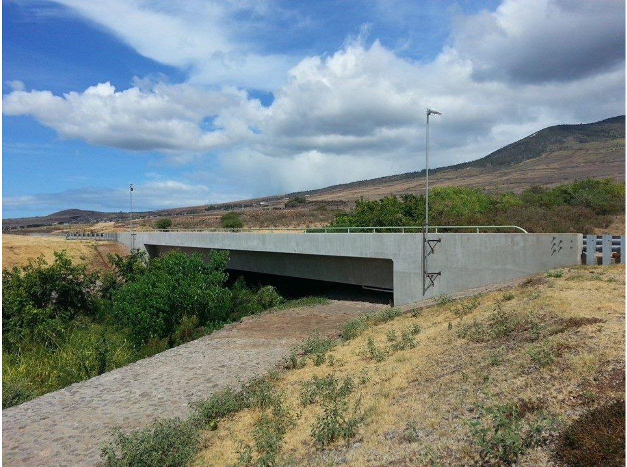
Figure 41 Completed GRS-IBS at Kauaula Stream
