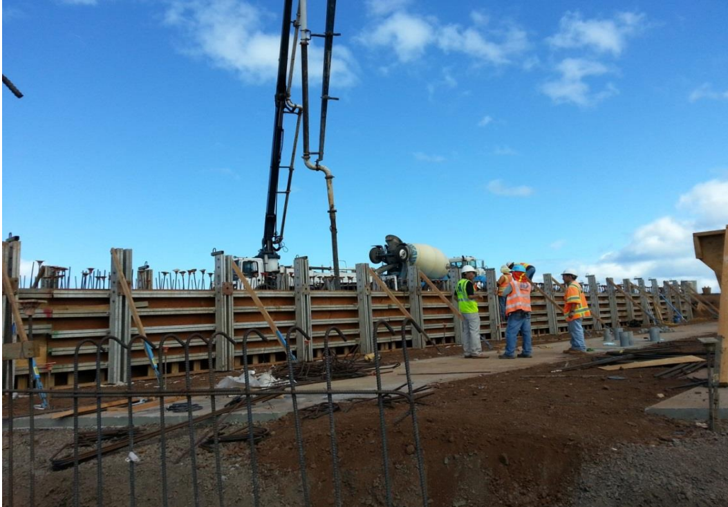
Figure 34 Concrete Floor Pour for Tub Girder
