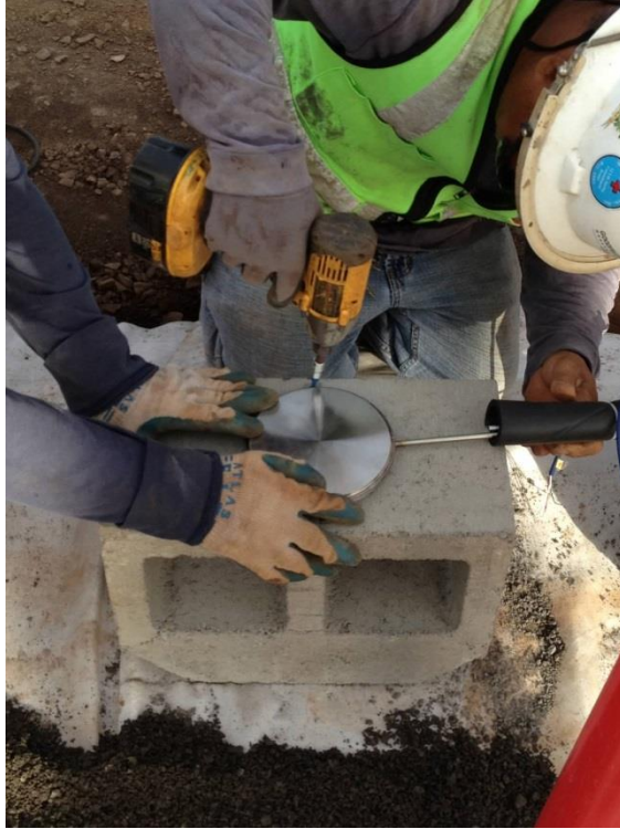
Figure 53 Fatback Cell Fastened to CMU Block
