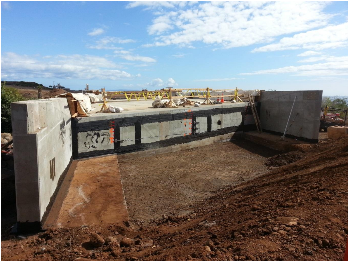
Figure 39 End Walls and Wing Walls Completed
