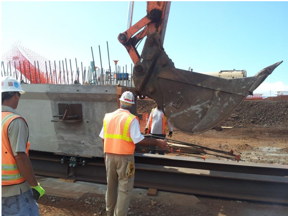
Figure 37 Large Backhoe Pushing Tub Girder
