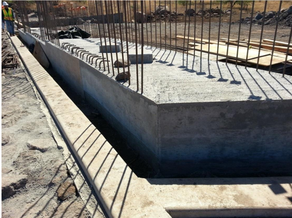
Figure 33 Completed Abutment 2 with Concrete Footing
