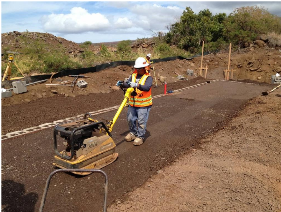
Figure 28 Compaction of Backfill Using a Hand Tamper
