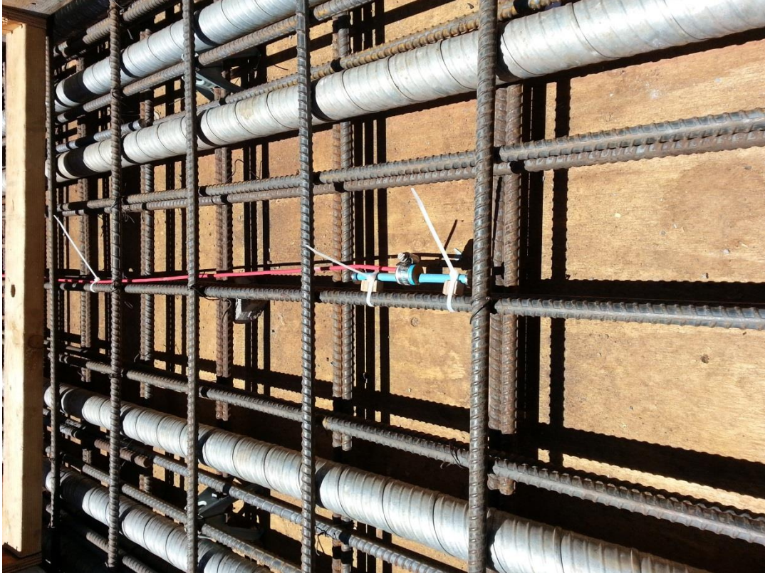
Figure 66 Strain Gage Fastened to Rebar Using Plastic Straps
