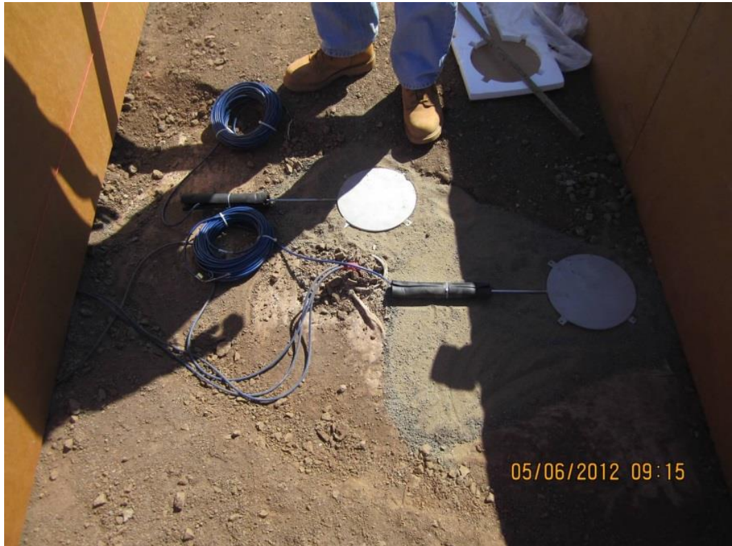
Figure 47 Earth Pressure Cells Placed on a Flat Layer of Sand
