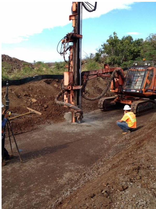
Figure 26 Drilling Hole for Inclinometer Casing
