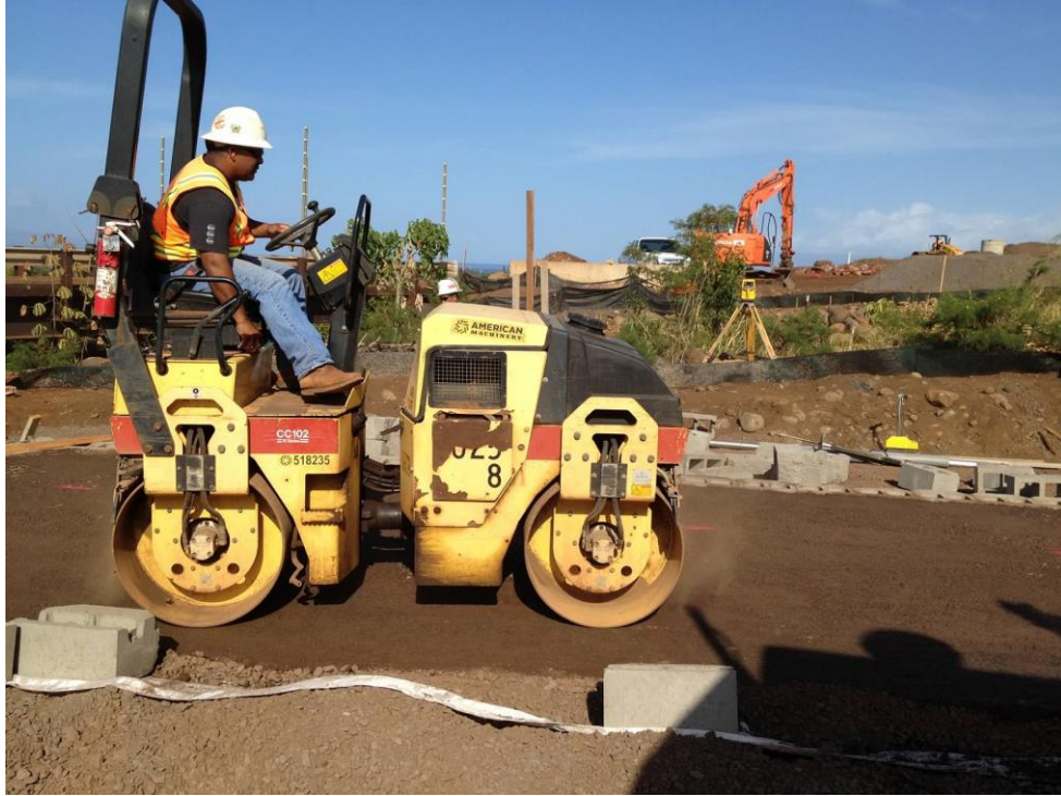
Figure 29 Compaction of Backfill by Vibratory Roller
