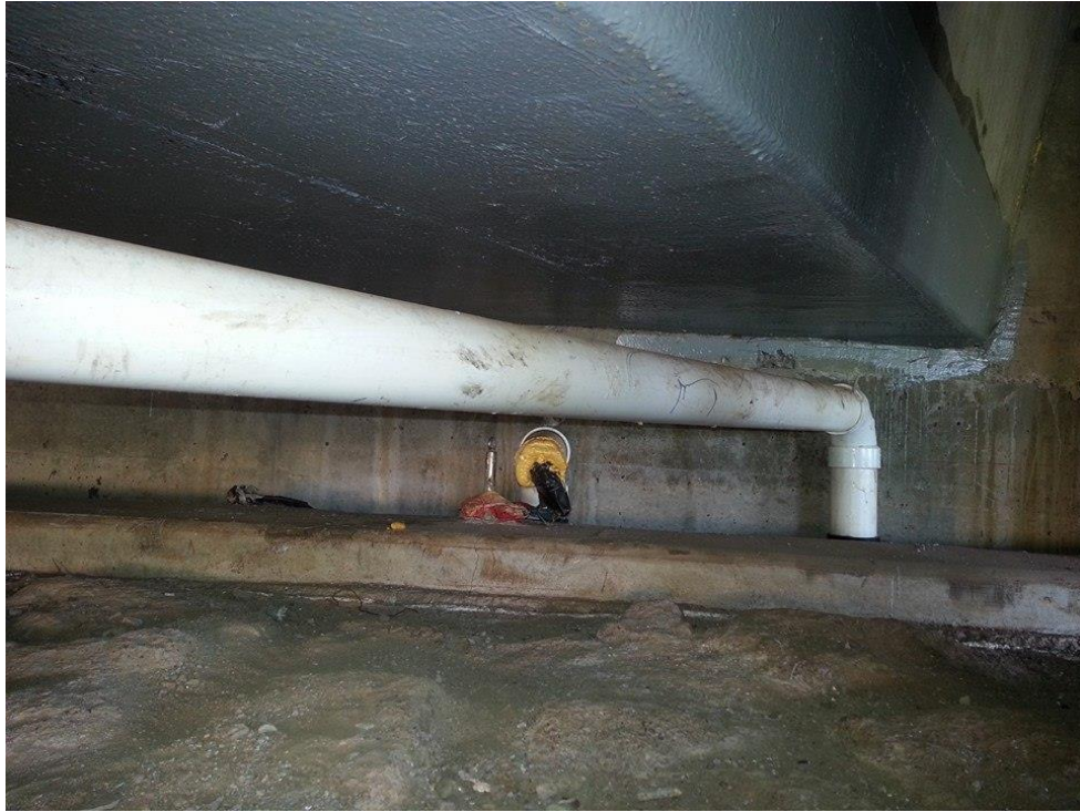
Figure 72 PVC Pipe System Under the Middle Tub Girder
