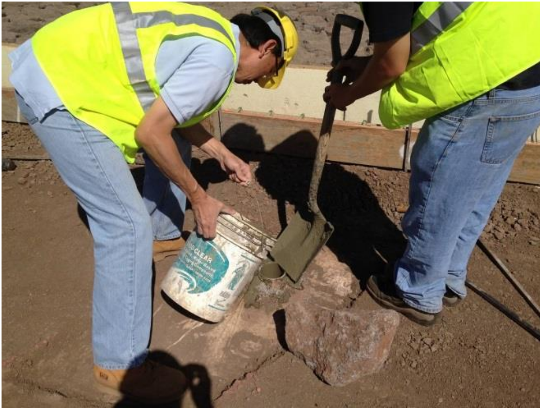
Figure 71 Grout Mixture Poured into PVC Pipe Housing Deformation Meter
